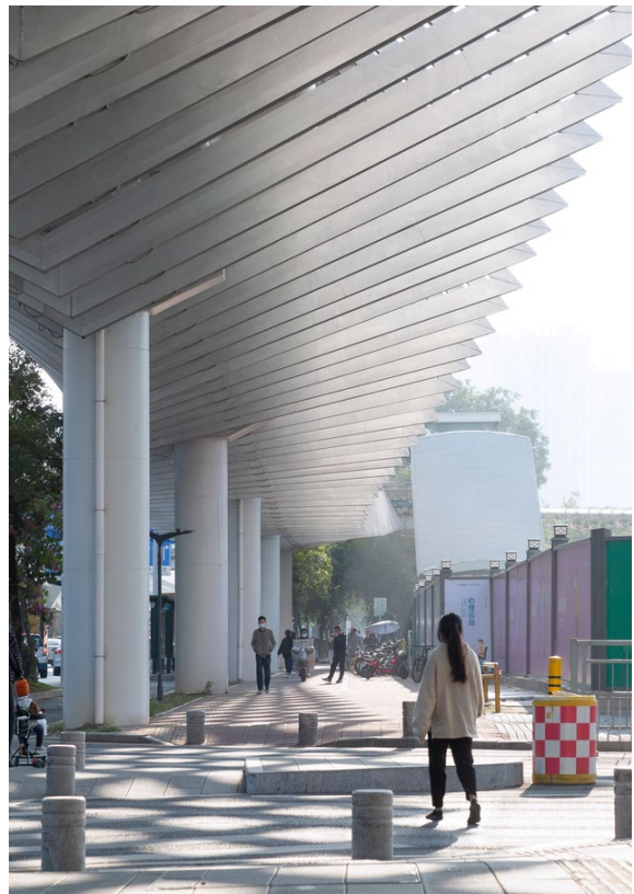
Creative design solution for the underbelly of the overpass gives a place a special feeling.
