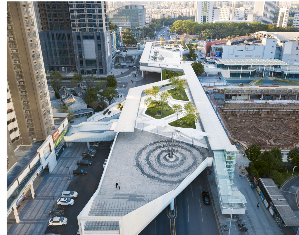
Opportunity to integrate elevated plazas, and green roofs as part of raised platforms, contributing to a sense of place and ownership for the community.
