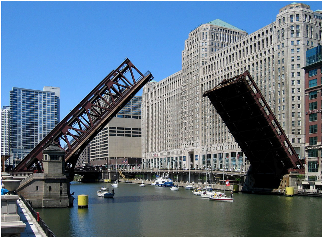
Figure 14. Double-deck Double-leaf Bascule Bridge Example – Wells Street Bridge, Chicago, IL
