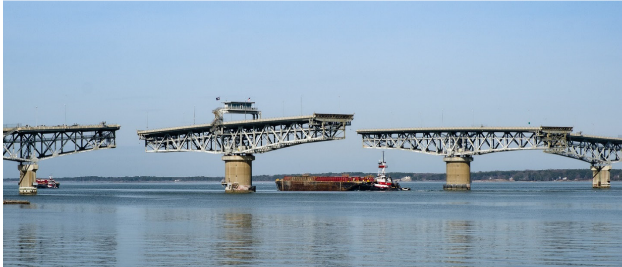
Figure 15. Single-deck Double-swing Bridge Example – Coleman Bridge, York County, VA
