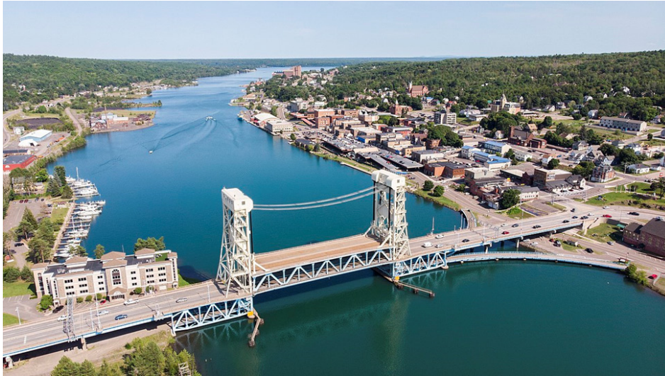
Figure 13. Double-deck Vertical Lift Bridge Example – Portage Lake Bridge, Houghton, MI
