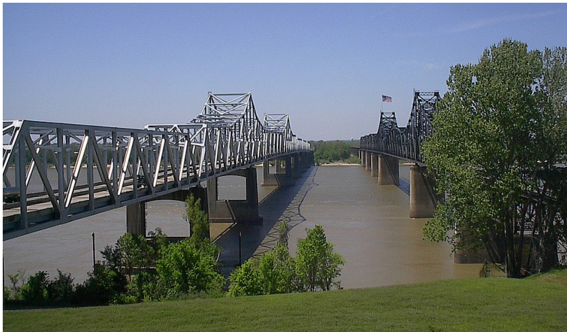
Figure 17. Mid-level Fixed Bridge Example – Vicksburg Bridge, Delta, LA and Vicksburg, MS
