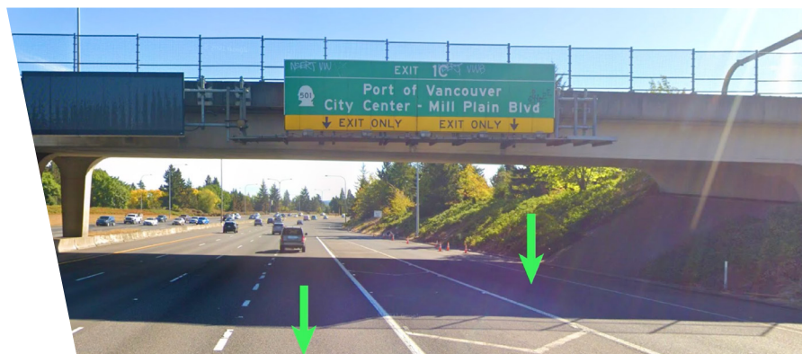
This is a photo of an auxiliary lane currently in place to connect the Fourth Plain on-ramp to the Mill Plain off-ramp to reduce merging and weaving.
