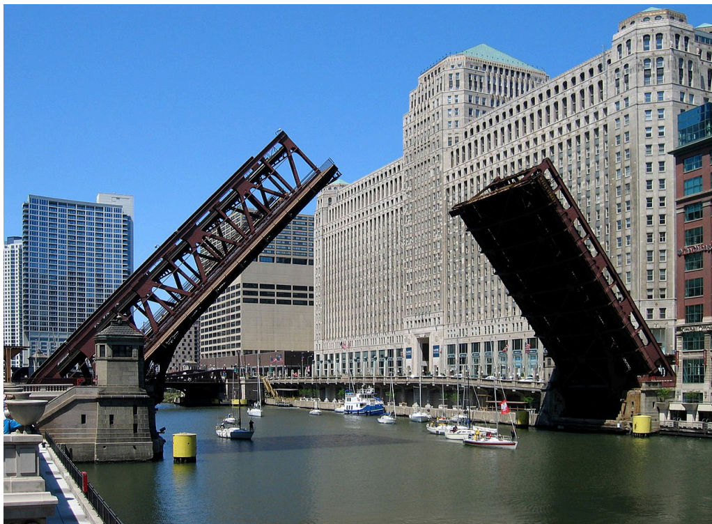
Figure 3. Double-deck Double-leaf Bascule Bridge Example – Wells Street Bridge, Chicago, IL
