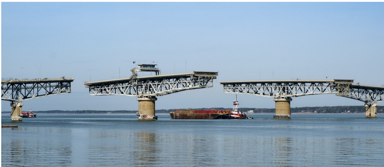
Figure 4. Single-deck Double-swing Bridge Example – Coleman Bridge, York County, VA
