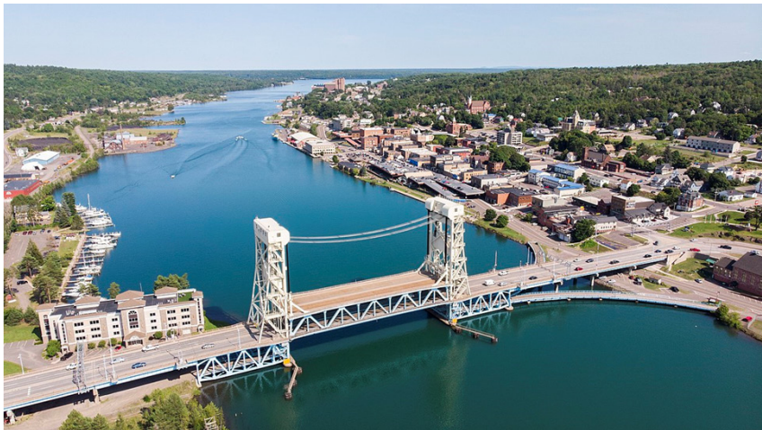
Figure 2. Double-deck Vertical Lift Bridge Example – Portage Lake Bridge, Houghton, MI
