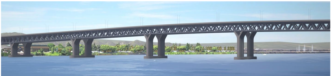
Figure 1-15. Conceptual Drawing of a Double-Deck Fixed-Span Configuration
