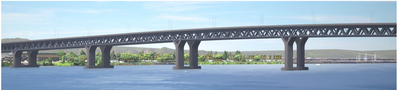
Figure 1-15. Conceptual Drawing of a Double-Deck Fixed-Span Configuration
