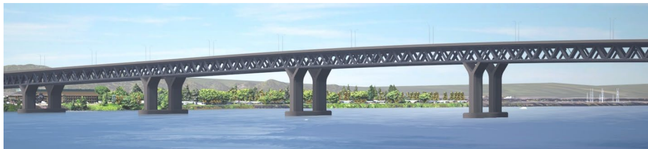
Figure 1-15. Conceptual Drawing of a Double-Deck Fixed-Span Configuration
