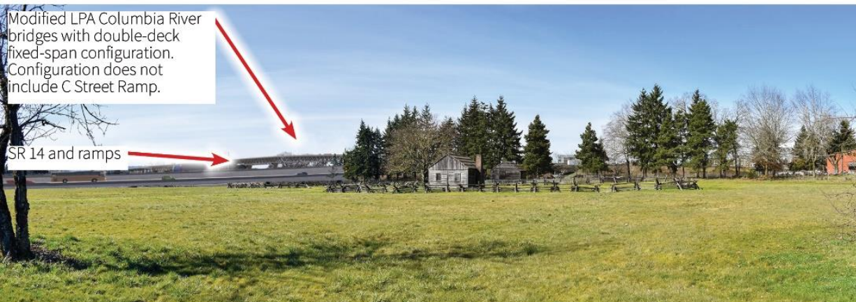
Photographic simulation of Modified LPA with double-deck fixed-span configuration without C Street Ramp
