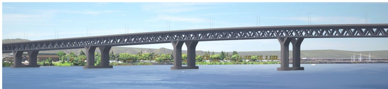
Figure 1-15. Conceptual Drawing of a Double-Deck Fixed-Span Configuration
