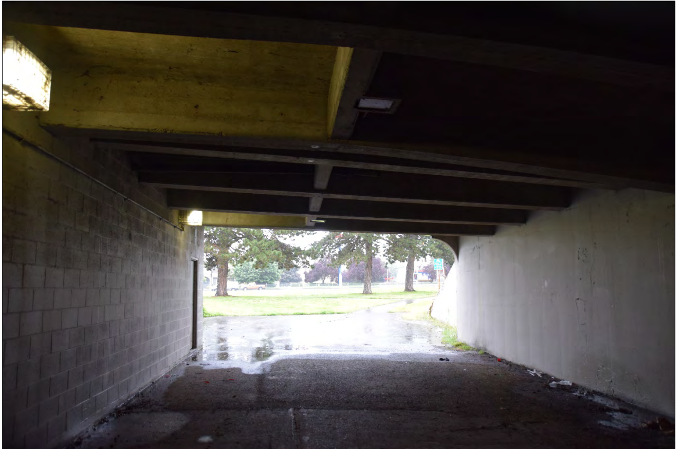
Figure 6. Jantzen Beach Pedestrian Tunnel, interior, view looking east (WillametteCRA June 10, 2022).
