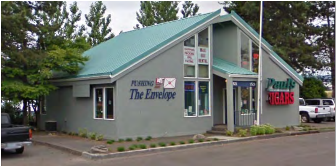
Figure 9. 2009 photograph of the building, view facing southeast. Note the since removed windows on the east (side) elevation (Google Street View, 2009).
