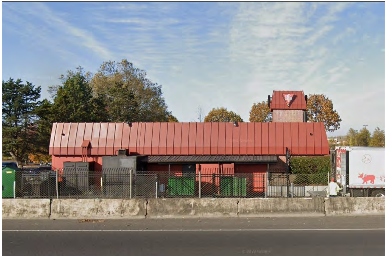
Figure 7. Engine House Pizza Co. #1, east elevation, view facing west. Note that the east side of the building was not accessible to pedestrian survey. The elevations have not been significantly altered since captured by Google (Google Street View November 2022).
