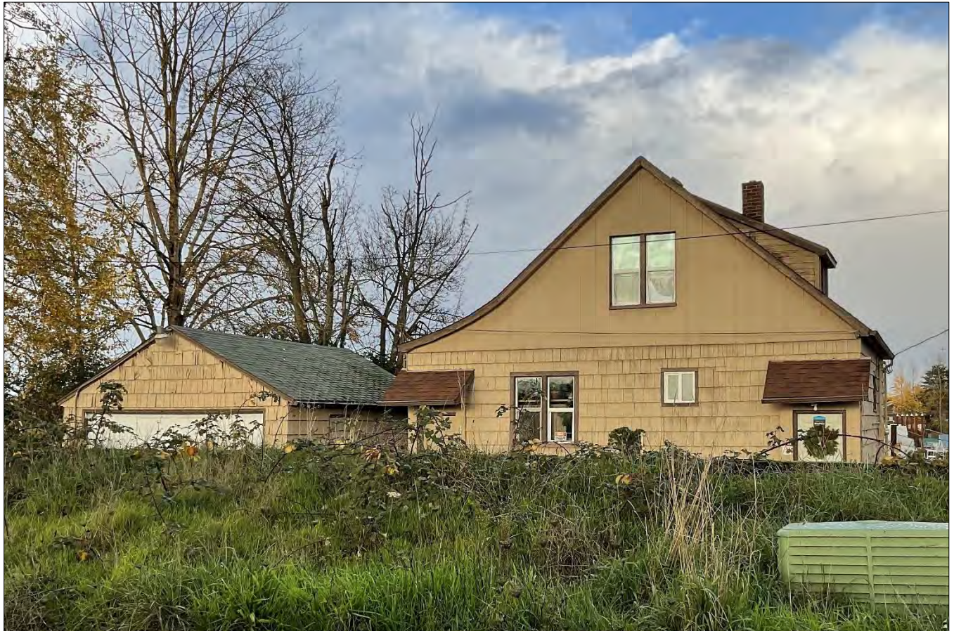
Figure 7. South elevation of the Westerlund Residence, view facing north (WillametteCRA December 2021).
