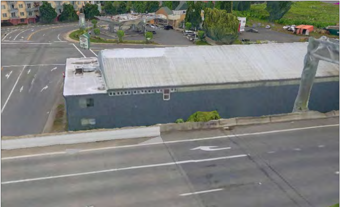
Figure 4. Rudy Yost Equipment, west elevation, view facing northeast showing garage fenestration (IBR/Bentley Systems May 26, 2002).
