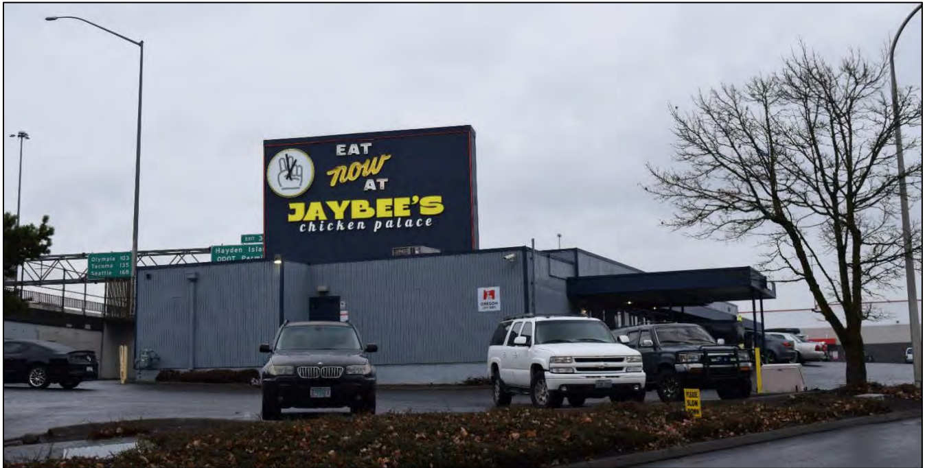
Figure 4. JayBee's Chicken Palace (Waddle's Drive-In Coffee Shop), south and east elevations, view facing northwest (WillametteCRA January 16, 2023).
