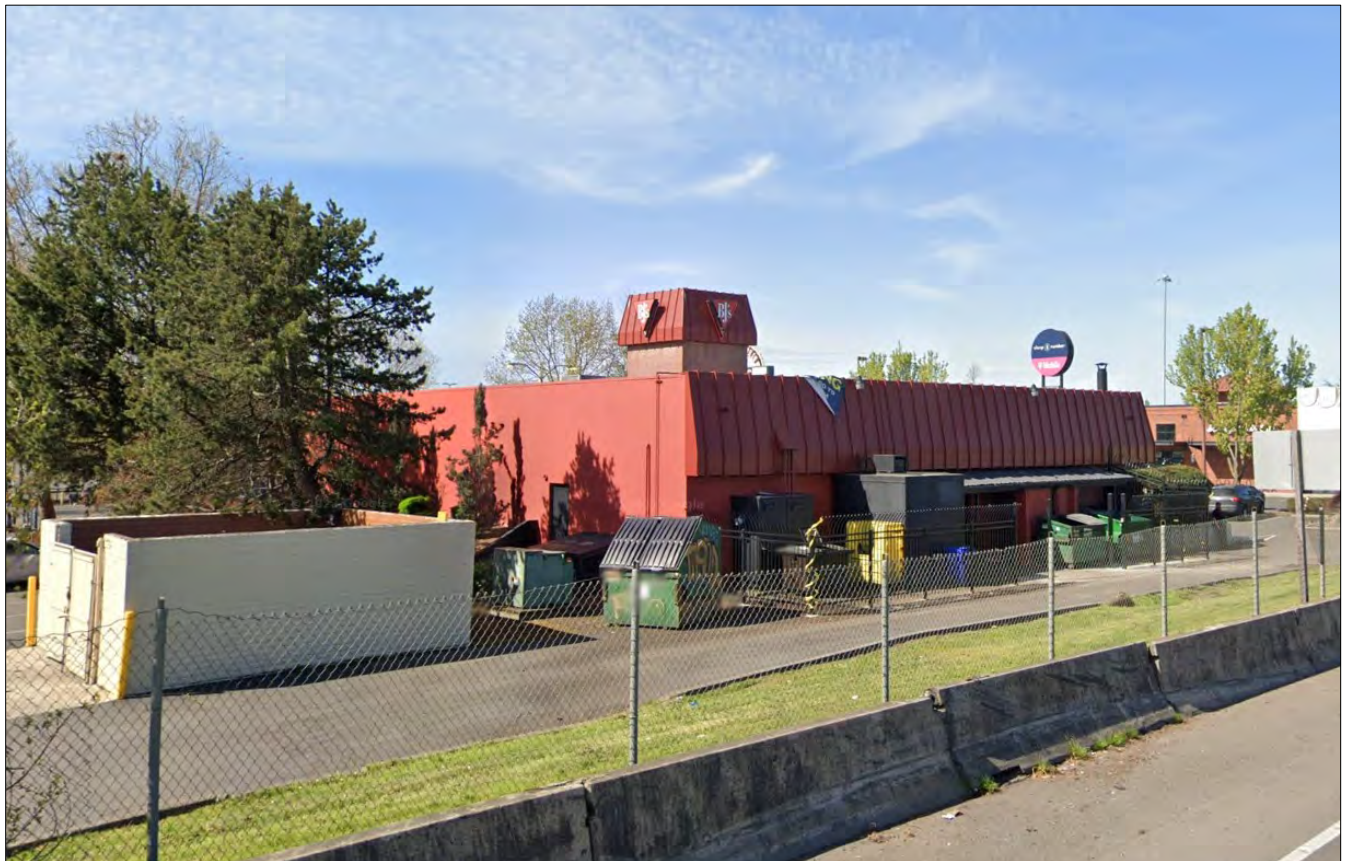
Figure 4. Engine House Pizza Co. #1, south and east elevations, view facing northwest. Note that the east side of the building was not accessible to pedestrian survey. The elevations have significantly altered since captured by Google (Google Street View April 2022).
