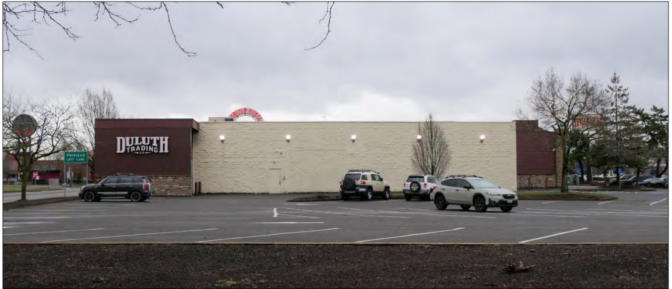
Figure 6. Montgomery Ward Automotive Center Building, north elevation, view facing south (WillametteCRA January 22, 2024).
