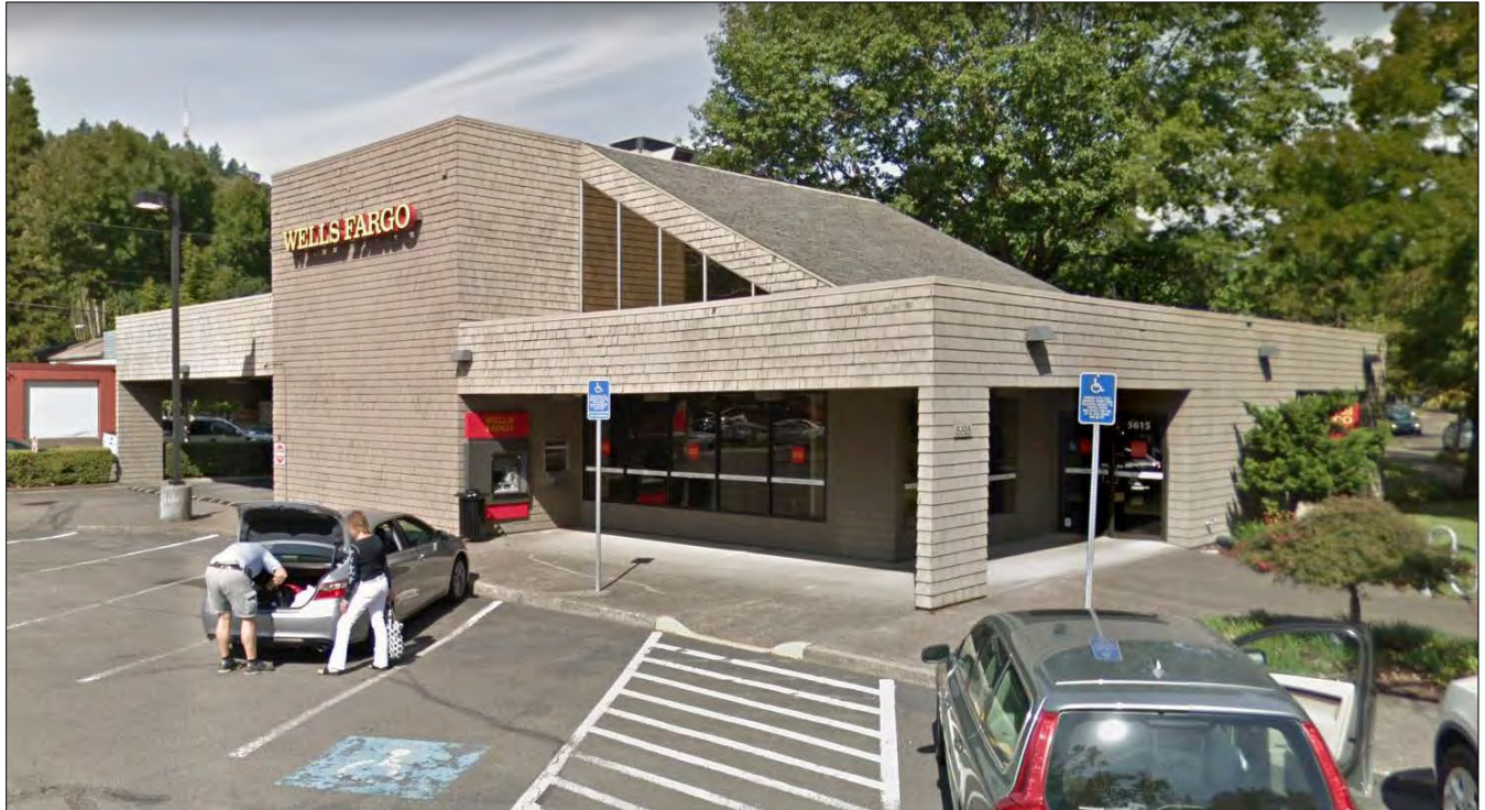
Figure 11. Wells Fargo (Formerly First Interstate Bank) branch office at 5615 Southwest Macadam Avenue, Portland, OR. Constructed by Modern Building Systems in 1972. Addition with shed roof constructed in 1980 (Google Street View, September 2017).
