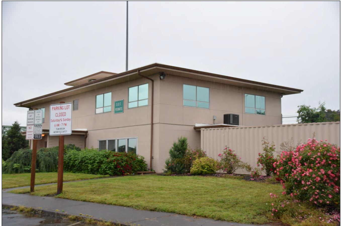
Figure 7. West and south elevations of the Toll Administration Building (ODOT Permit Center). View facing northeast (WillametteCRA June 10, 2022).
