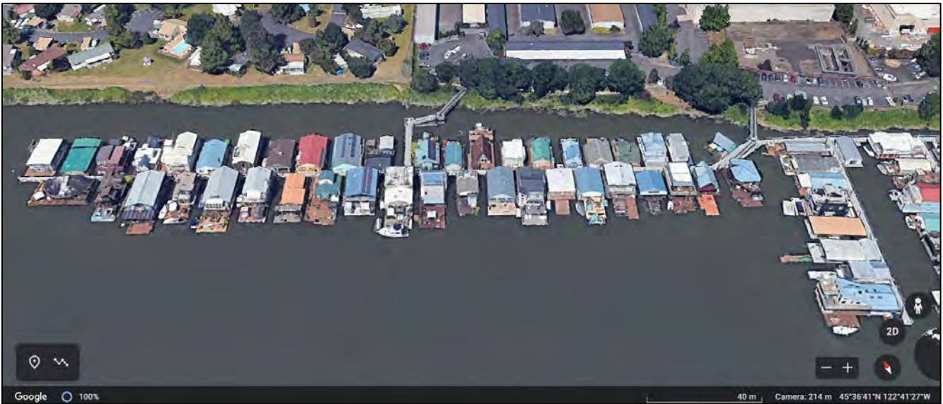
Figure 9. Jantzen Beach Moorage, M walk West and Row Q. View facing north (Google Earth 2023).
