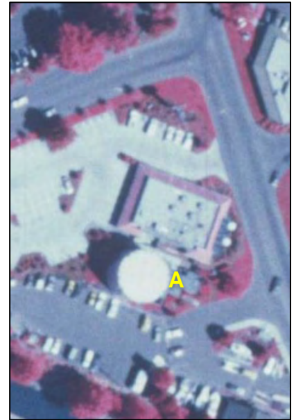
Figure 17. 1986 aerial photograph of Water Tank and Pump House. Building B appears to have been removed while Building A has been expanded (Portland Maps, 1986).
