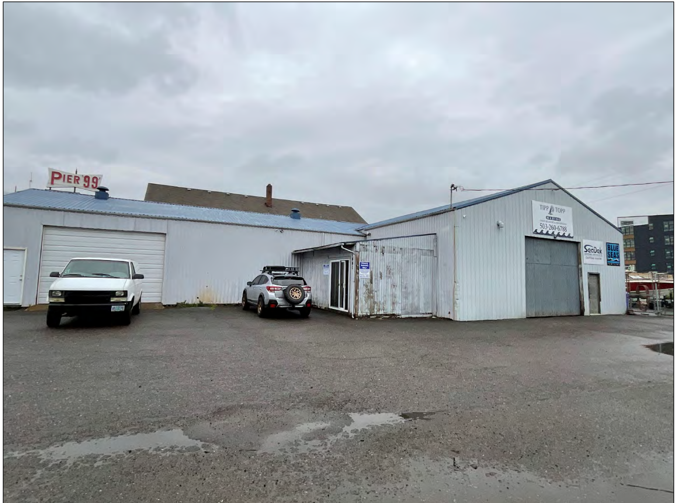
Figure 16. Tipp Topp Marine Building, main entrance. View facing northeast (WillametteCRA May 4, 2023).
