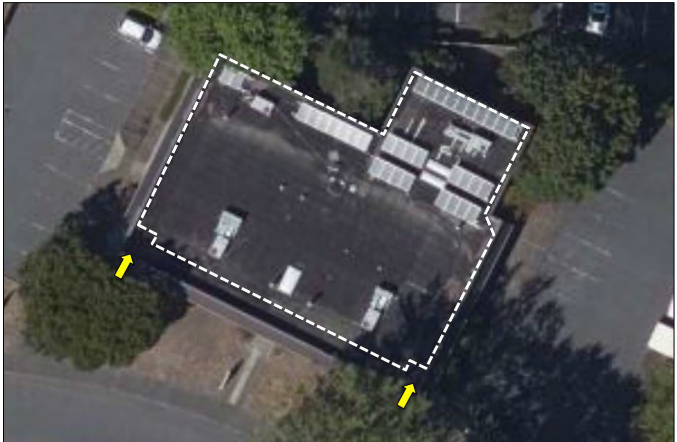
Figure 4. Annotated 2021 Aerial photo of the building shows the approximate outline of the building's outer walls recessed under the overhanging roof. Arrows point to recessed entries on the building's south elevation (Portland Maps).
