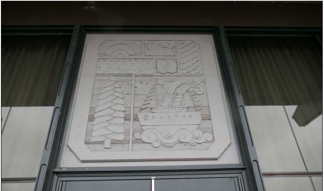
Figure 17. Representative view of carved glulam panels on north elevation of banquet hall (WillametteCRA May 4, 2023).
