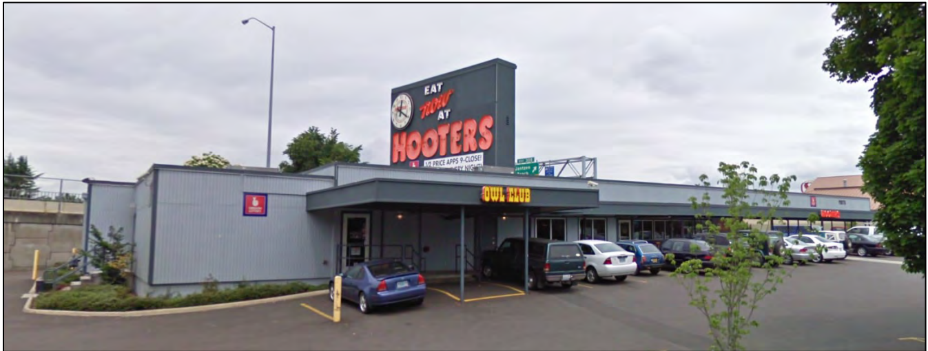
Figure 39. Hooters Restaurant, east elevation, view facing northwest (Google Streetview, June 2009).
