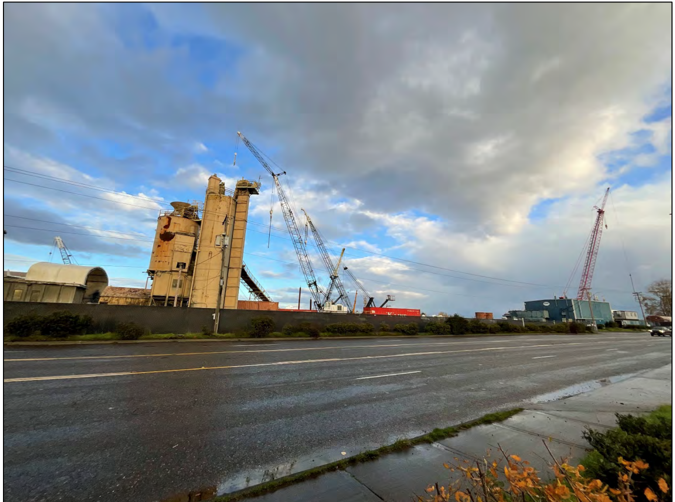
Figure 5. View of Vanport Pier from southwest (WillametteCRA, December 8, 2021).
