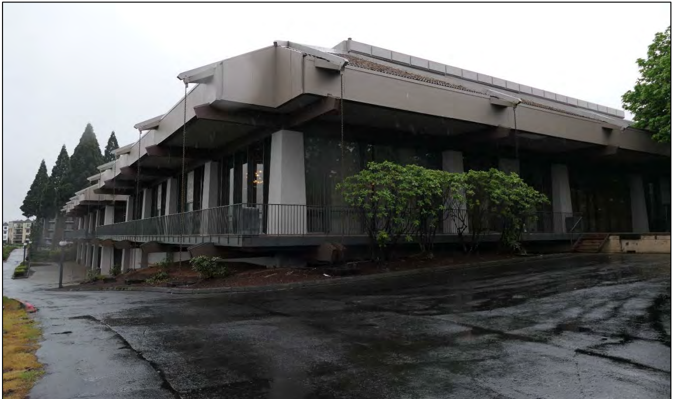
Figure 12. North and east elevations of banquet hall, with balcony and roof details. View facing southwest (WillametteCRA May 4, 2023).
