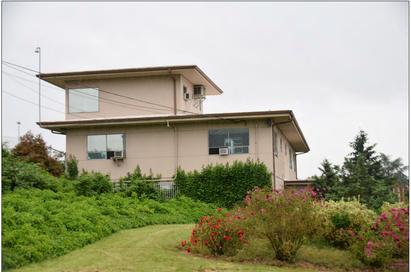
Figure 4. North elevation of the Toll Administration Building (ODOT Permit Center). View facing south (WillametteCRA June 10, 2022).
