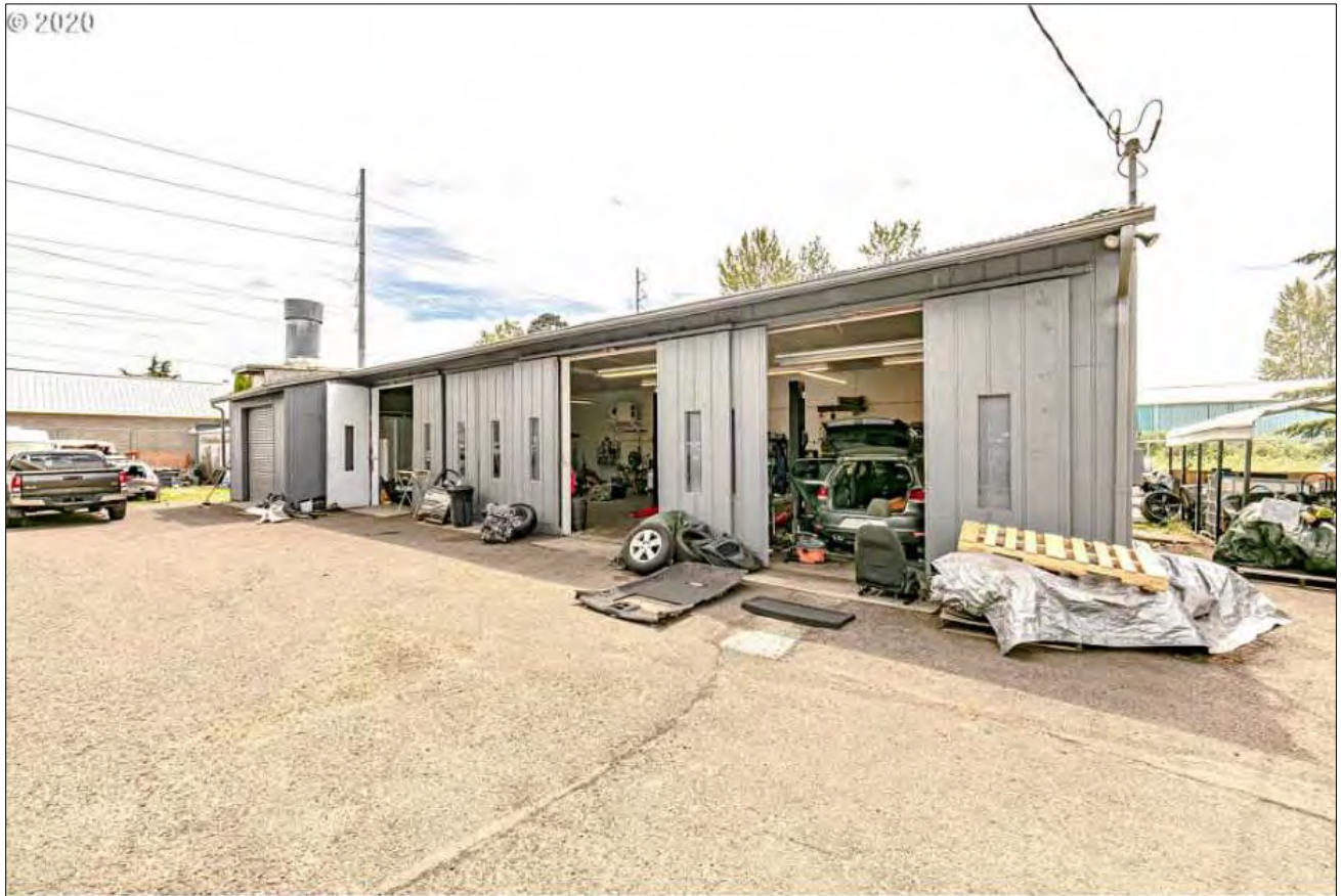
Figure 11. Garage 2, north elevation including sliding vehicular entrances, facing southeast (Zillow, 2020).
