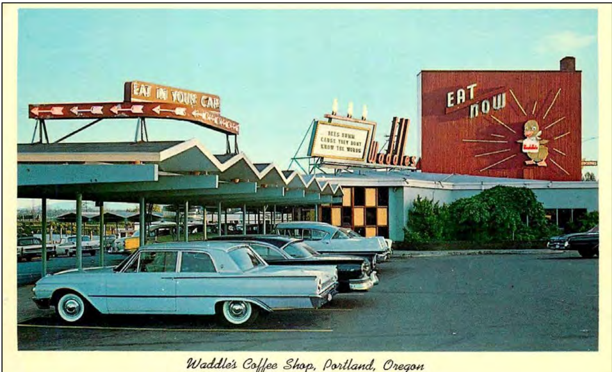
Figure 33. Postcard of Waddle's Drive-In Coffee Shop, view facing south. This image likely dates to the early 1960s, shortly after the completion of alterations begun in 1959 (eBay).
