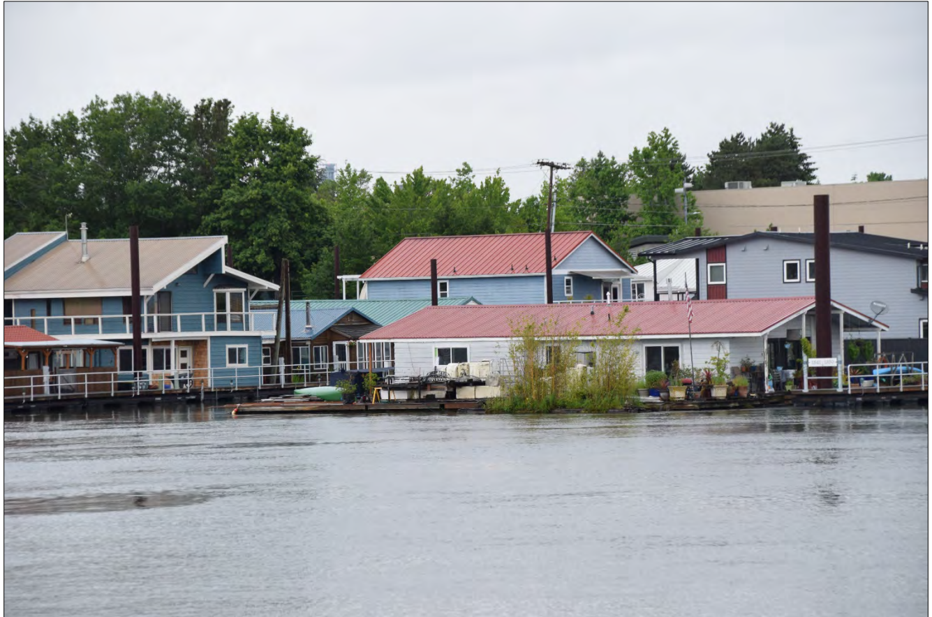
Figure 17. Jantzen Beach Moorage. View facing north (WillametteCRA June 10, 2022).
