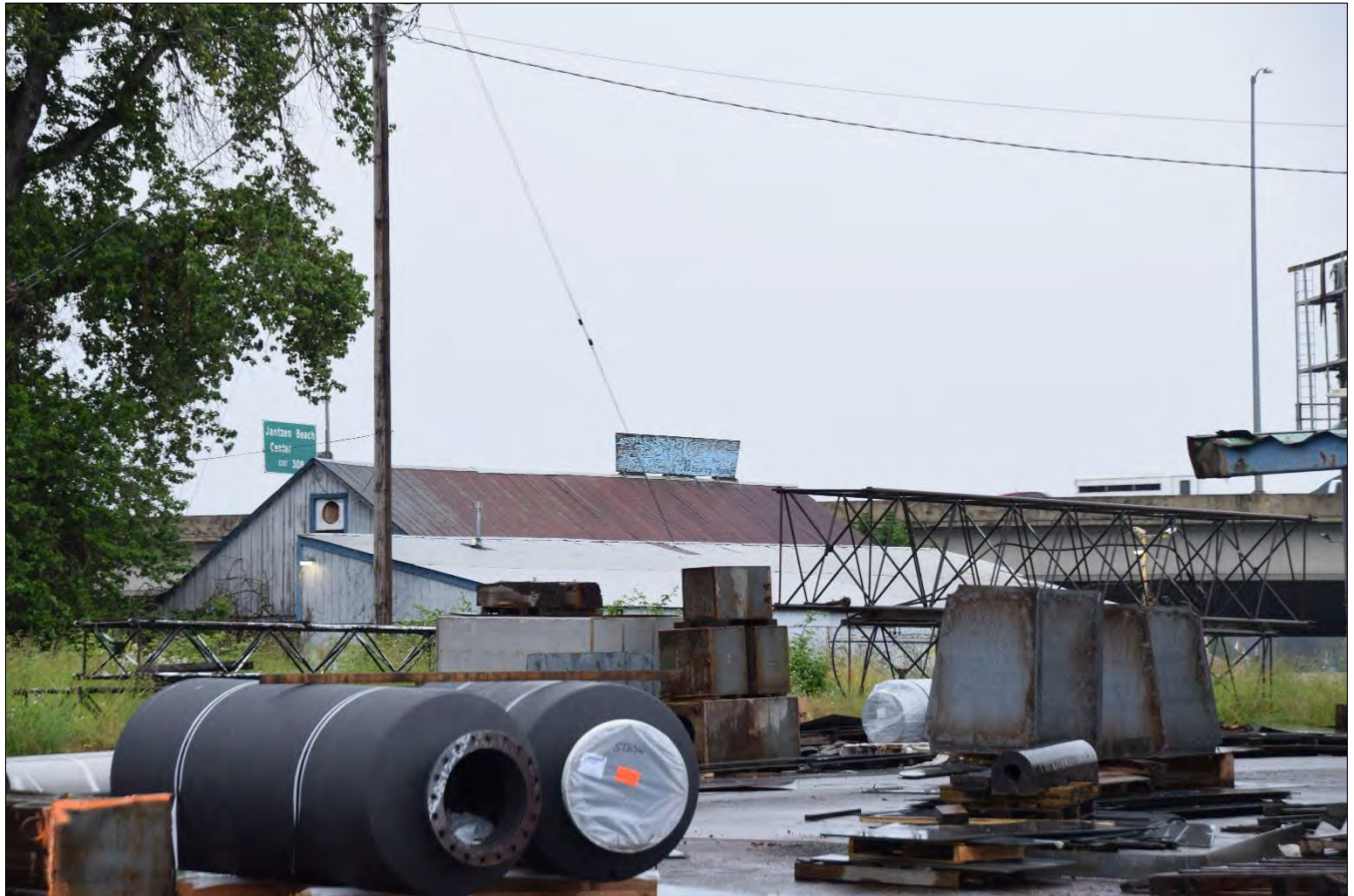
Figure 9. West and south elevations of the Westerlund Boat and Machine Shop, view facing northeast (WillametteCRA June 10, 2022).
