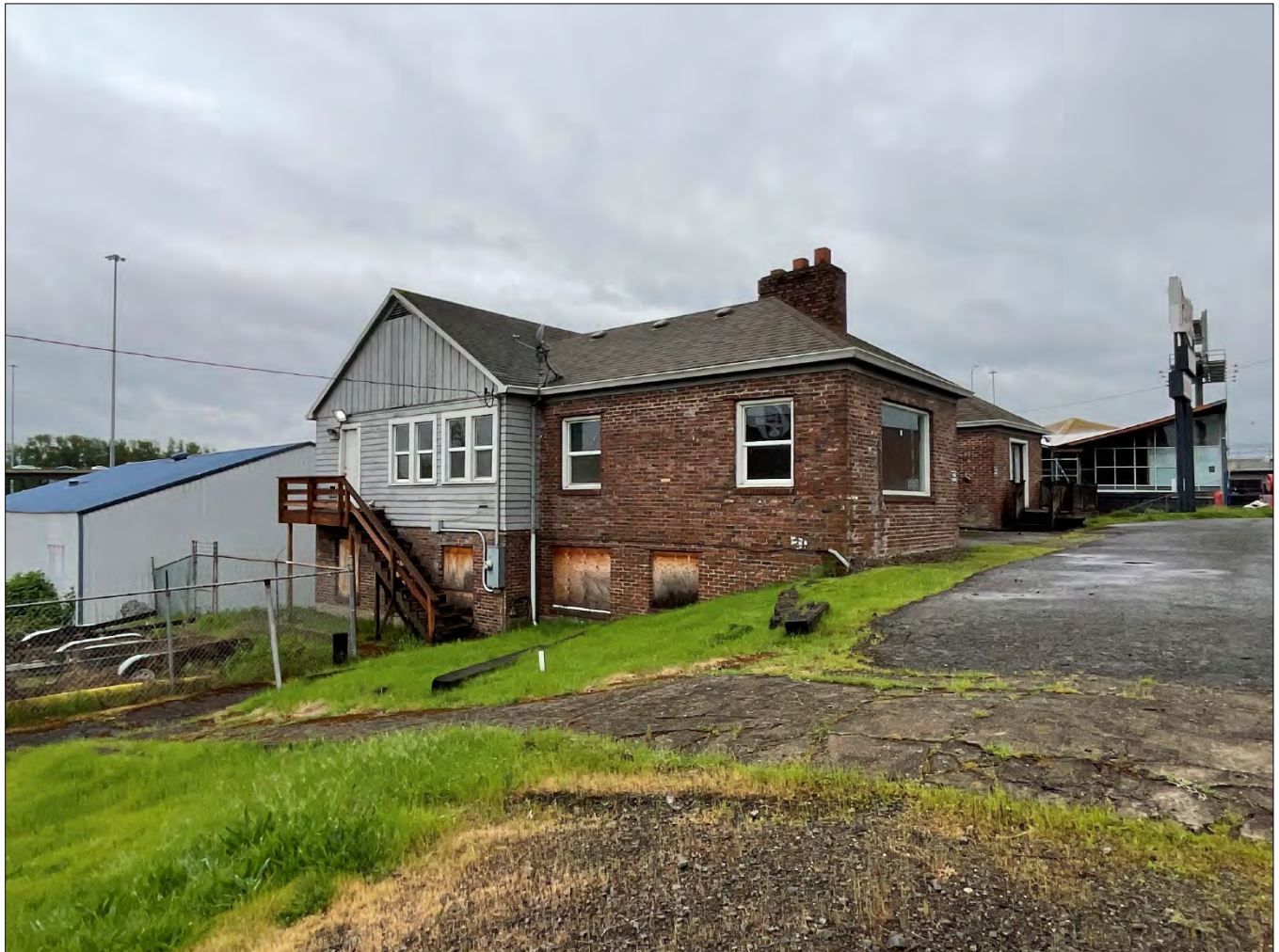
Figure 9. East elevation of the Gault house, view facing southwest (WillametteCRA May 4, 2023).
