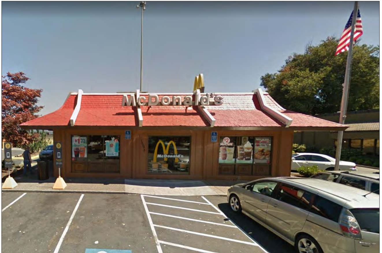
Figure 9. West elevation of the Jantzen Beach McDonald's, view facing east (Google Maps, July 2017).
