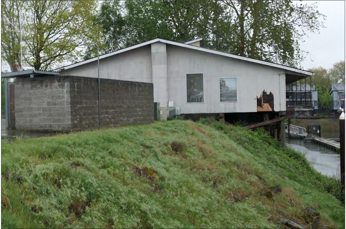
Figure 7. View of Hayden Island Yacht Club Clubhouse from south (WillametteCRA, May 4, 2023).
