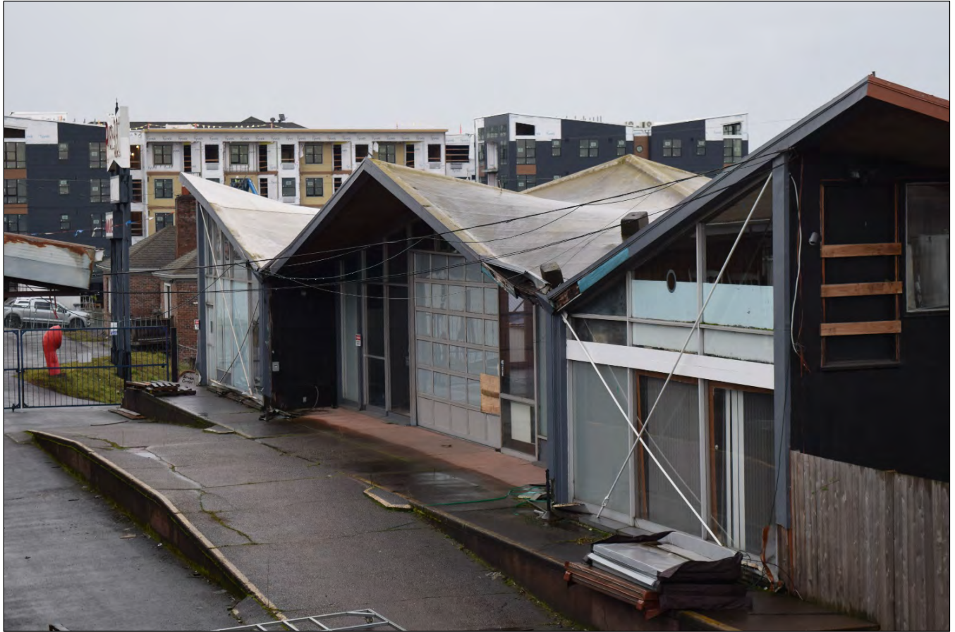
Figure 10. Concrete ramp and main entry, prior to demolition of second story and roof. View facing southeast (WillametteCRA January 16, 2023).
