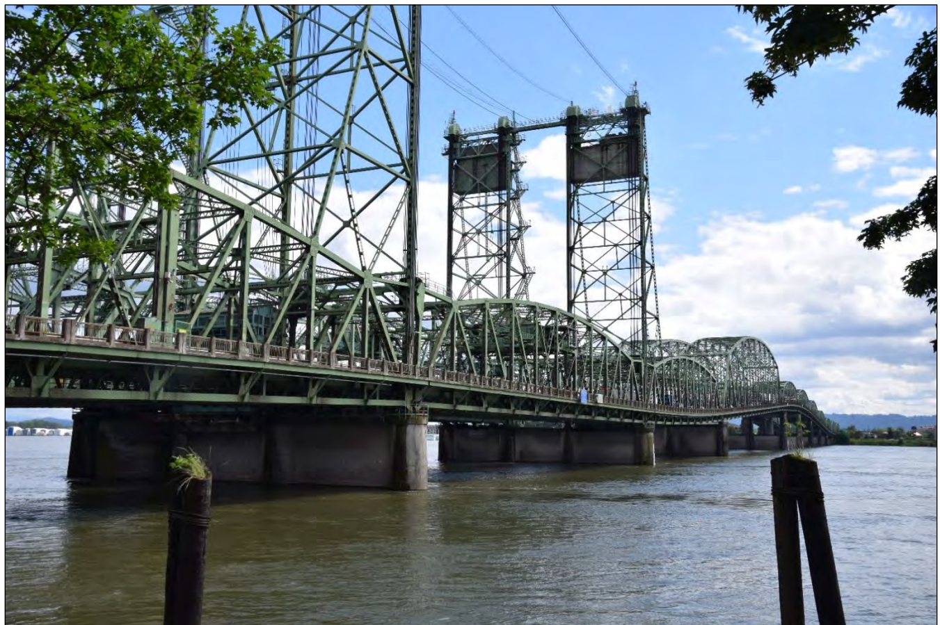
Figure 3. The Southbound Interstate 5 Columbia River Bridge. View facing south (WillametteCRA June 14, 2022).
