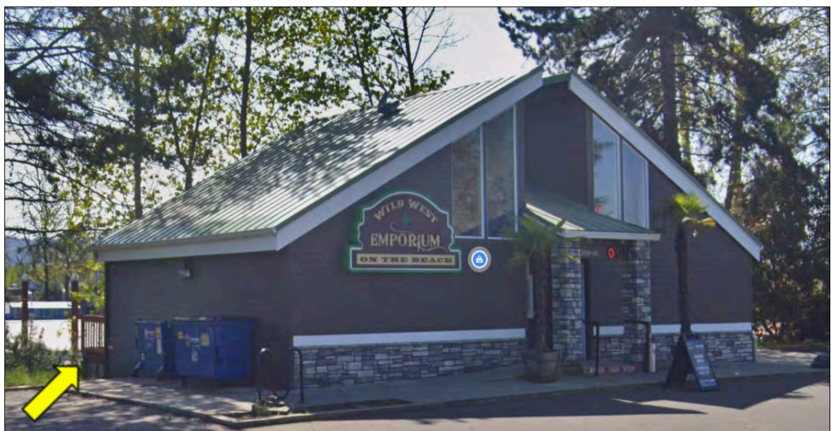
Figure 6. Northwest Marine Brokers Building, north and east elevations, view facing southwest. Arrow points to corner wooden deck (Google Street View, April 2022).
