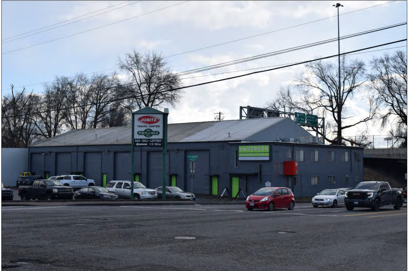
Figure 1. View of Rudy Yost Equipment, north and east elevations, view facing southwest (WillametteCRA March 8, 2023).
