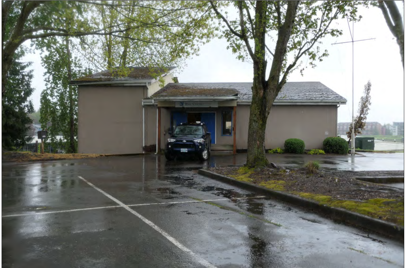
Figure 1. Hayden Island Yacht Club Clubhouse, north elevation, view facing southwest (WillametteCRA, May 4, 2023).
