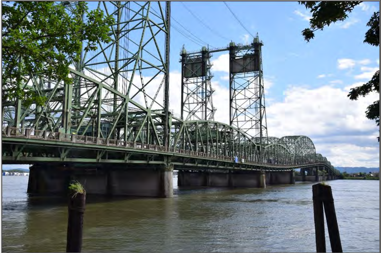
Figure 1. The Southbound Interstate 5 Columbia River Bridge. View facing south (WillametteCRA June 14, 2022).
