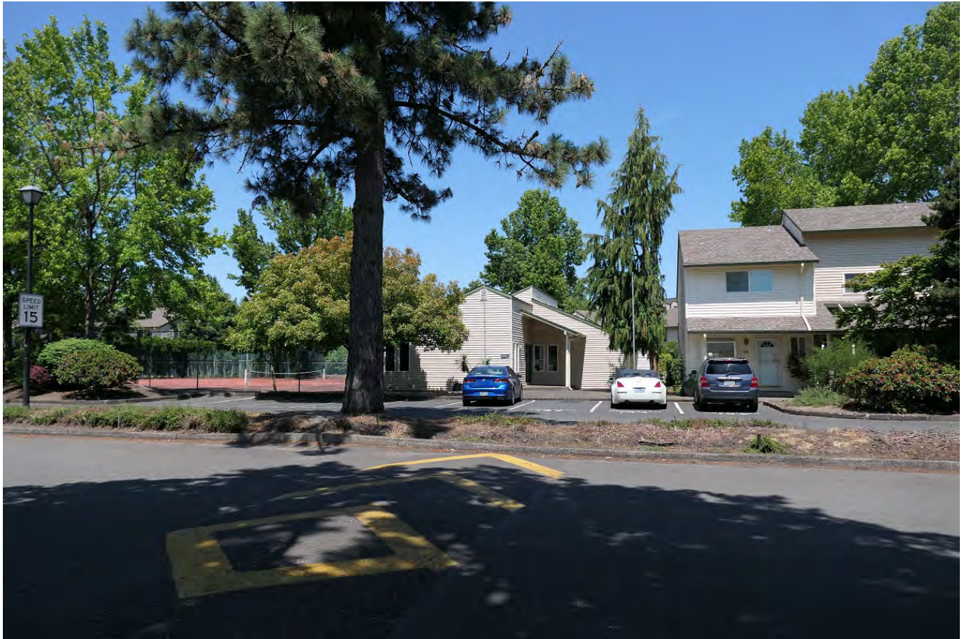
Figure 5. View of Jantzen Beach Village Condominiums from east, showing east recreation building (WillametteCRA, June 2023).
