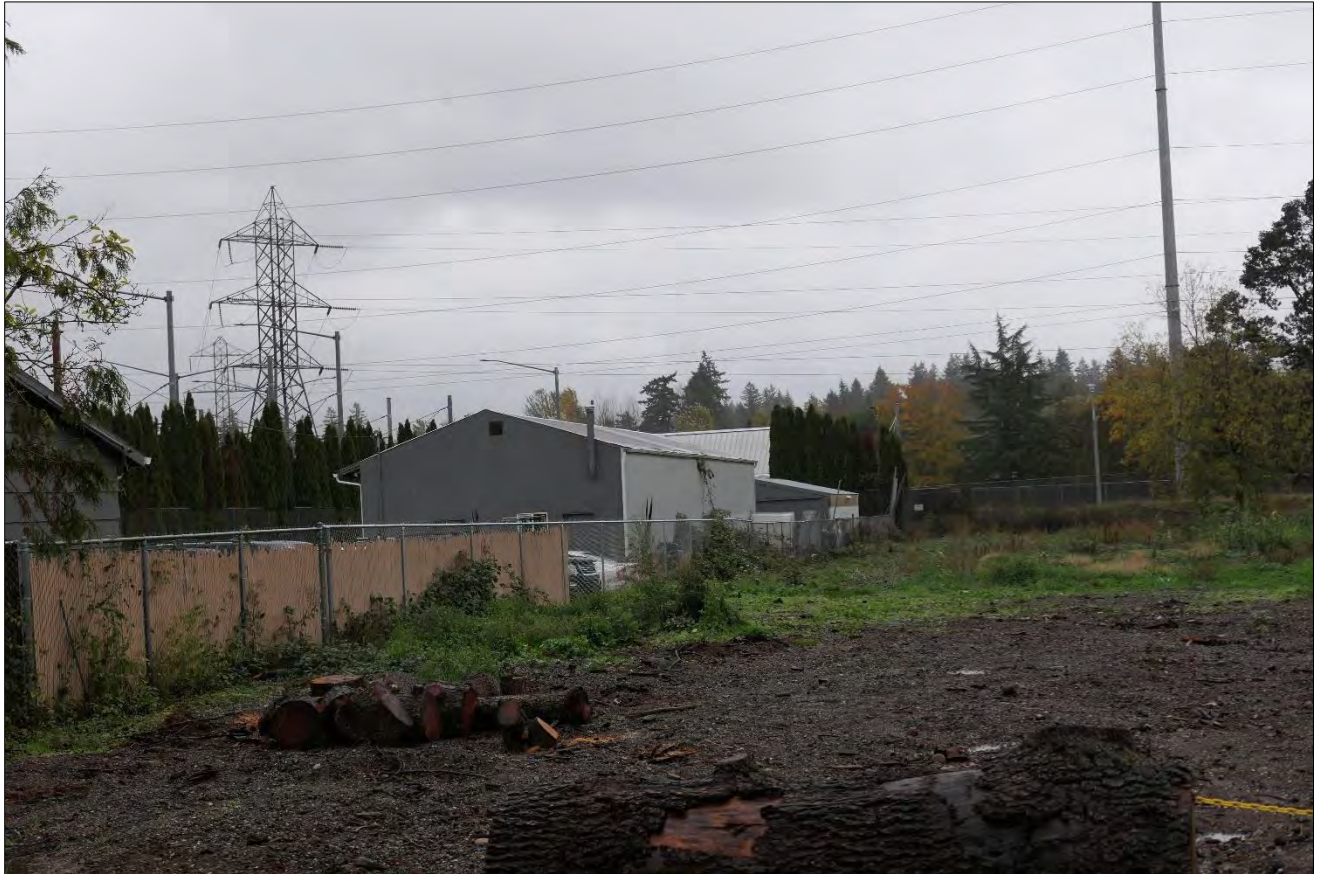
Figure 10. Garage 2, south and west elevations, facing northeast (WillametteCRA October 25, 2023).
