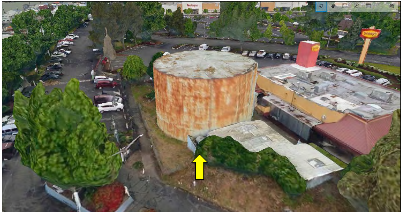
Figure 6. 3D rendering of the Jantzen Beach Water Tank and Pump House (center), view facing northwest. Arrow points to the backup diesel generator (Bentley, Summer 2022).
