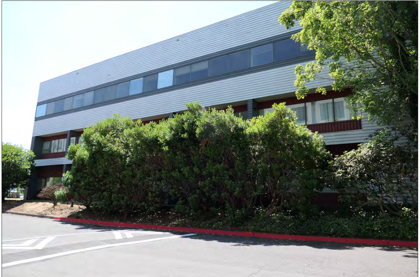
Figure 5. View of Hayden Island Plaza from north (WillametteCRA, June 2023).
