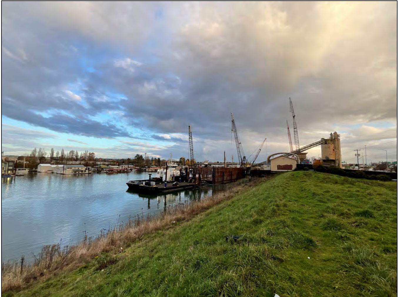
Figure 4. View of Vanport Pier from west (WillametteCRA, December 8, 2021).
