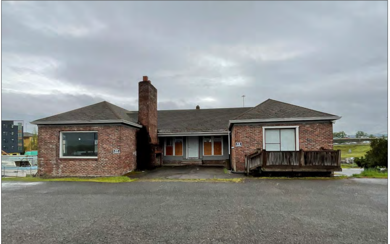
Figure 1. The Gault Residence at 1425 North Pier 99 Street, view facing south (WillametteCRA May 4, 2023).
