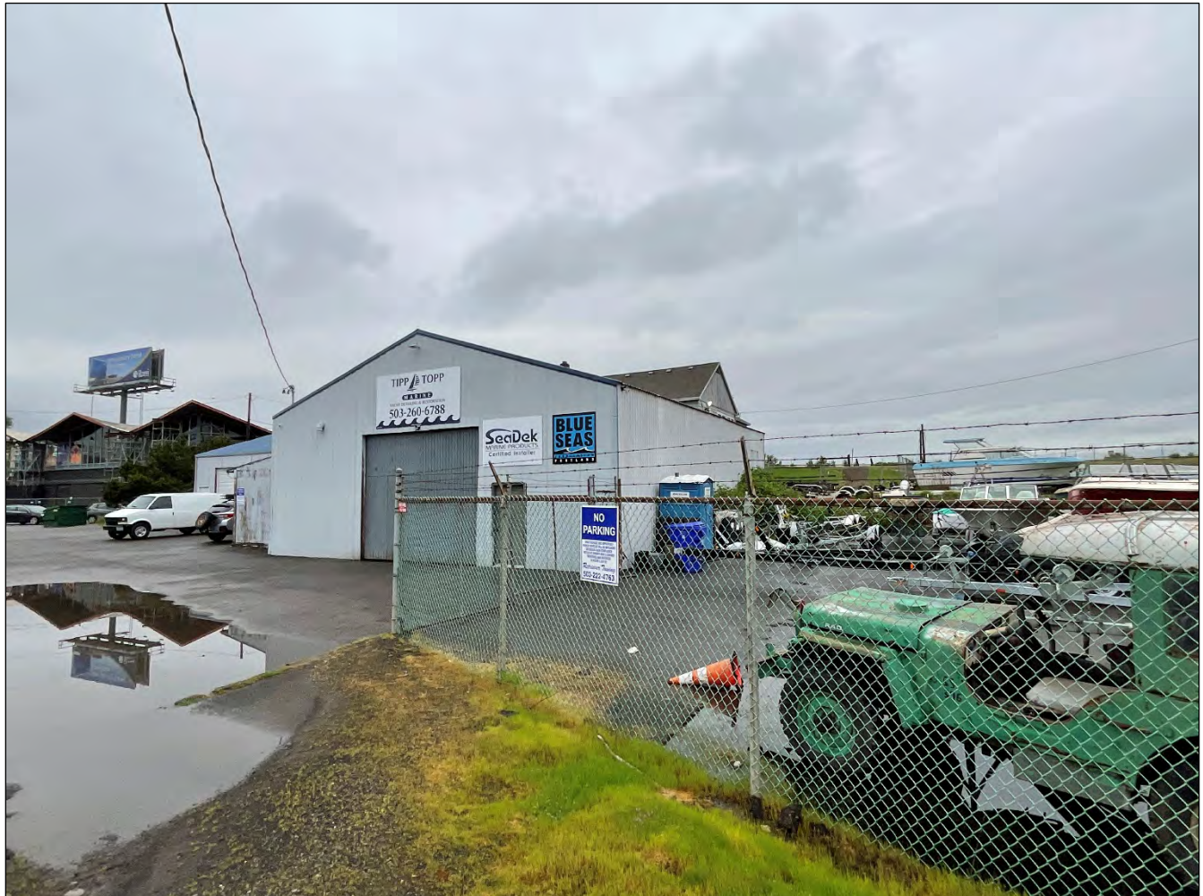
Figure 15. Tipp Topp Marine Building, view facing north (WillametteCRA May 4, 2023).
