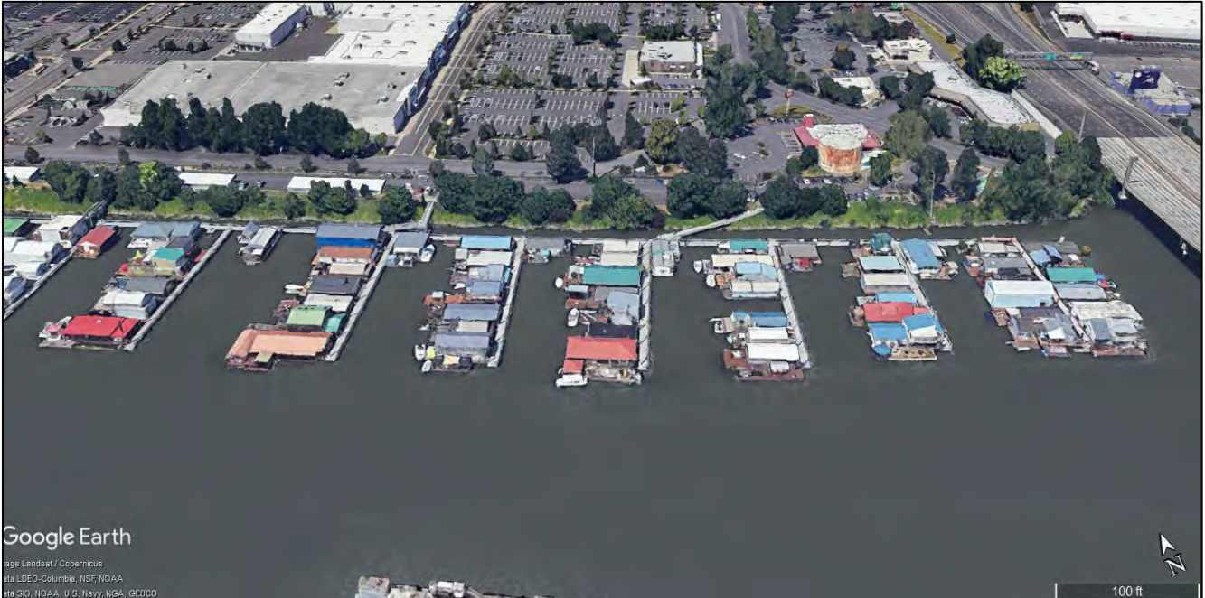
Figure 7. Jantzen Beach Moorage, Rows A, B, C, D, E, F, G from right to left. View facing north (Google Earth Pro 2023).
