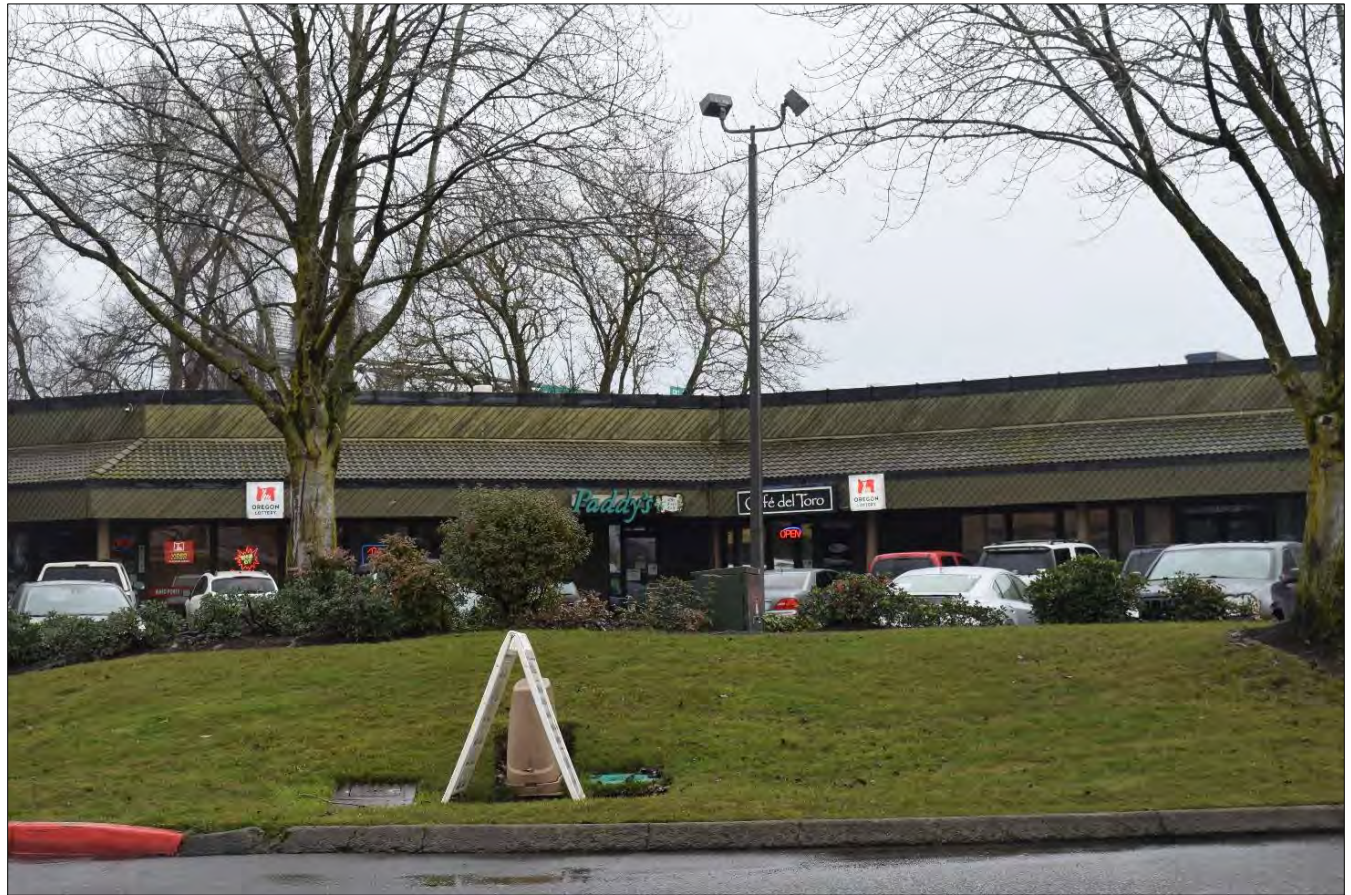
Figure 6. Partial west elevation of the “Harbor Shops” building, view facing east (WillametteCRA January 16, 2023).
