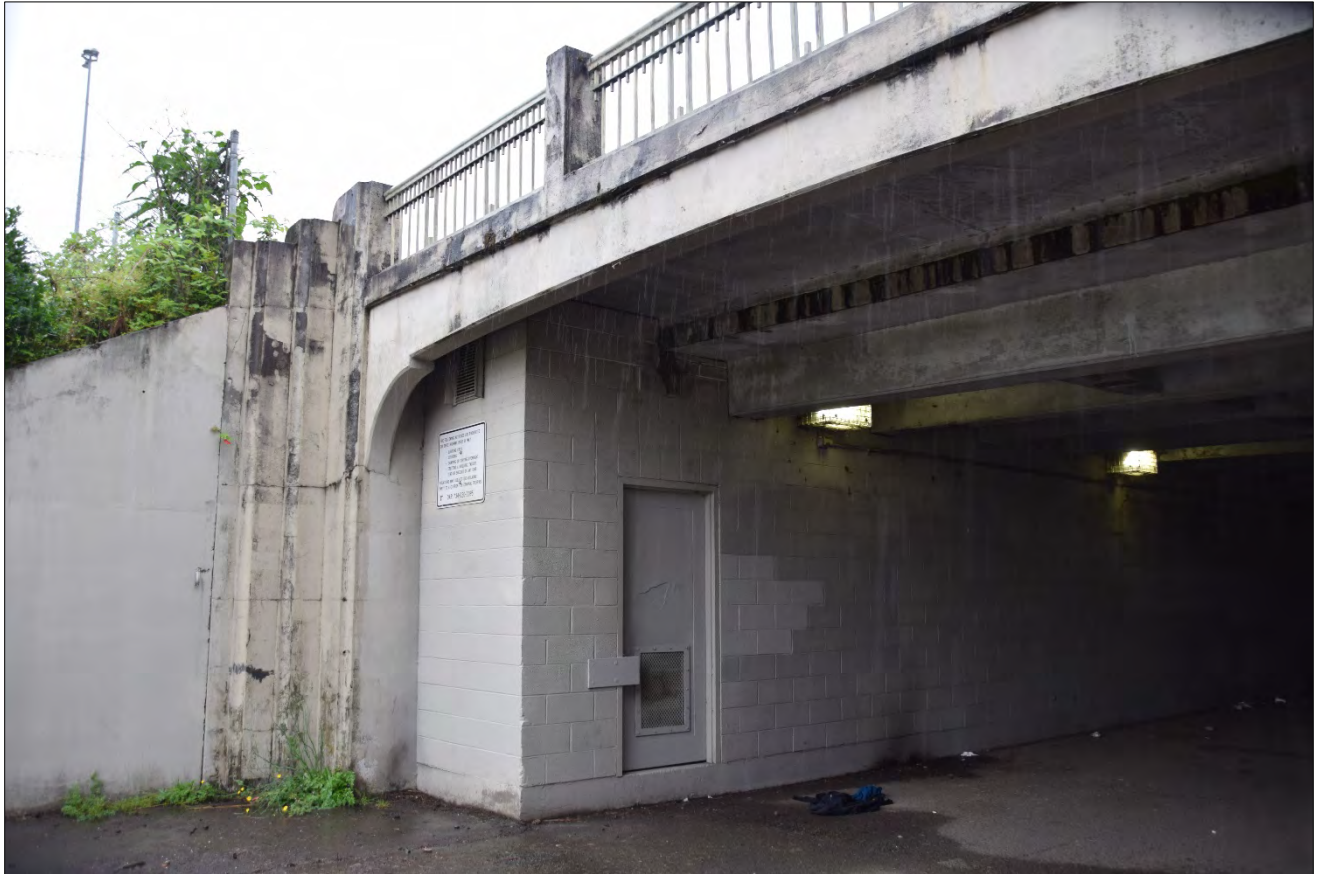
Figure 5. Jantzen Beach Pedestrian Tunnel, detail of west portal, view looking northeast (WillametteCRA June 10, 2022).
