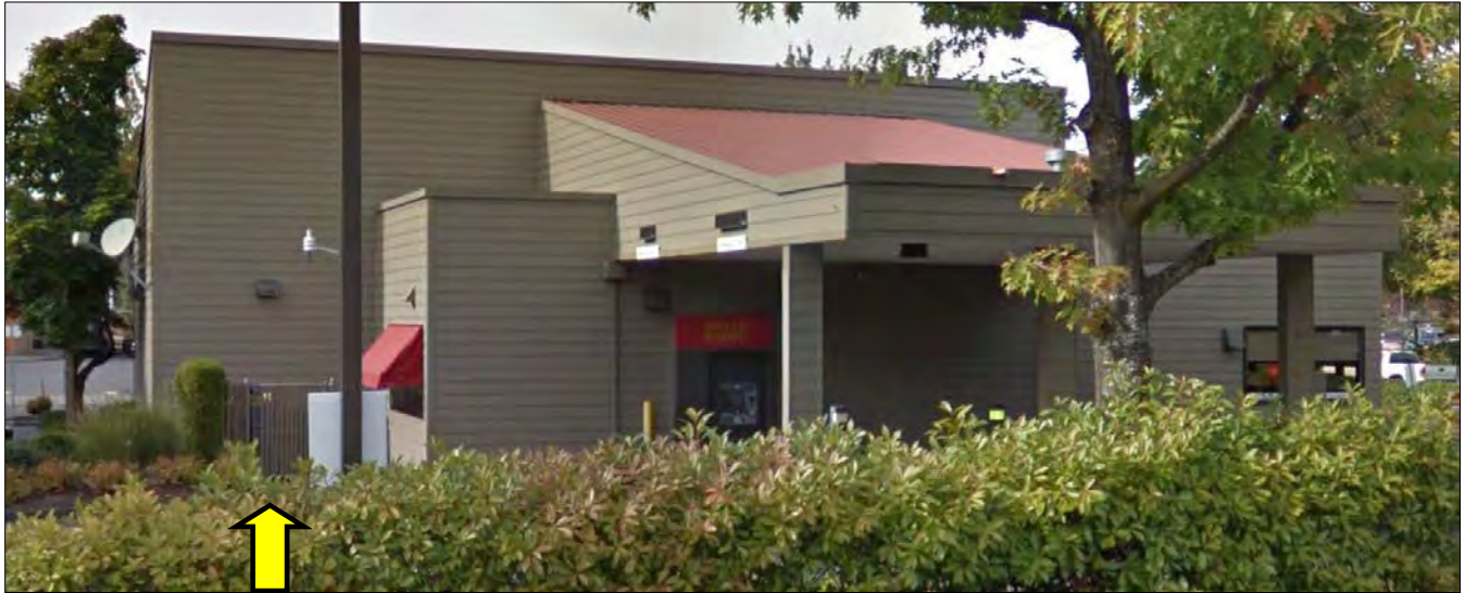
Figure 5. The First Interstate Bank Building, east elevation, view facing northwest. Arrow points to recessed utility meter area (Google Street View, October 2018).
