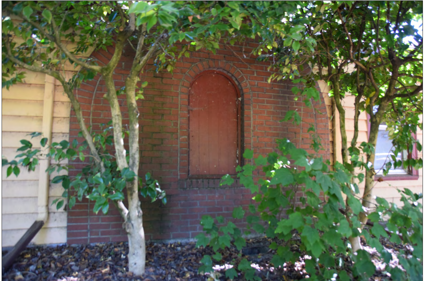
Figure 5. West elevation of Building at 10890 North Denver Ave, detail of brick chimney. View facing east (WillametteCRA September 6, 2022).
