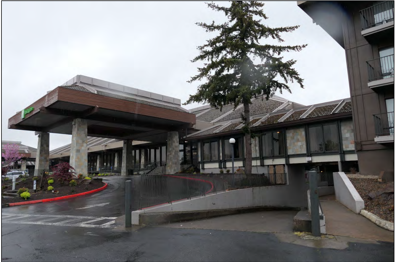
Figure 5. Overview of southwestern elevation. View facing northeast (WillametteCRA May 4, 2023).
