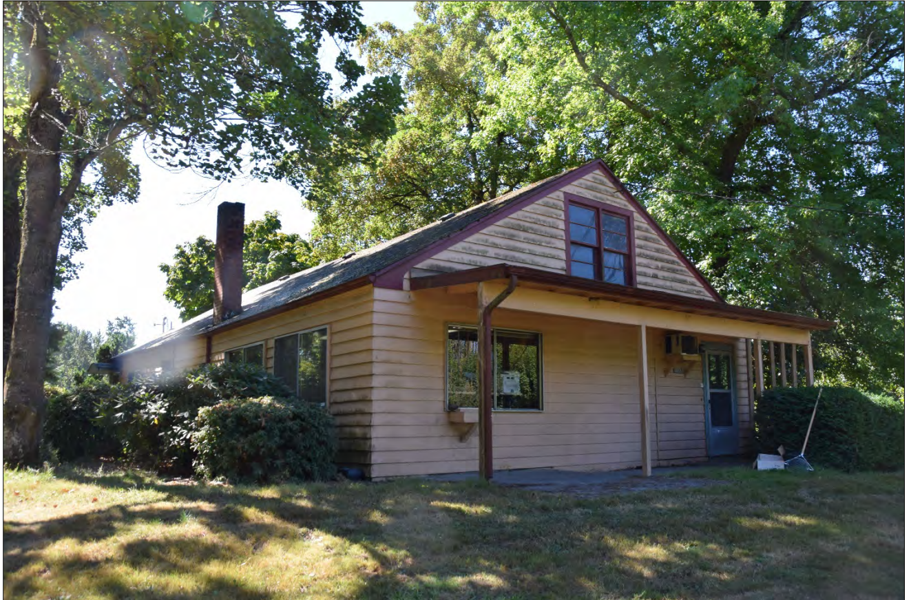
Figure 1. North and east elevations of 10890 N Denver Ave. The secondary entrance is located on the north elevation. View facing southwest (WillametteCRA, September 6, 2022).
