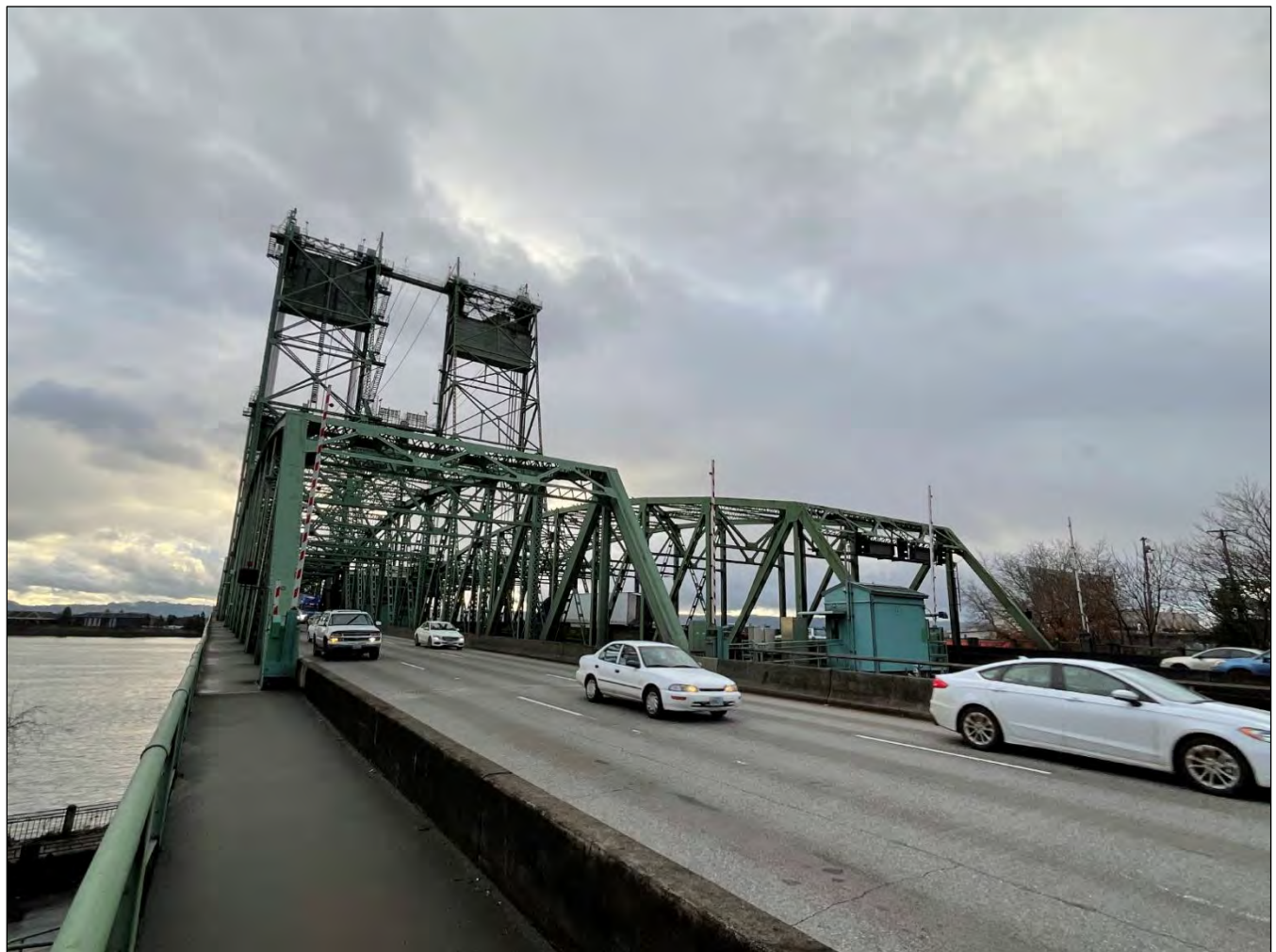
Figure 7. The north portal of the Northbound Interstate Bridge (left) and north portal of the Southbound Interstate 5 Columbia River Bridge (right). View facing south (WillametteCRA December 9, 2021).
