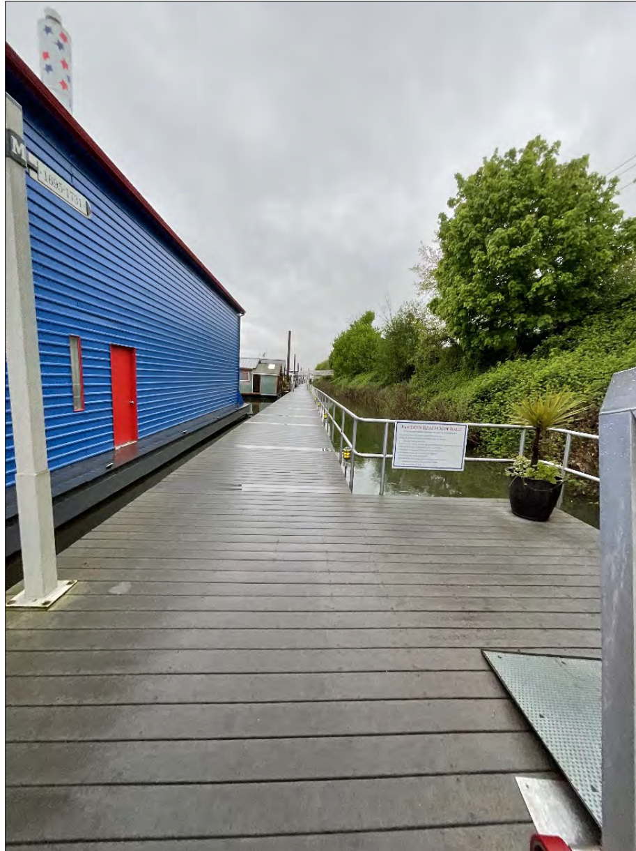
Figure 13. M Walk West. View facing west (WillametteCRA May 4, 2023).
