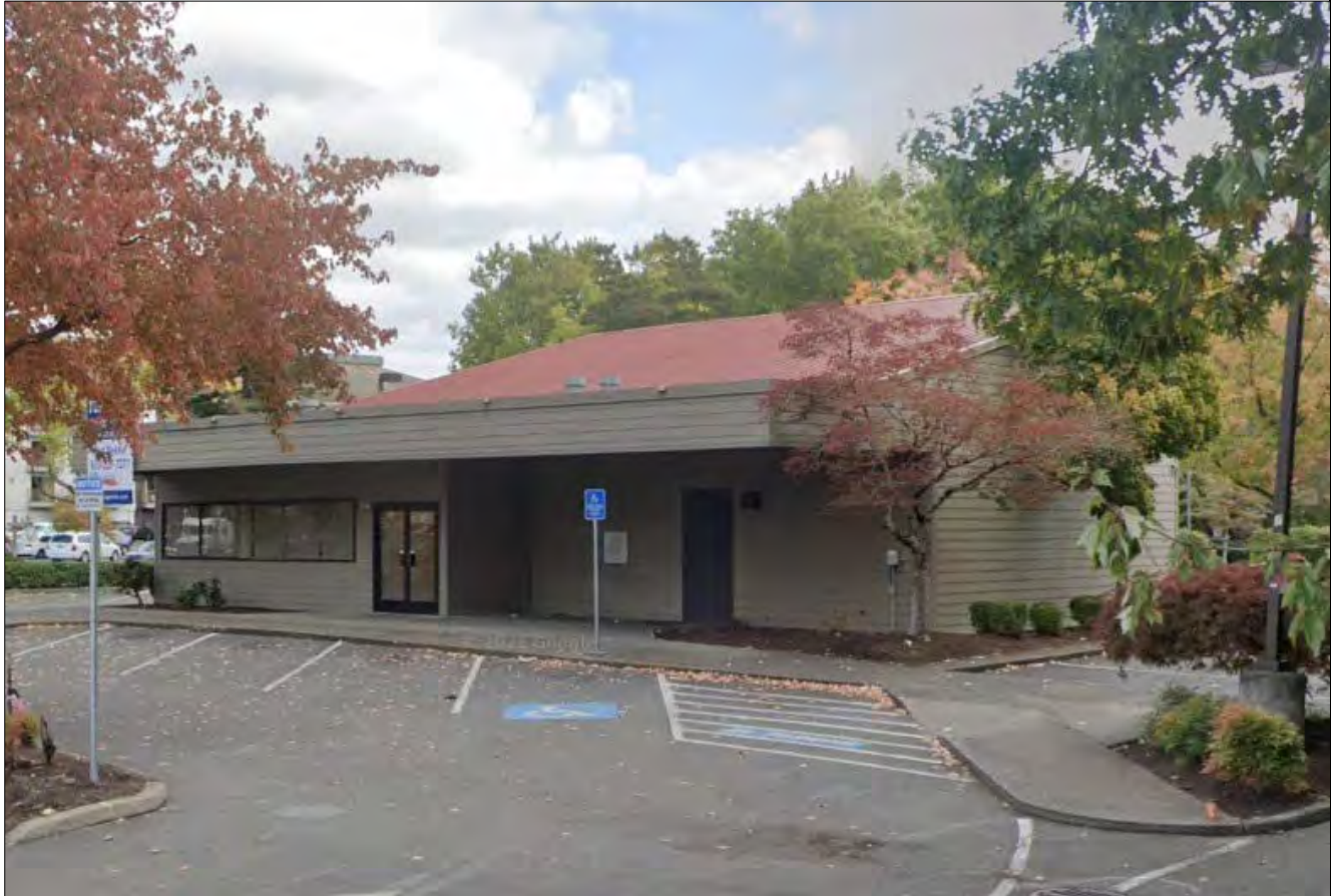
Figure 1. The First Interstate Bank Building, west elevation, view facing northeast. Note the two-section window at the far left is anodized and was added in 1984. The three-section window adjacent to it is not anodized and dates to the building's original construction. It was repurposed and moved forward from its original position in 1984 (WillametteCRA, February 26, 2022).
