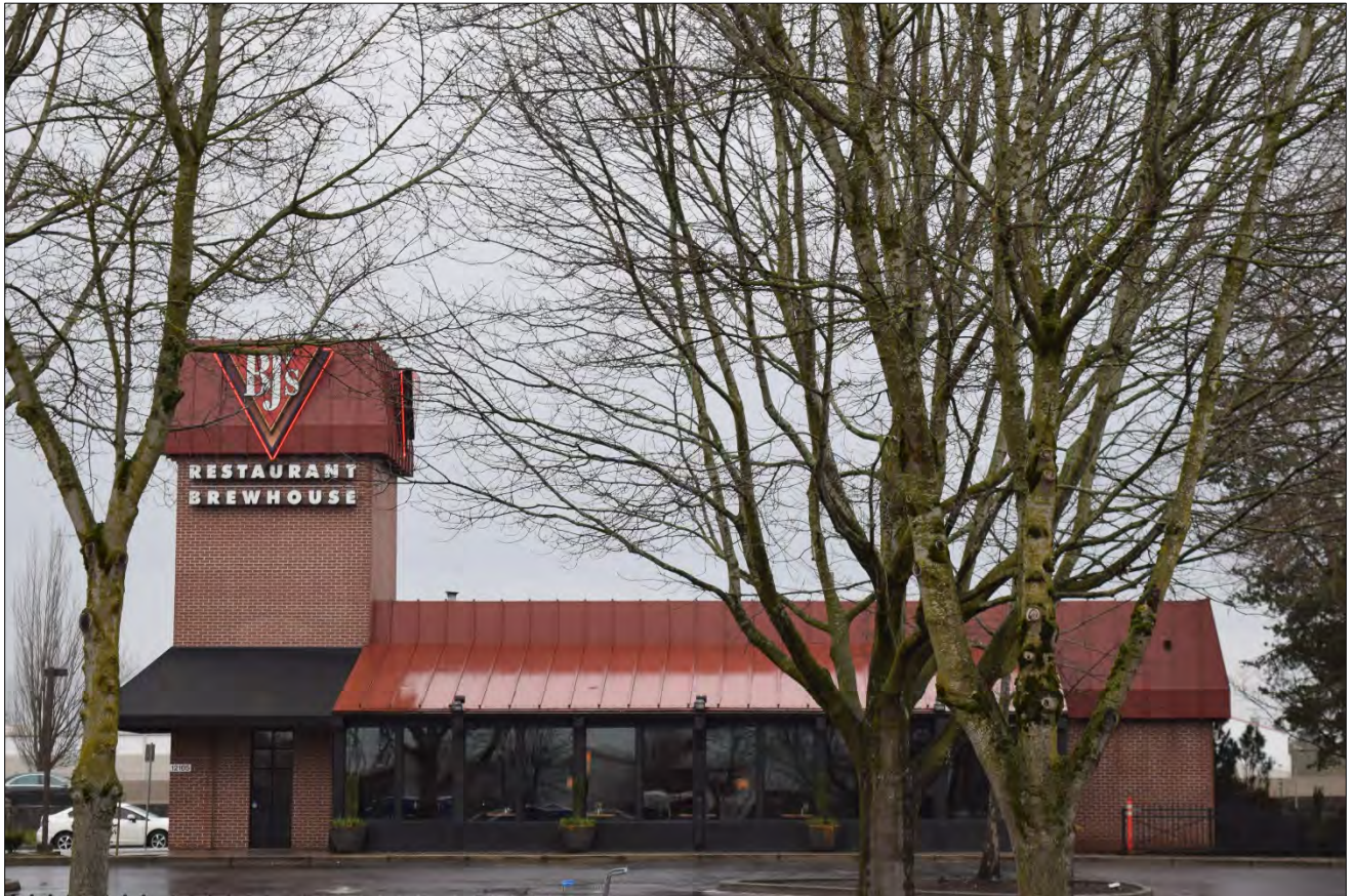
Figure 5. Engine House Pizza Co. #1, west elevation, view facing east (WillametteCRA April 30, 2023).
