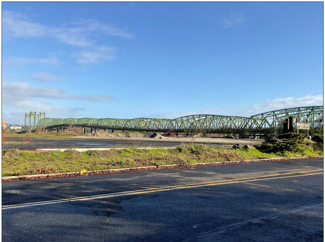
Figure 4. The Southbound Interstate 5 Columbia River Bridge. View facing north (WillametteCRA December 8, 2021).
