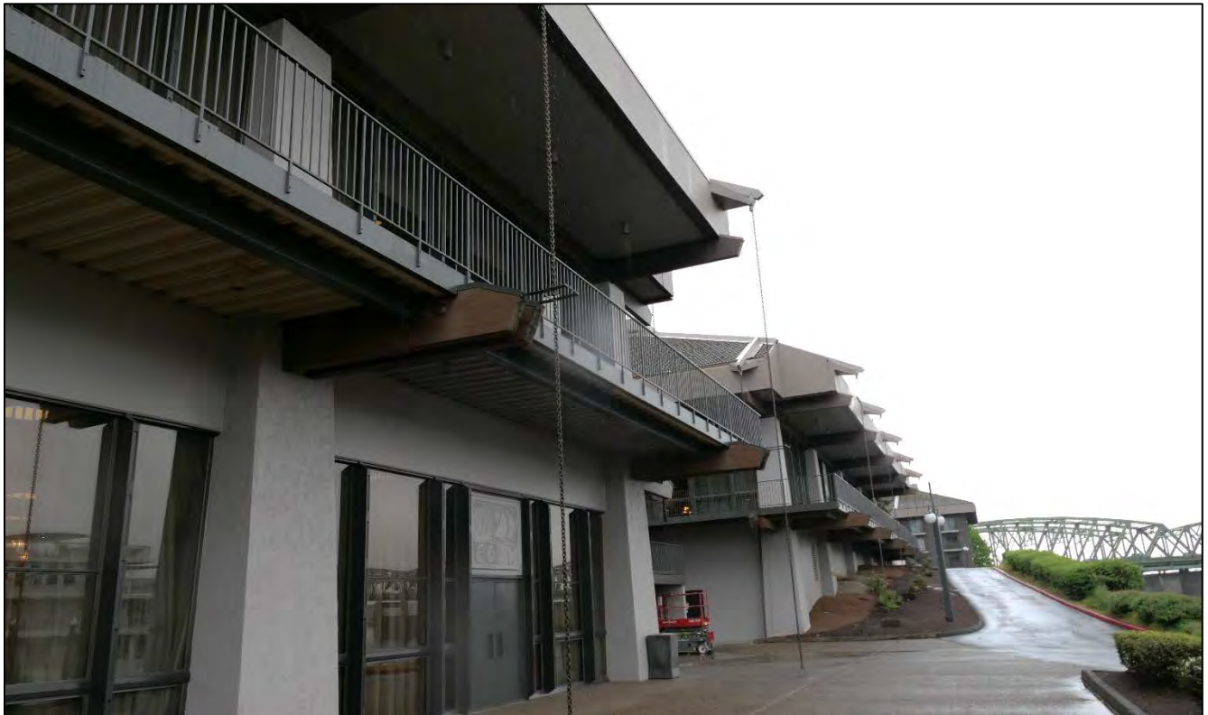
Figure 16. North elevation of banquet hall, with second-floor balcony. View facing west (WillametteCRA May 4, 2023).
