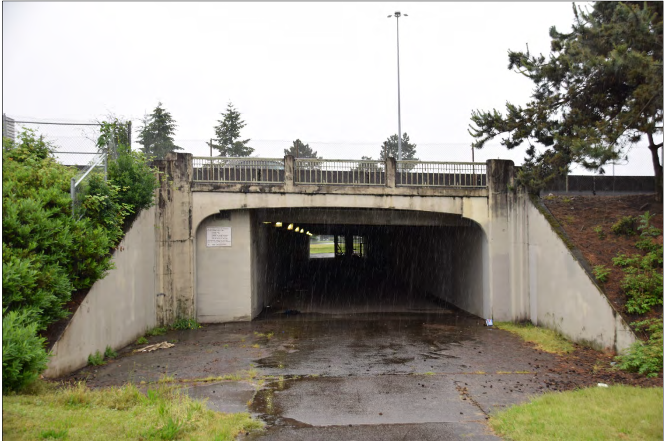
Figure 4. Jantzen Beach Pedestrian Tunnel, west portal, view looking east (WillametteCRA June 10, 2022).
