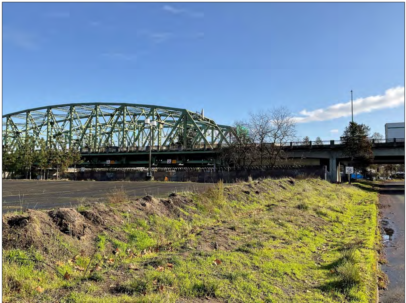
Figure 5. South portal of the Southbound Interstate 5 Columbia River Bridge. View facing east (WillametteCRA December 8, 2021).
