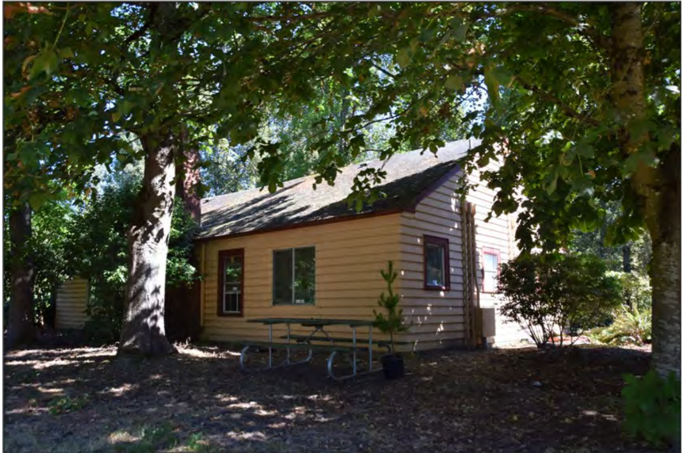
Figure 7. West and south elevations, including detail of historic windows set in wooden casing and newer windows. View facing northwest (WillametteCRA September 6, 2022).
