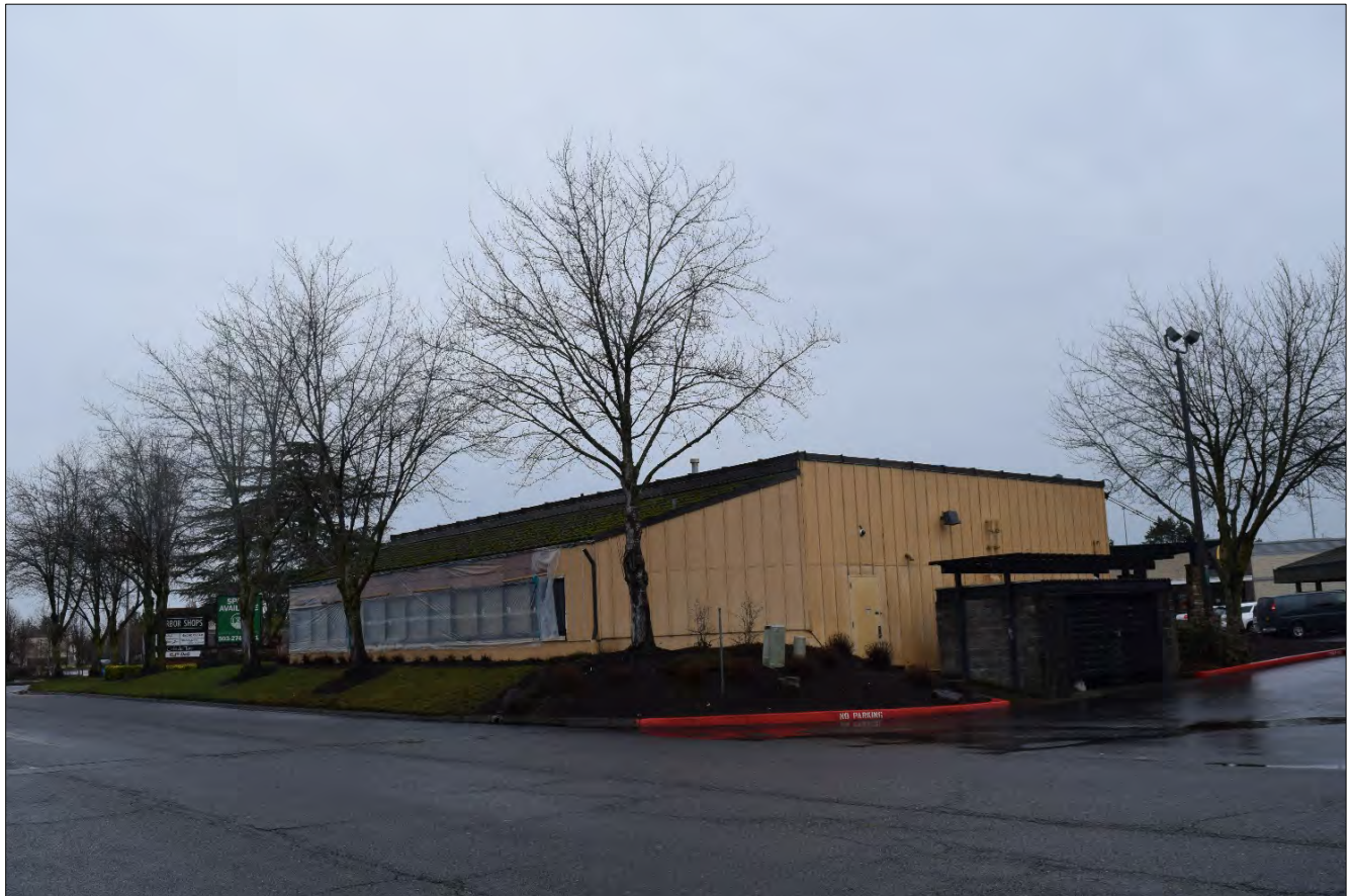
Figure 6. View of 12055 North Center Avenue from the southwest (WillametteCRA January 13, 2023).
