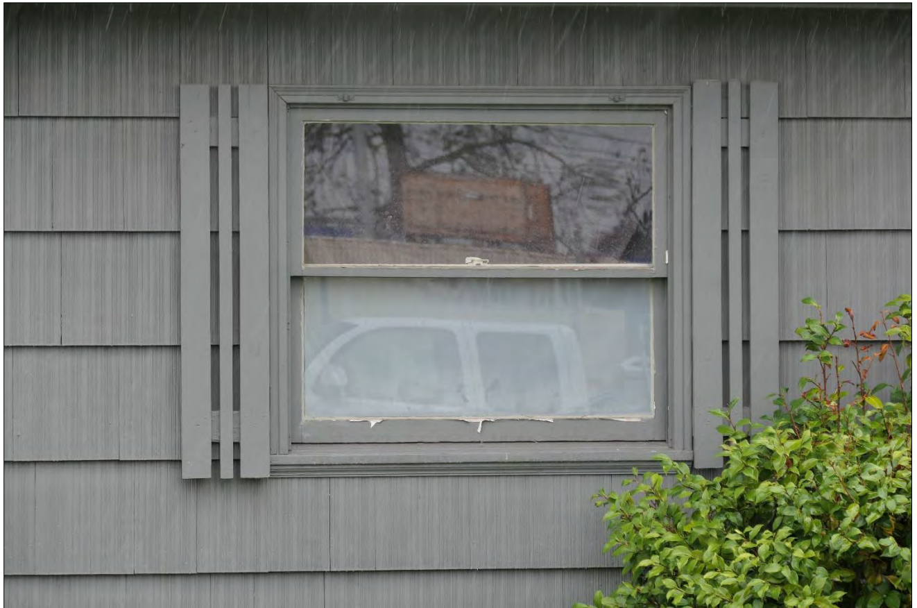
Figure 7. Residence, west elevation, detail of sash window, facing east (WillametteCRA October 25, 2023).
