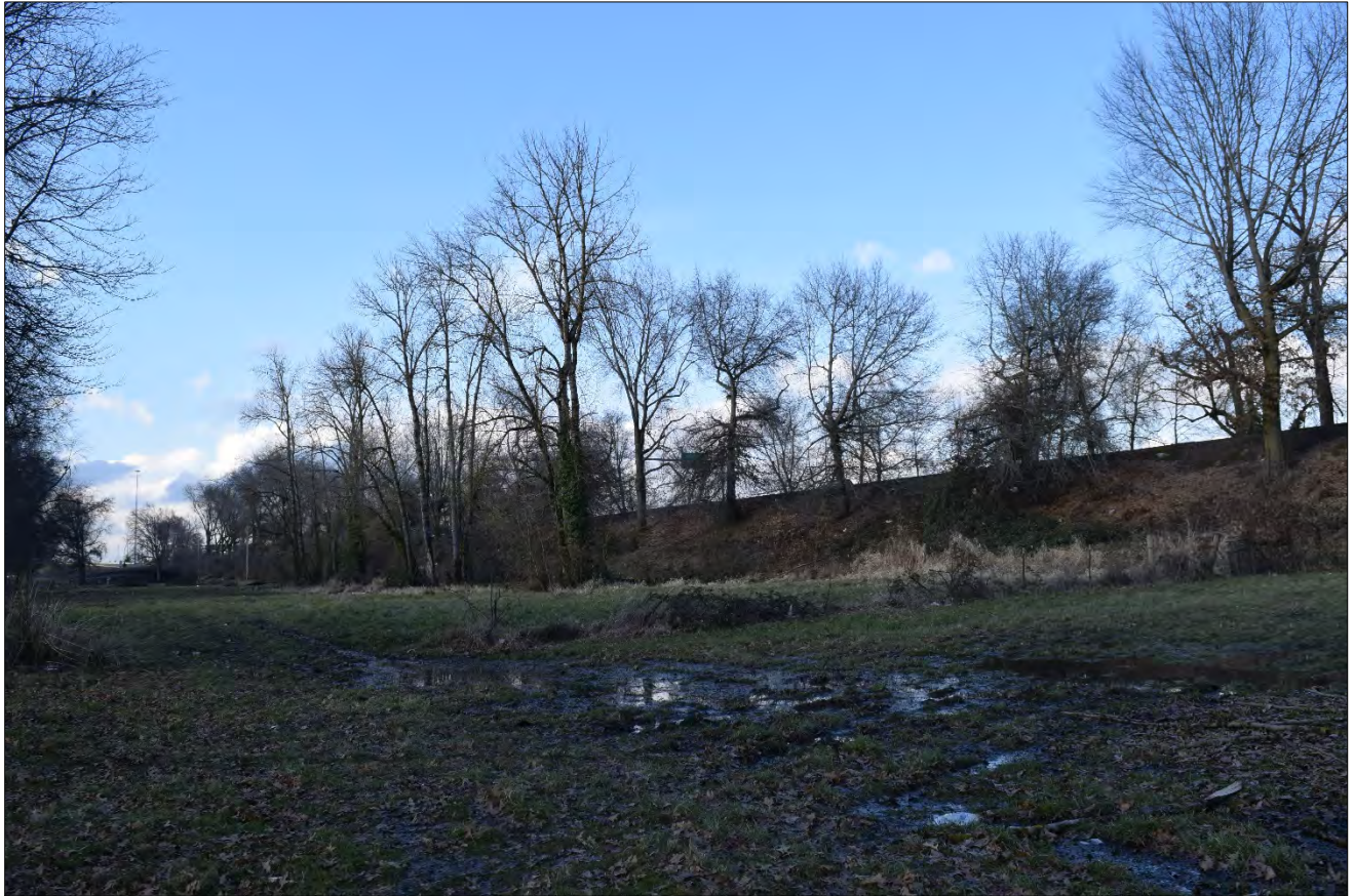
Figure 16. View of the Union Avenue/MLK Jr. Boulevard Cross Levee, south side, view facing northwest (WillametteCRA March 8, 2023).
