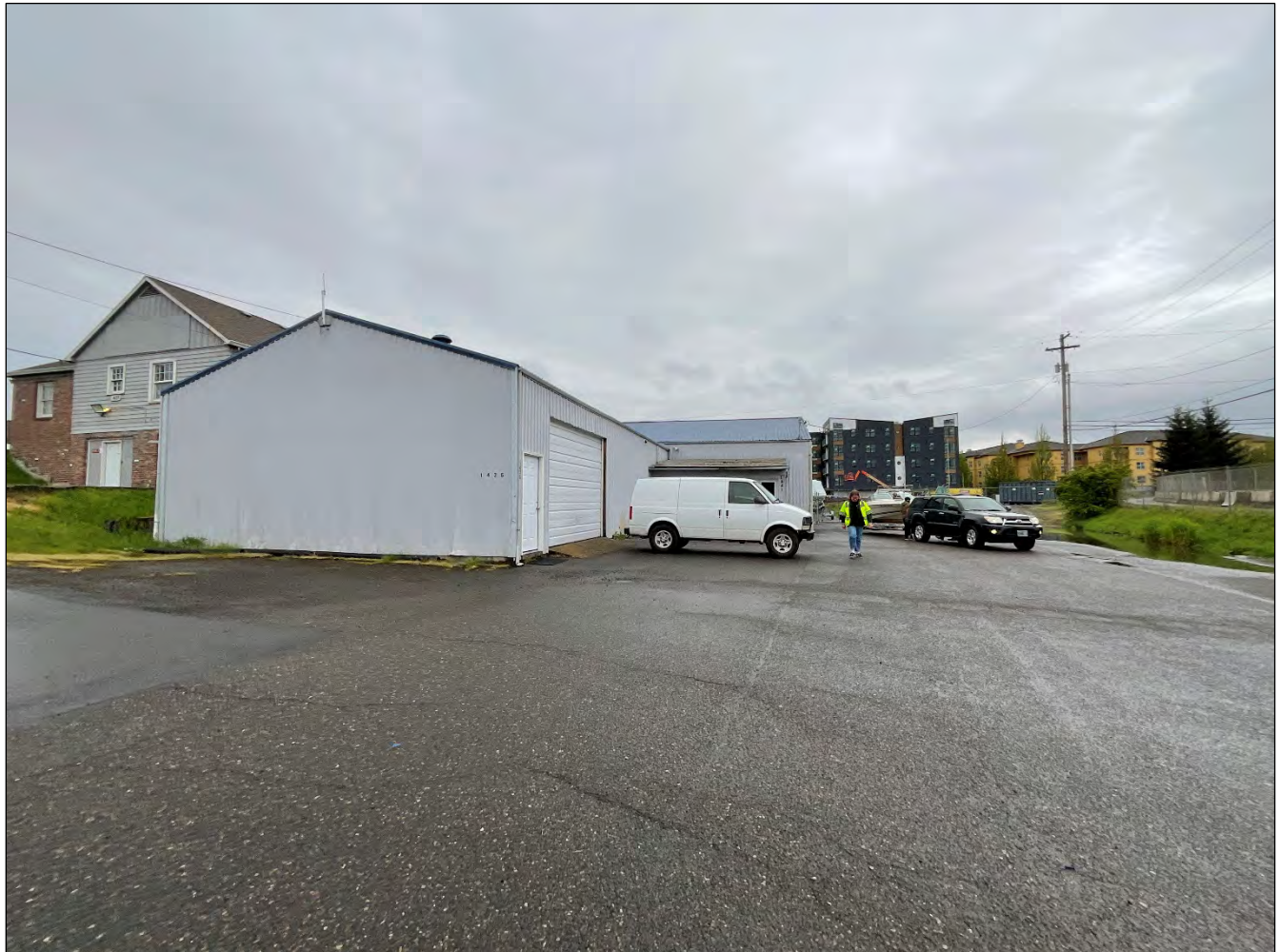
Figure 14. Tipp Topp Marine Building, view facing east (WillametteCRA May 4, 2023).
