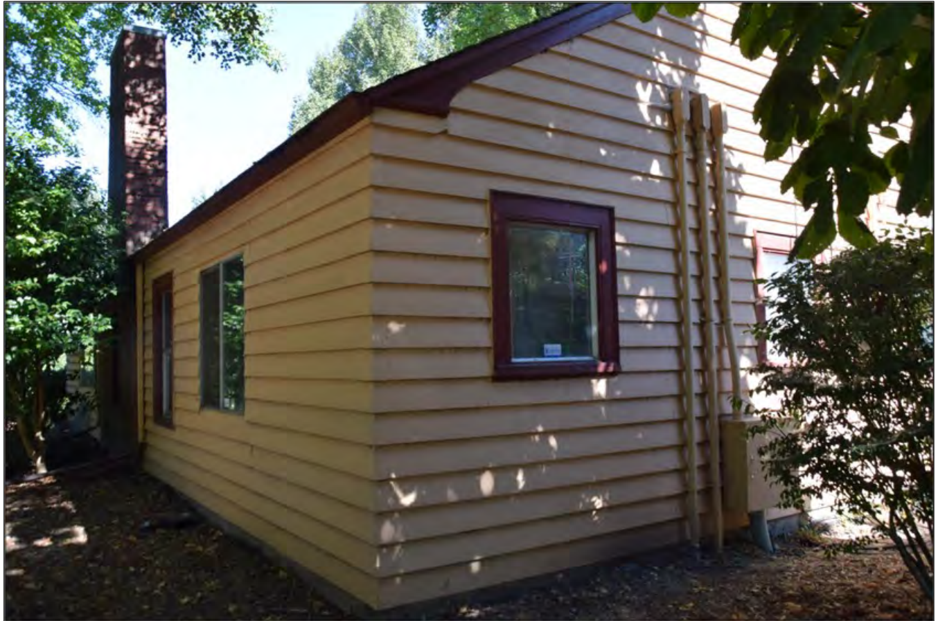
Figure 4. West and south elevations of 10890 North Denver Ave, including detail of trim and historic windows set in wooden casing and newer windows. View facing northeast (WillametteCRA September 6, 2022).
