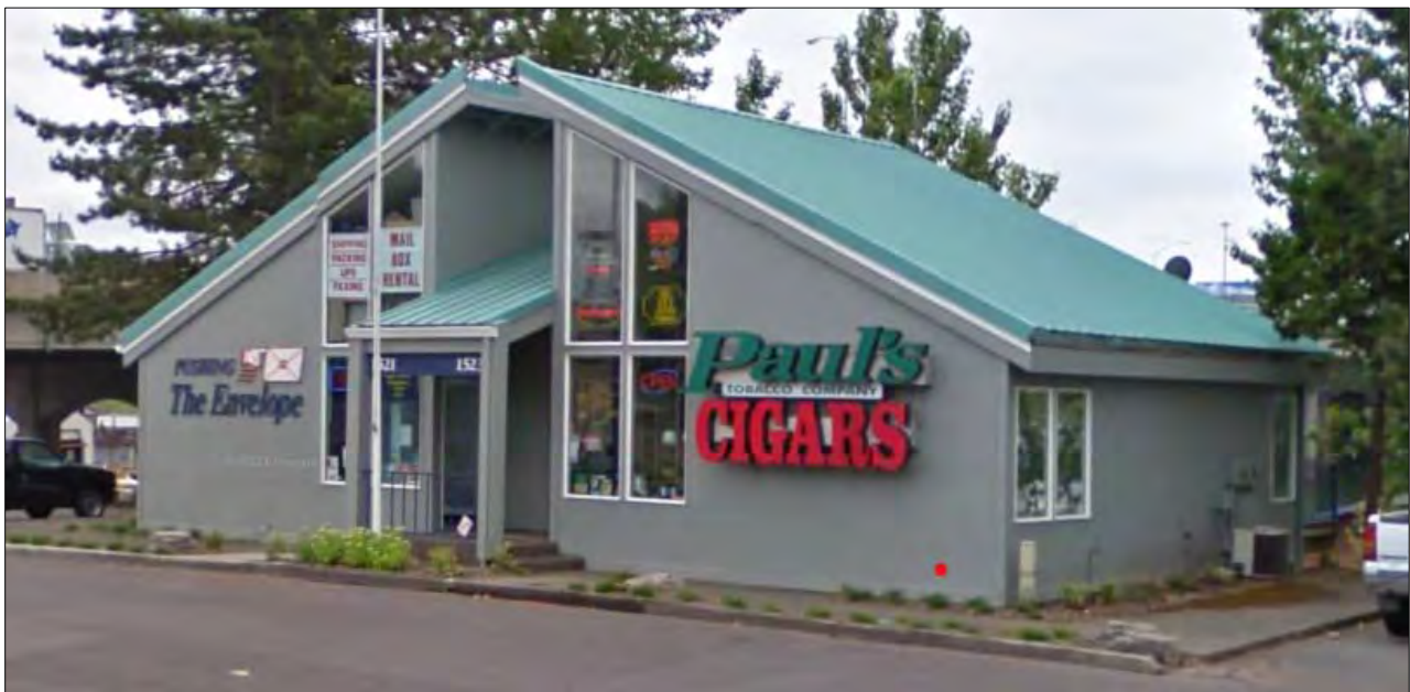
5 Figure 10. 2009 photograph of the building, view facing southwest. Note the since removed windows on the west (side) elevation (Google Street View, 2009).
