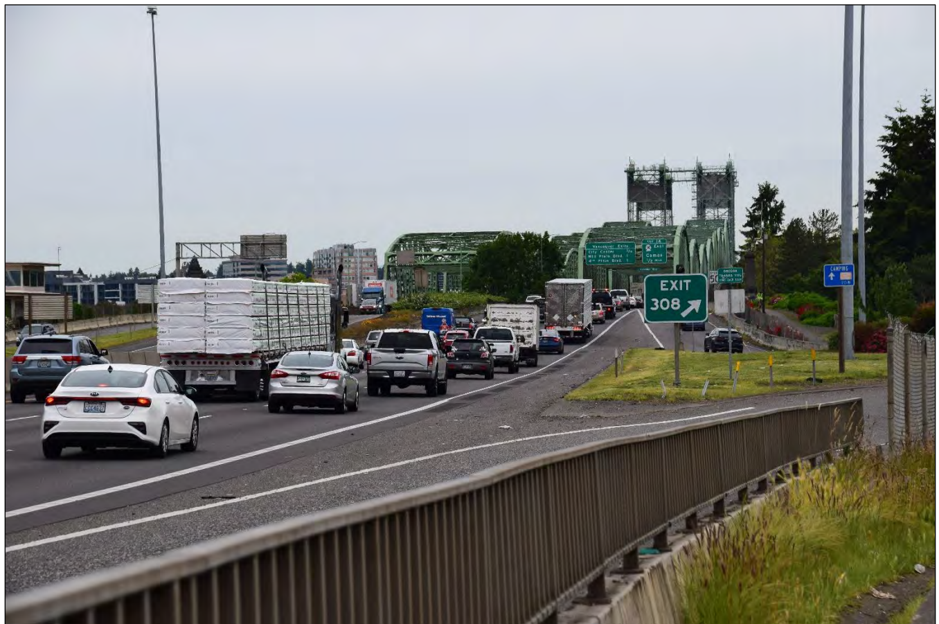
Figure 6. South approach of the Southbound Interstate 5 Columbia River Bridge. View facing north (WillametteCRA June 7, 2022).
