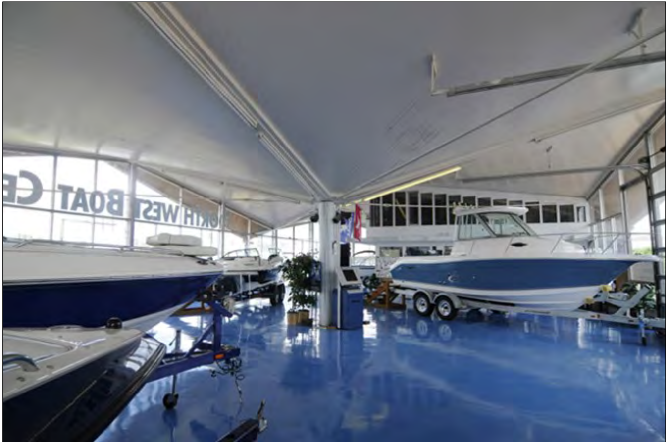
Figure 7. Interior view of 1415 North Pier 99 Street prior to demolition of second story and roof ( Daily Journal of Commerce , June 15, 2011).
