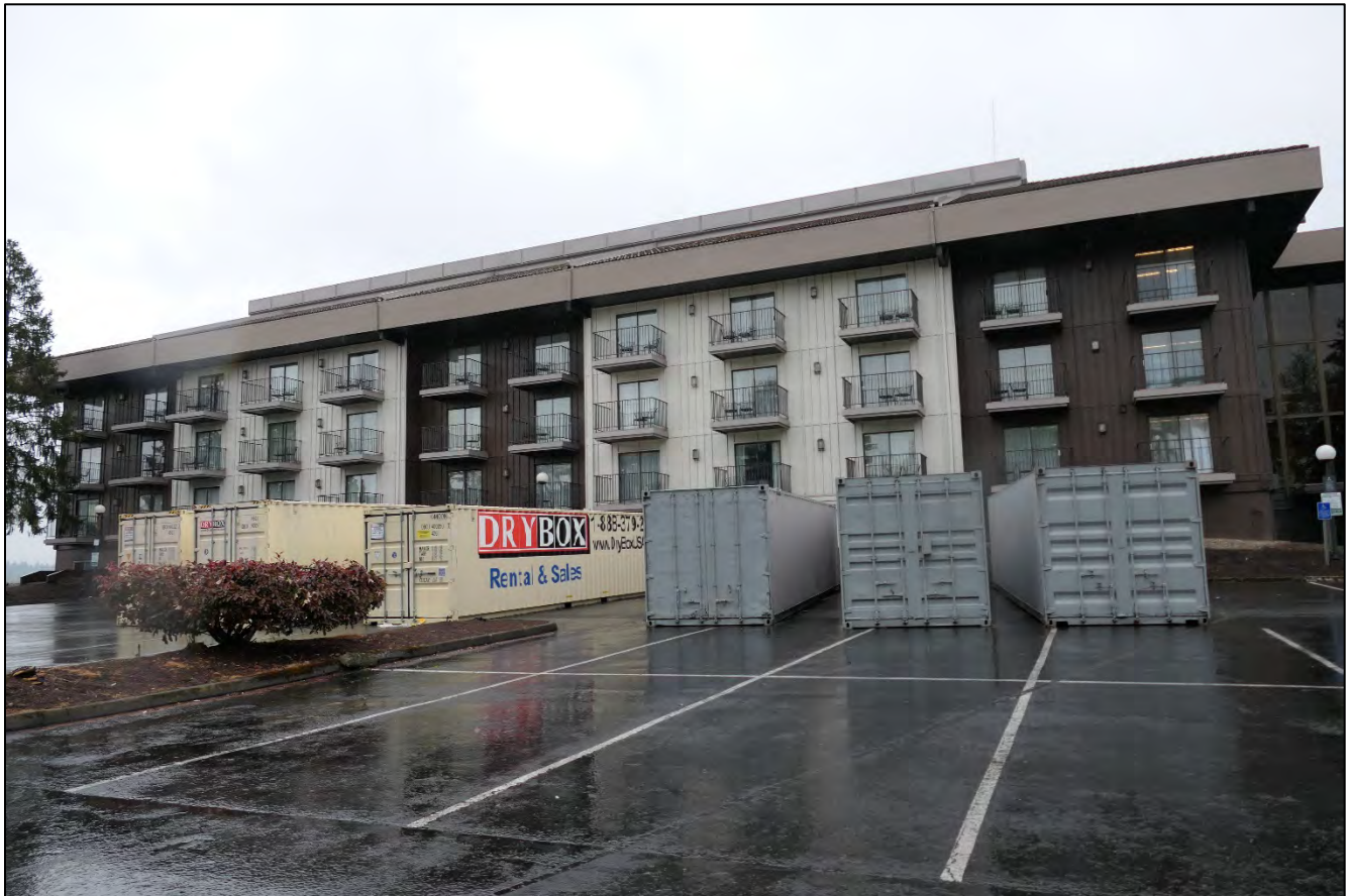
Figure 8. Overview of southwestern elevation. View facing northeast (WillametteCRA May 4, 2023).
