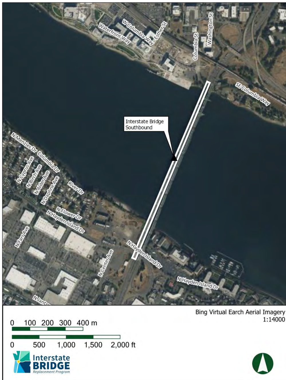
Figure 2. Aerial photograph showing location of Southbound Interstate 5 Columbia River Bridge.
