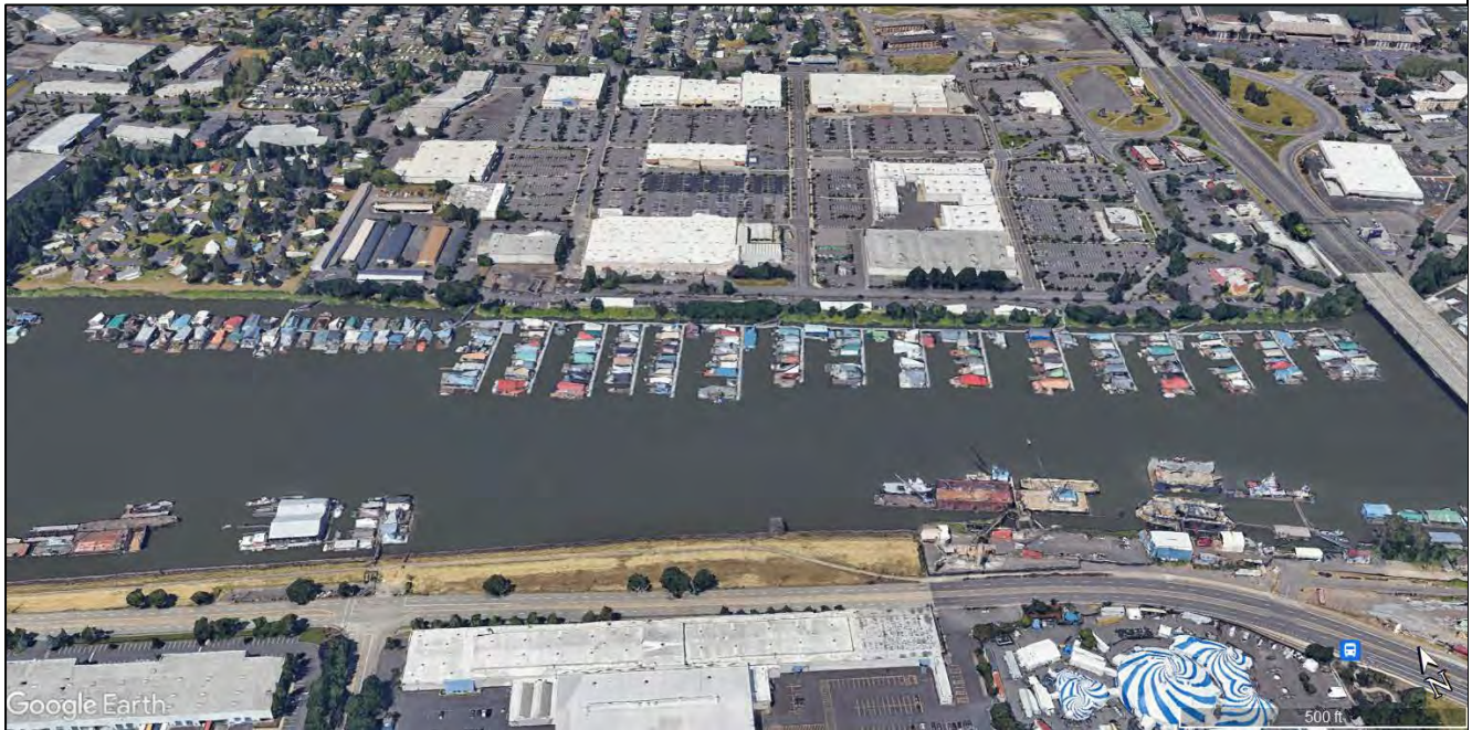
Figure 1. View of Jantzen Beach Moorage, facing northeast (Google Earth Pro 2023).
