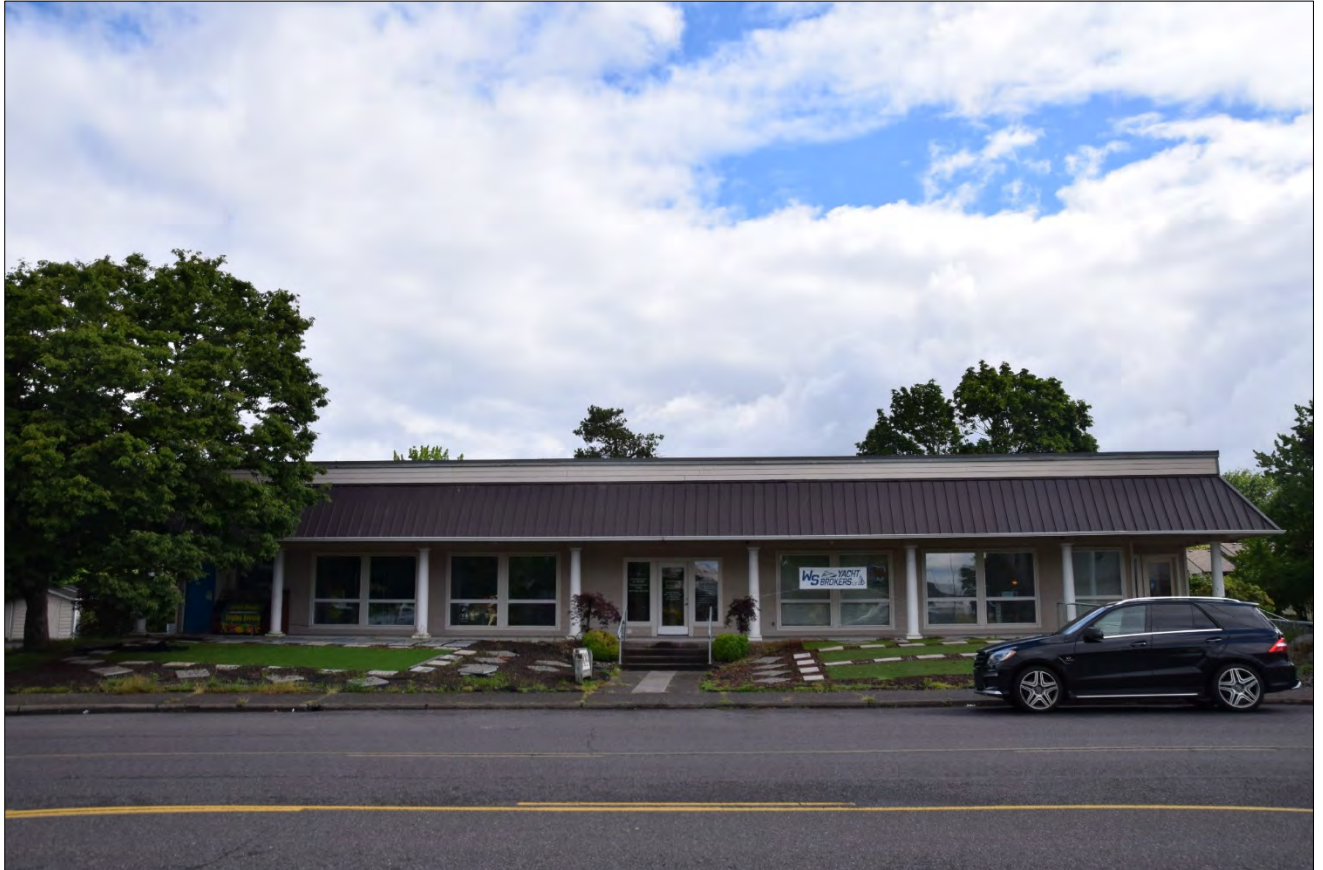
Figure 1. Hayden Island Inc. Building, view facing northeast (WillametteCRA, June 14, 2022).
