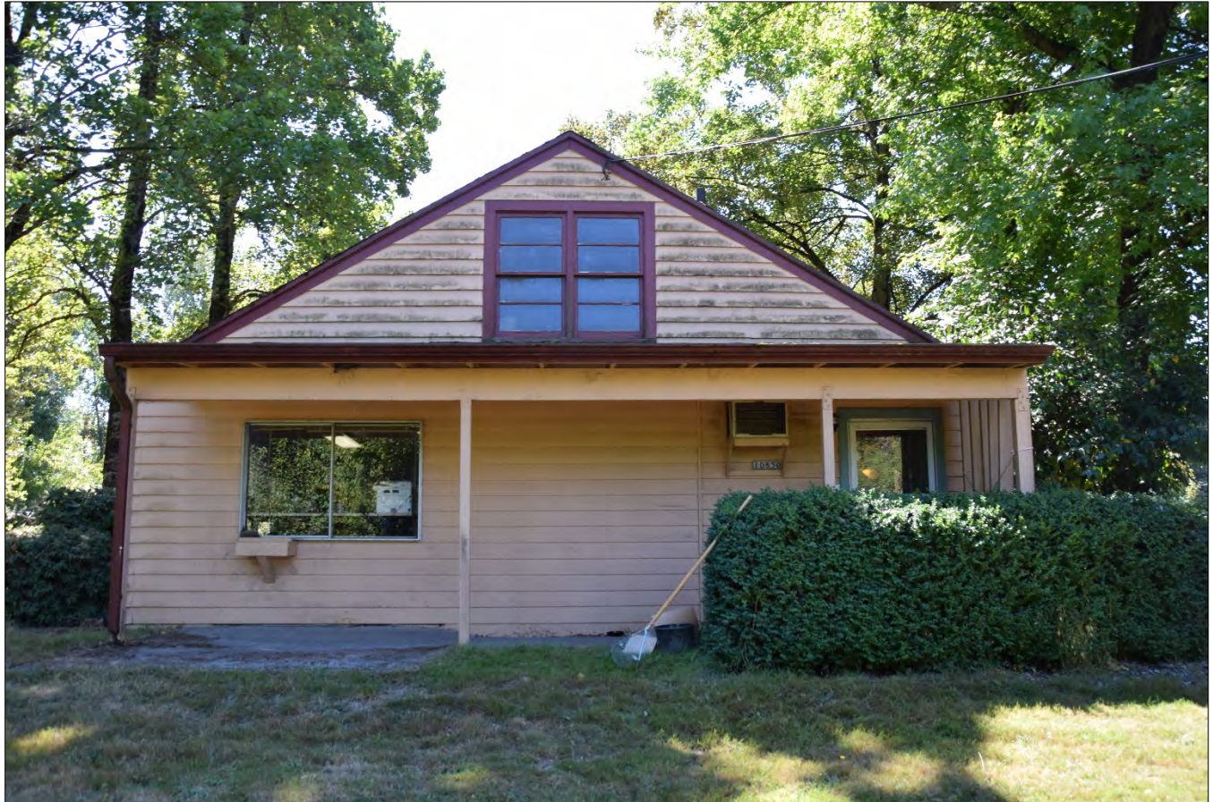
Figure 9. North elevation including secondary entrance. View facing south (WillametteCRA September 6, 2022).
