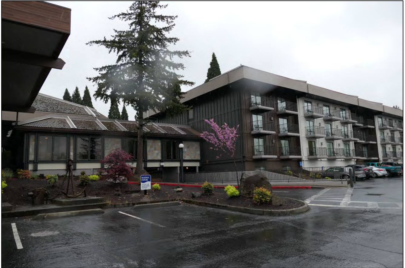
Figure 6. Overview of southwestern elevation of banquet hall and guest building. View facing northwest (WillametteCRA May 4, 2023).
