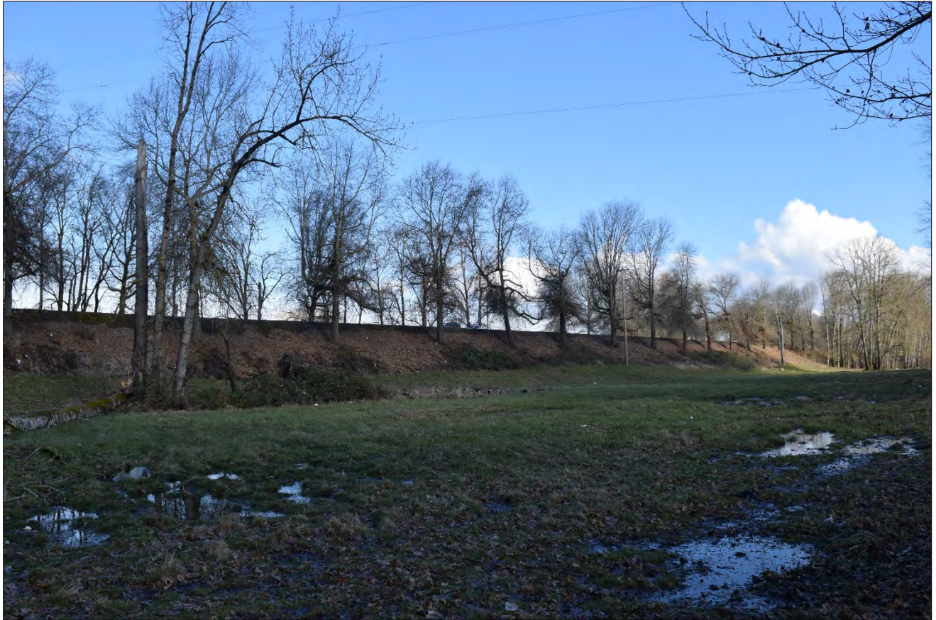
Figure 15. View of the Union Avenue/MLK Jr. Boulevard Cross Levee, south side, view facing north (WillametteCRA March 8, 2023).
