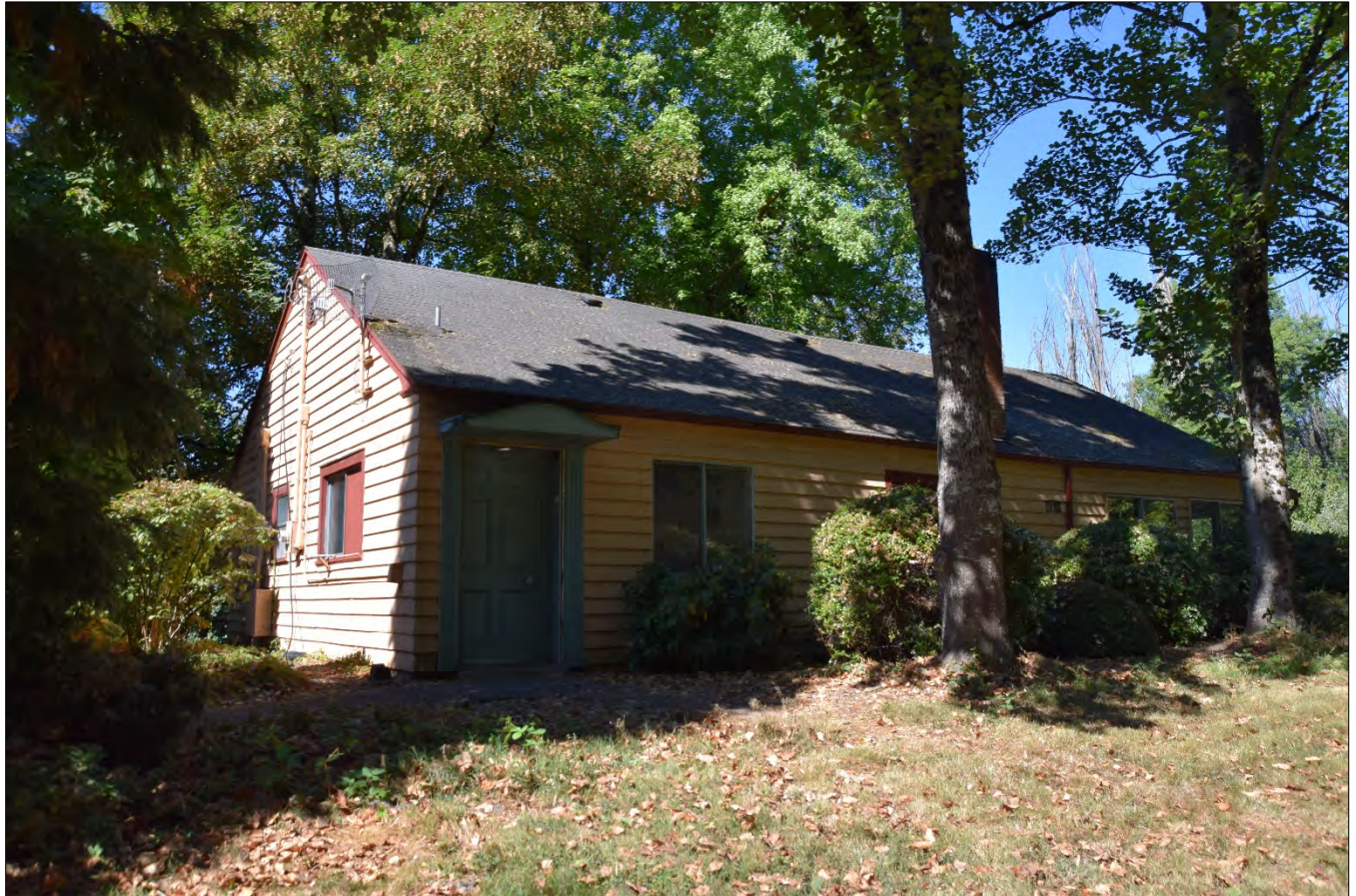
Figure 6. South and east elevations of building at 10890 North Denver Ave, including primary entrance. View facing northwest (WillametteCRA September 6, 2022).
