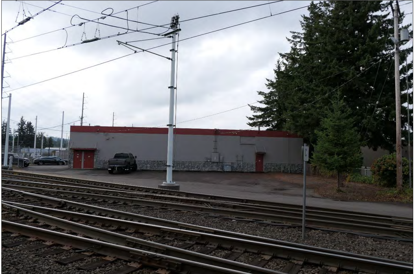
Figure 1. View of the warehouse, north elevation, view facing south (WillametteCRA September 29, 2023).
