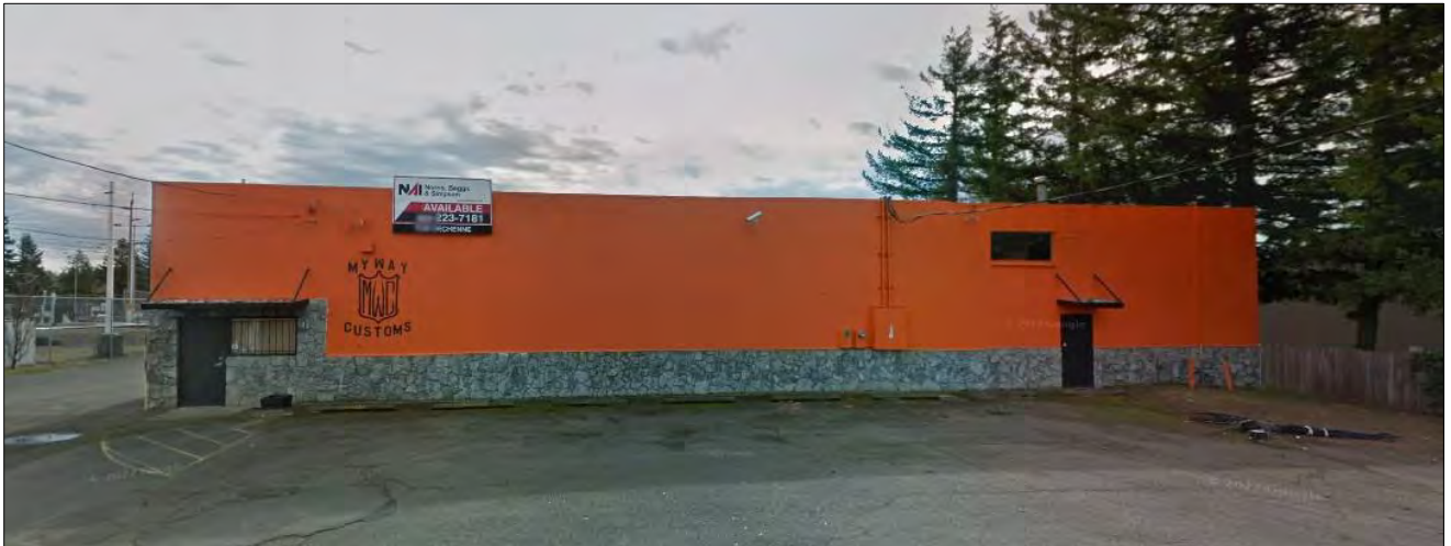
Figure 8. The warehouse, north elevation, view facing south, showing main entrance prior to alteration (Google Street View March 2016)
