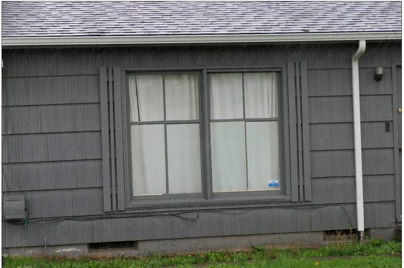
Figure 6. Residence, west elevation, detail of fixed window, facing east (WillametteCRA October 25, 2023).
