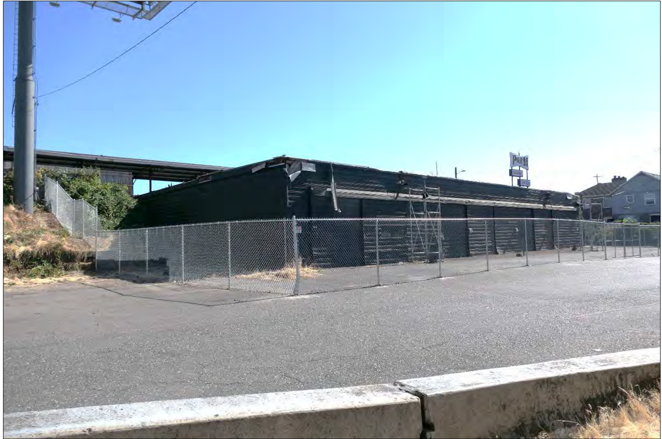
Figure 5. View of Totem Pole Marina No. 2, facing northeast (WillametteCRA August 11, 2023).
