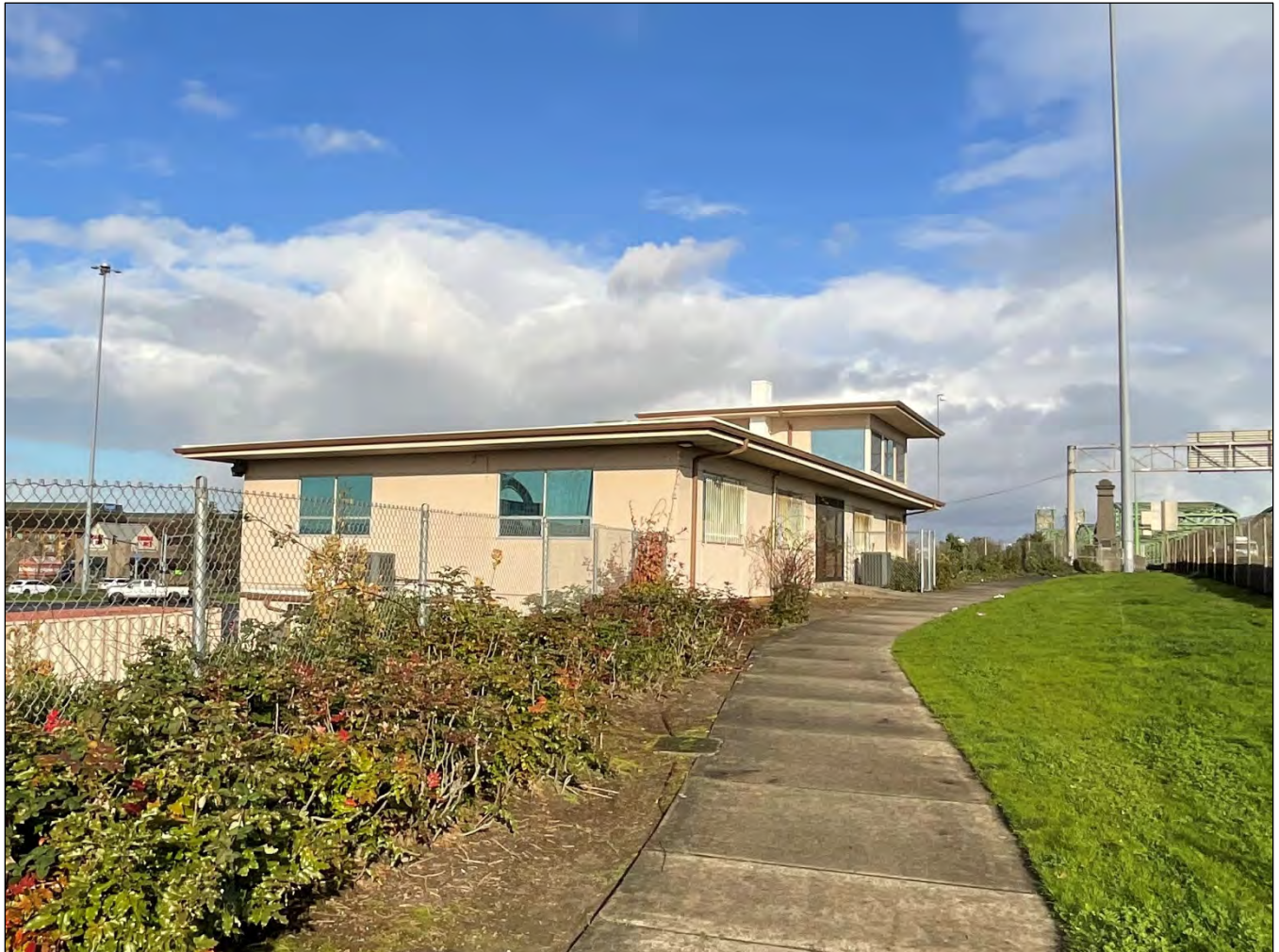
Figure 8. South and east elevations of the Toll Administration Building (ODOT Permit Center). View facing north (WillametteCRA December 8, 2021).
