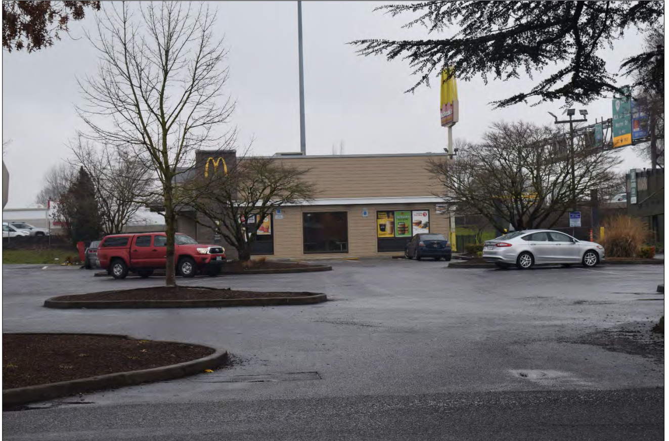
Figure 1. Jantzen Beach McDonald's, west elevation, view facing east (WillametteCRA March 8, 2023).
