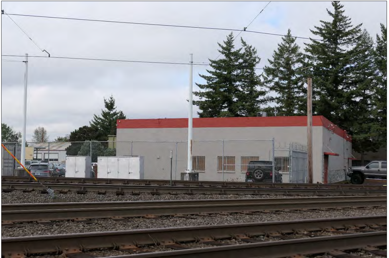
Figure 4. The warehouse, east elevation, view facing west showing fenestration (WillametteCRA September 29, 2023).
