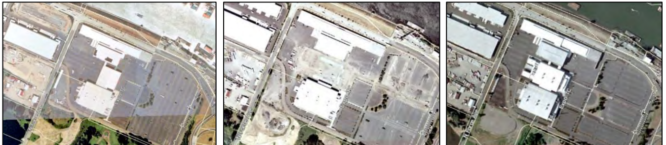
5 Figures 8–10. Aerial images of the center from summer 1999, 2000, and 2001 documenting the removal and replacement of Hall D (PortlandMaps 2023).
