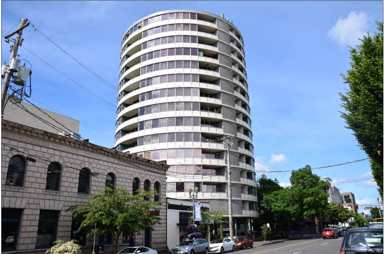
Figure 1. View of Smith Tower from the east (WillametteCRA June 08, 2022).
