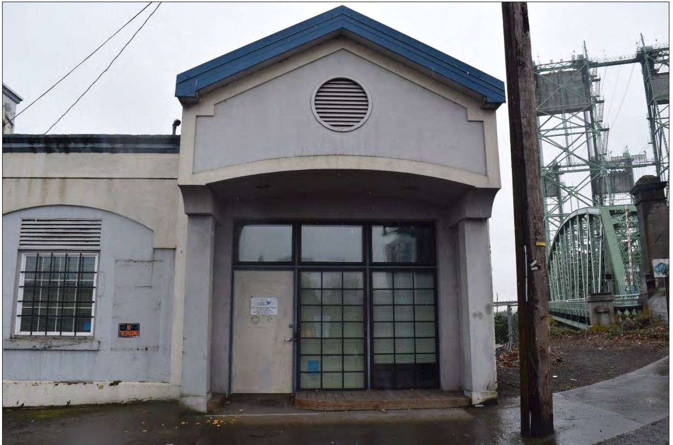
Figure 13. Closeup view of 100 SE Columbia Way from north (WillametteCRA March 8, 2023).
