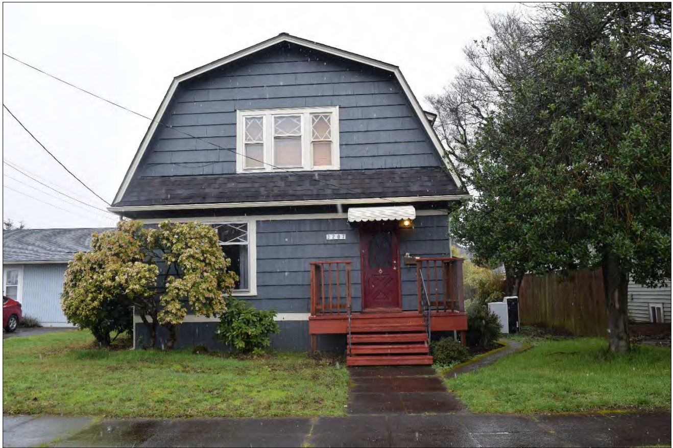
Figure 6. 3207 K Street, west elevation, view facing east (WillametteCRA, March 8, 2023).
