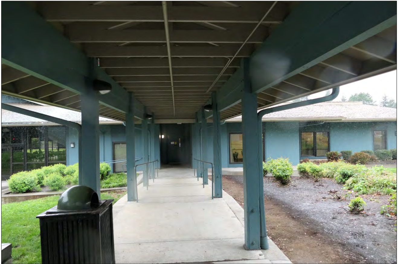
Figure 9. Luepke Center, north elevation and walkway, view facing south. (WillametteCRA, May 4, 2023).
