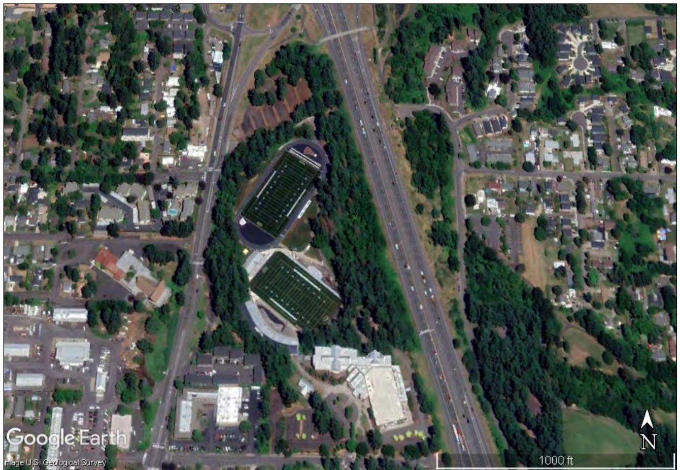
Figure 10. Kiggins Bowl with newly installed north football field and enlarged south field and pathways (Google Earth Pro July 2022).
