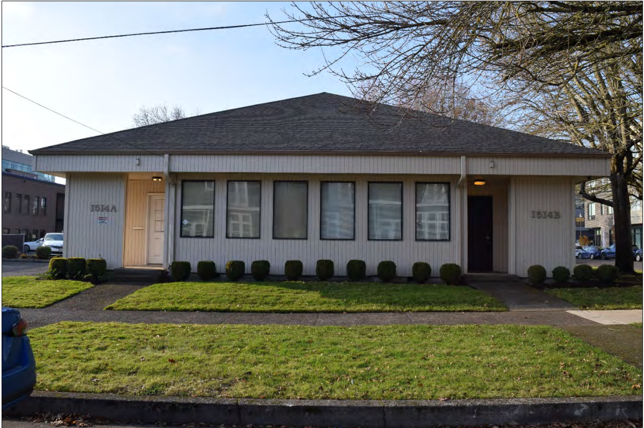
Figure 4. View of the Office Building at 1514 E Street, looking west (WillametteCRA December 14, 2022).
