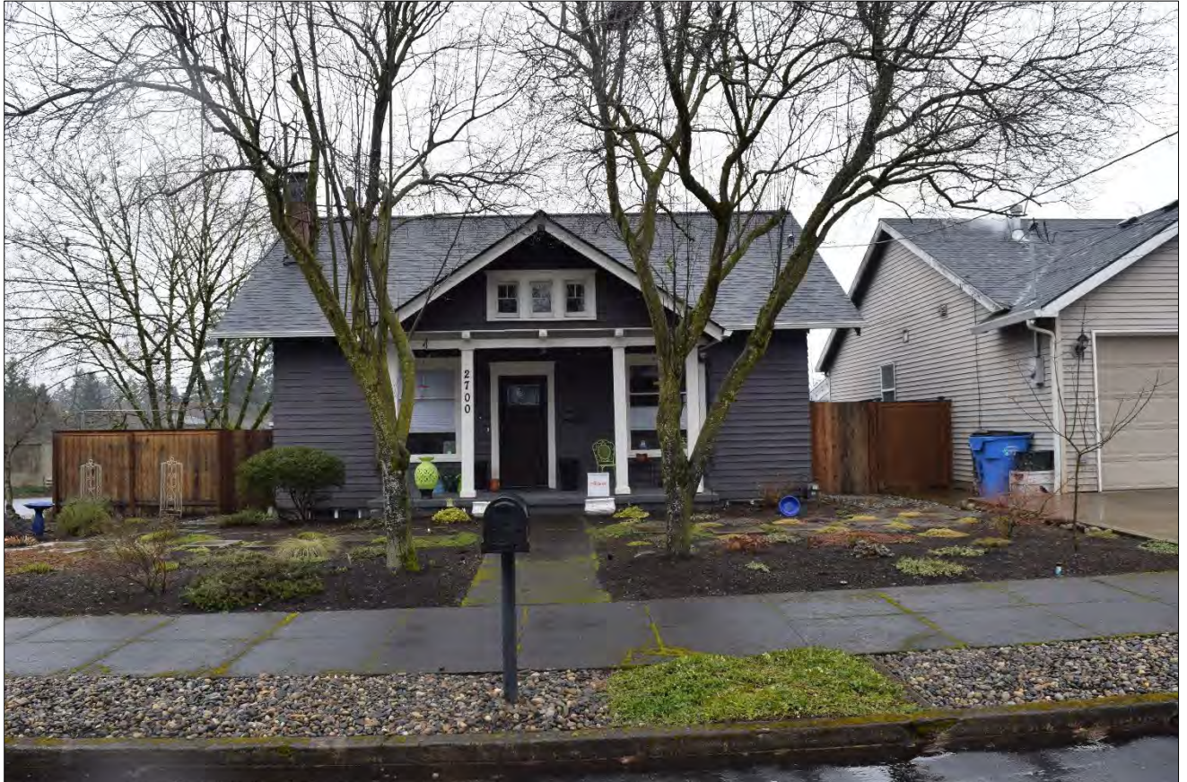
Figure 1. View of 2700 K Street, East Elevation, view facing west (WillametteCRA March 8, 2023).
