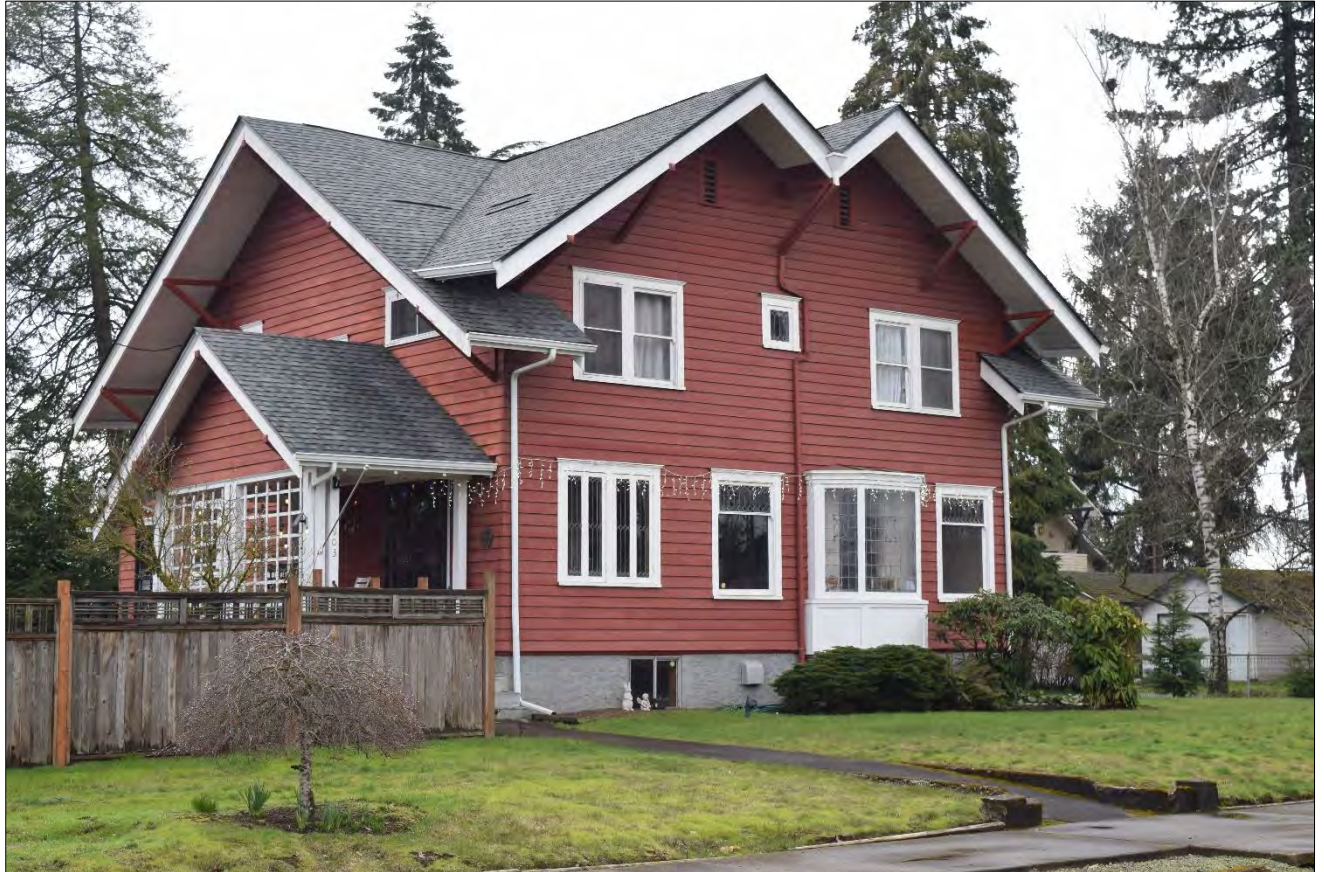
Figure 1. Hall House, north elevation, view facing southwest (WillametteCRA March 8, 2022).
