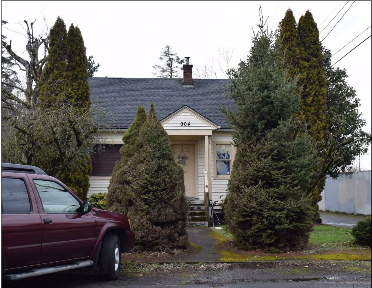
Figure 1. Peter Rosegard House, south elevation, view facing north. Building is heavily obscured by vegetation, see Figure 5 for a less obstructed image from the Clark County Assessor (WillametteCRA, March 8, 2023).
