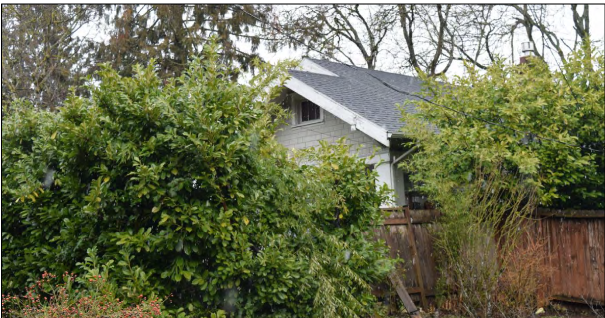
Figure 6. Hood Residence, west elevation, view facing northeast (WillametteCRA, March 8, 2023).
