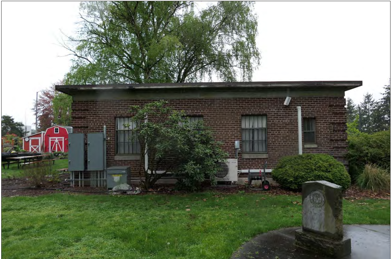
Figure 4. The Radio Transmission Building, west elevation, view facing east (WillametteCRA May 4, 2023).
