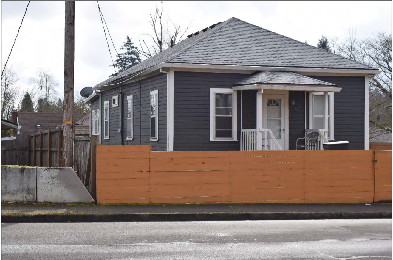
Figure 4. 901 East 29th Street, east and north elevations, view facing south (WillametteCRA March 8, 2023).
