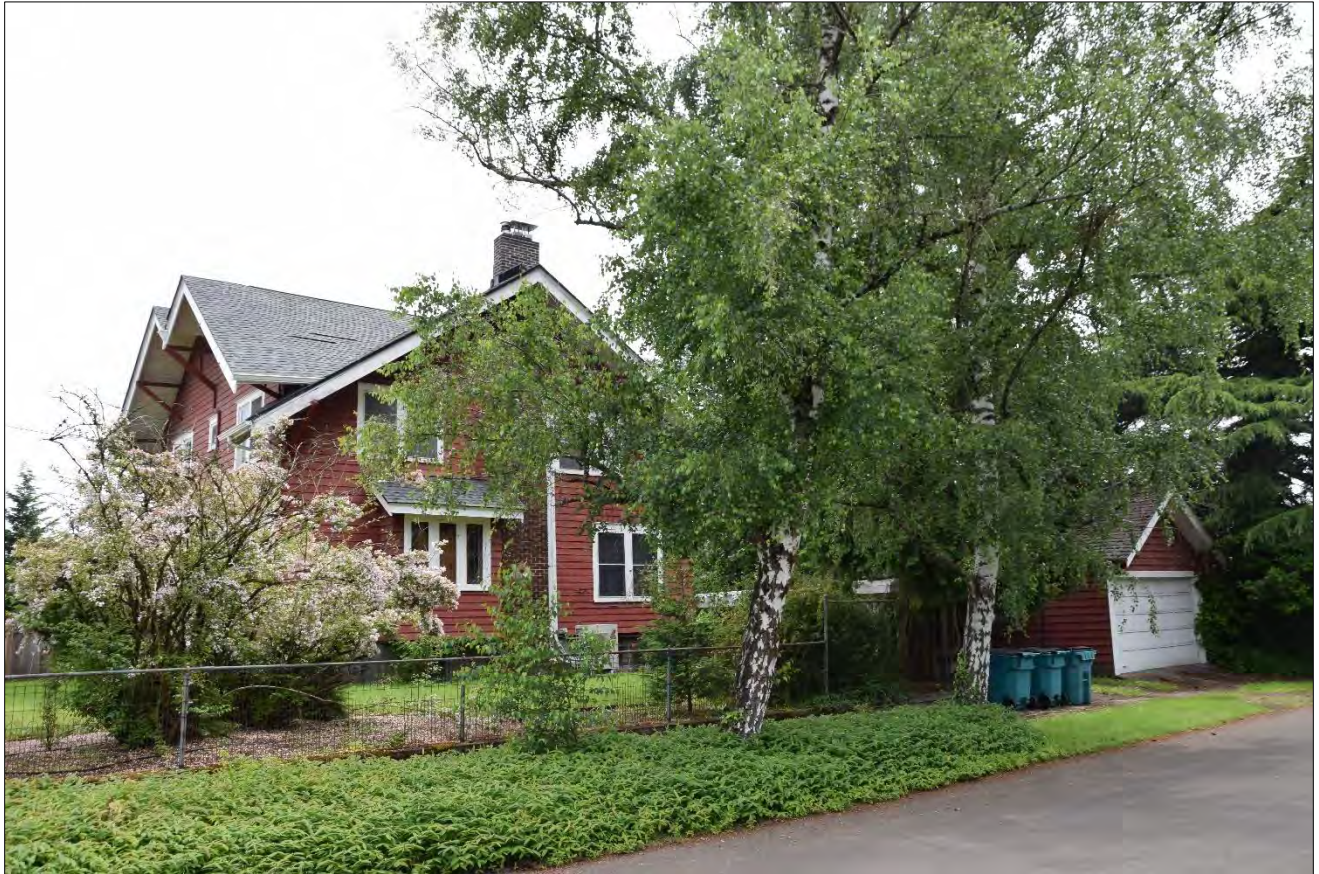
Figure 6. Hall House, north and west elevations, view facing southeast (WillametteCRA June 8, 2022).
