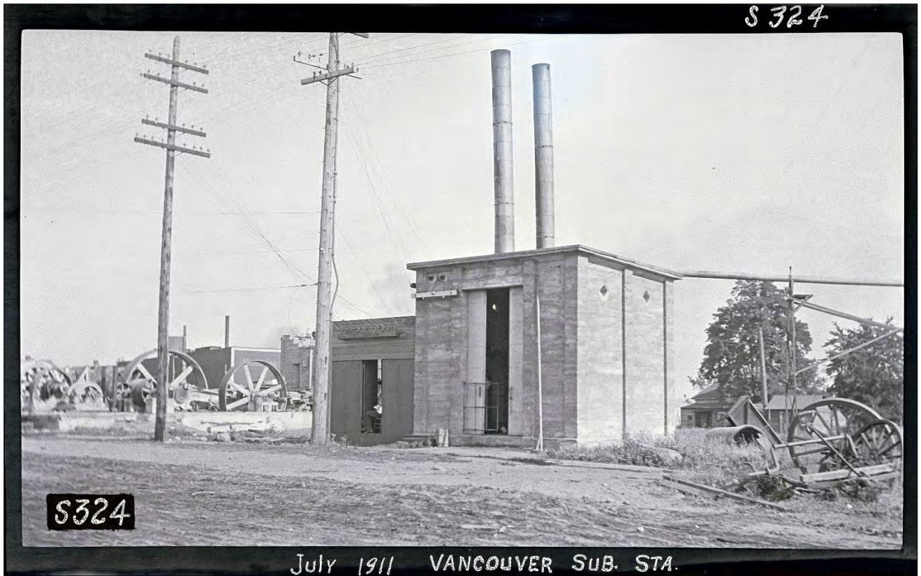
Figure 32. Portland Railway, Light and Power (PRLP) power station at Vancouver, destroyed by fire in June 1909. Only the reinforced-concrete transformer house remains standing (Oregon Historical Society).
