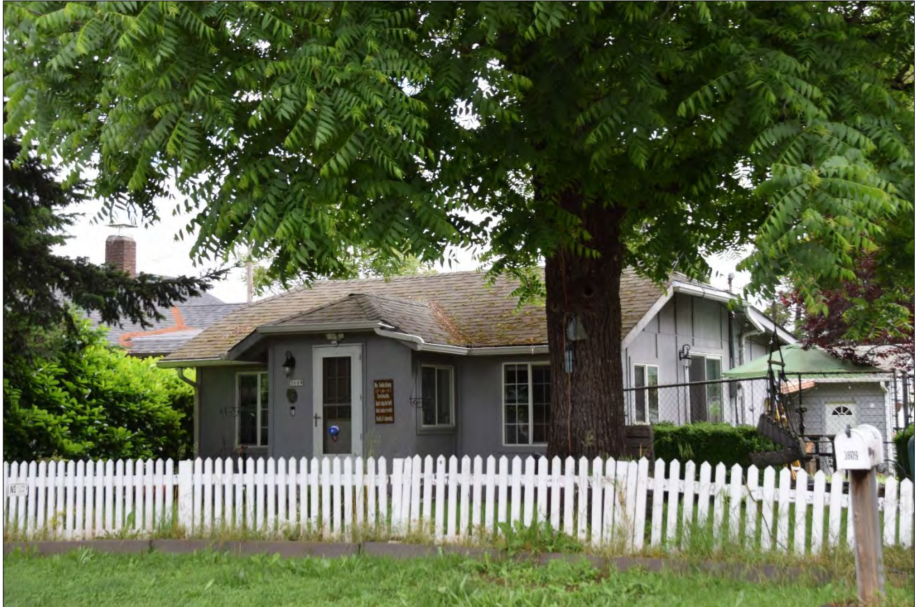
Figure 1. 3609 I Street, west elevation, view facing east (WillametteCRA June 14, 2022).
