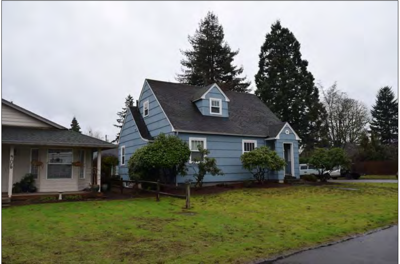
Figure 6. Nested gable on the east elevation. View facing southwest (WillametteCRA January 16, 2023).
