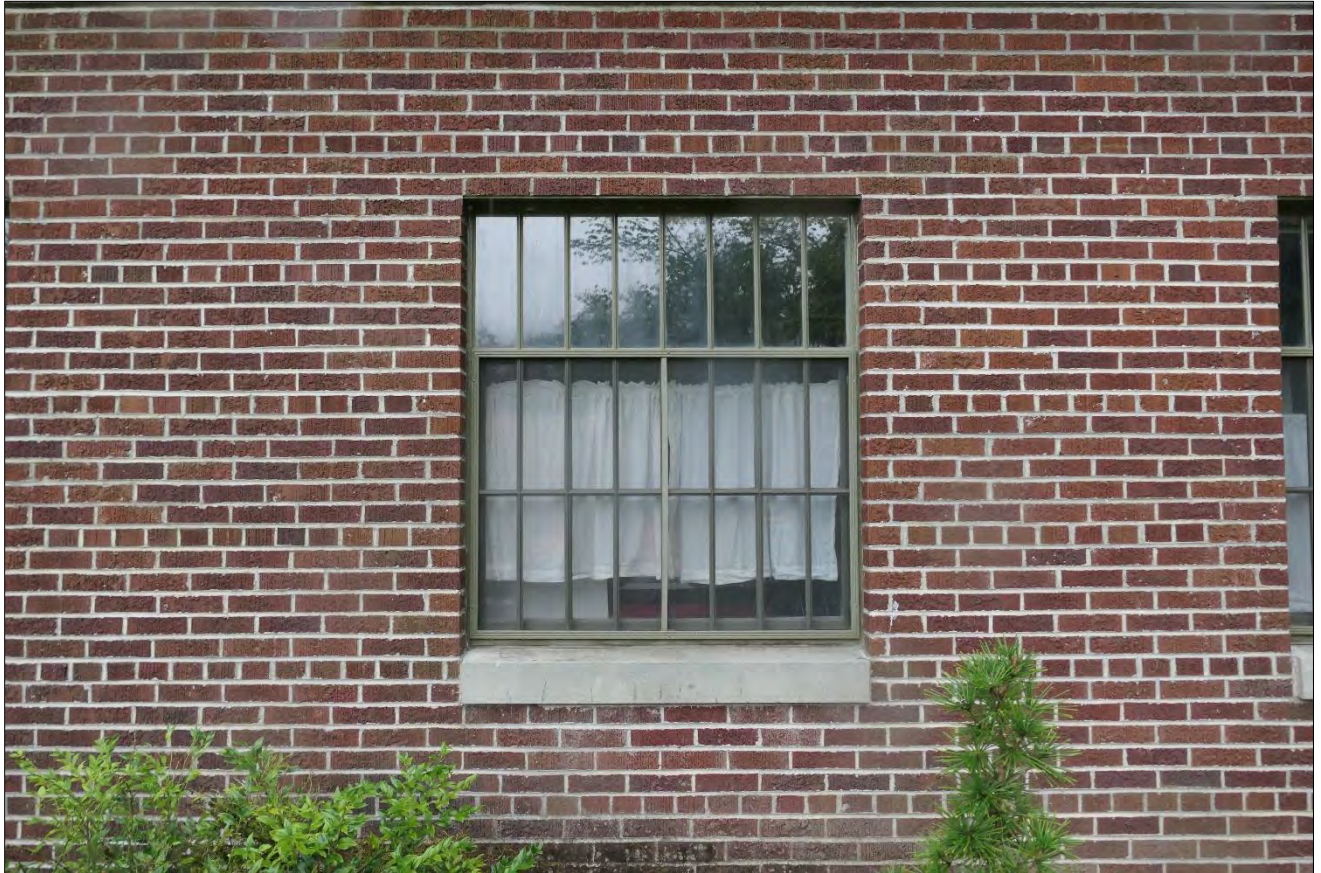
Figure 10. The Radio Transmission Building, north elevation, view facing south. Detail of window (WillametteCRA May 4, 2023).
