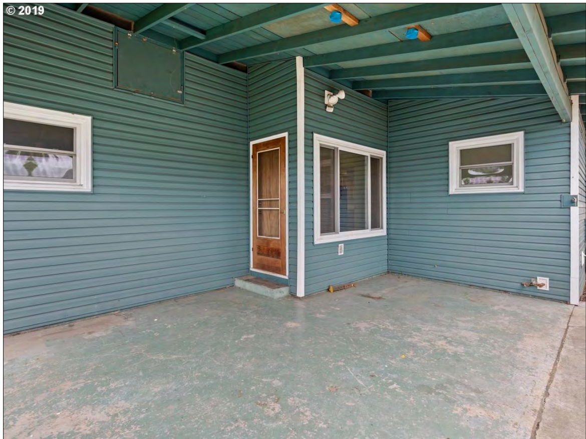
Figure 6. The Oddie Larson House, rear entrance, view facing southwest (Zillow, 2019).
