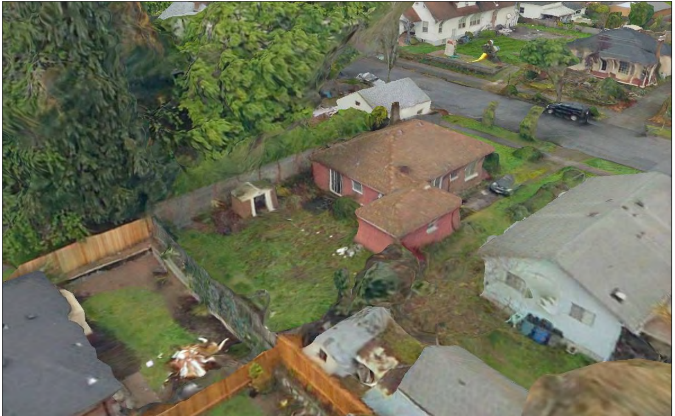
Figure 10. 809 East 29th Street, south and east elevations, oblique aerial view facing northwest (IBR/Bentley Systems May 26, 2022).
