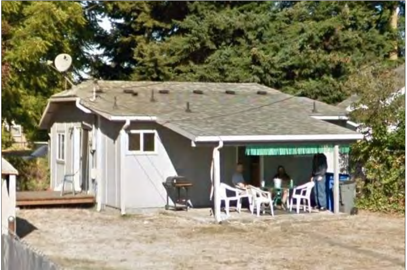
Figure 11. 3609 I Street, south and east elevations of main building, view facing northwest (Google Street View, 2014).
