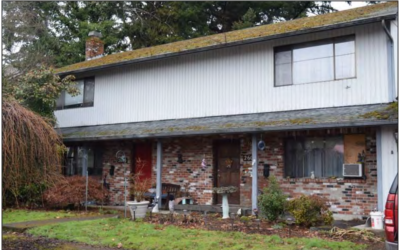
Figure 4. 2601 K Street, front porch, view facing east (WillametteCRA March 8, 2023).
