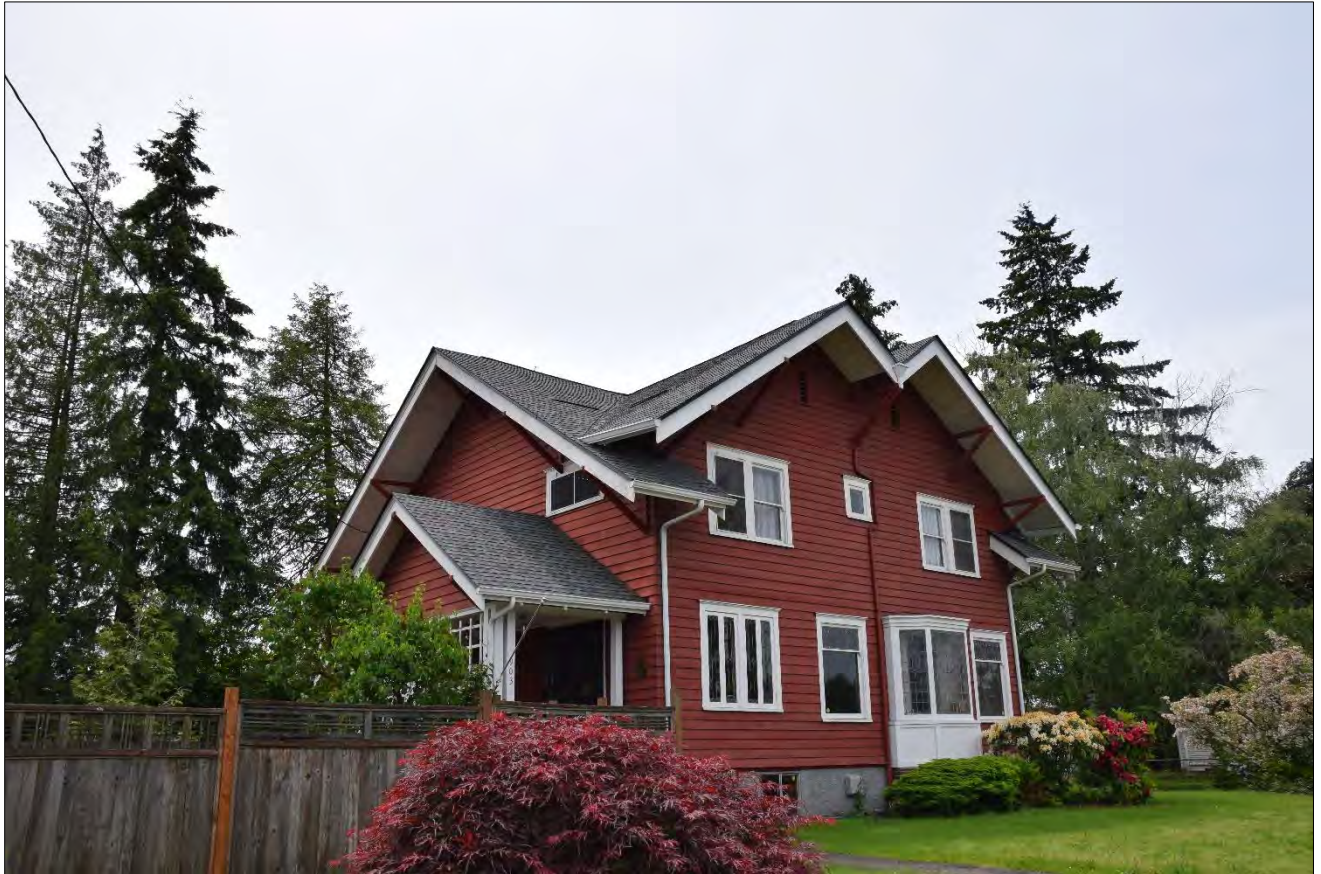
Figure 4. Hall House, east and north elevations, view facing southwest (WillametteCRA June 8, 2022).
