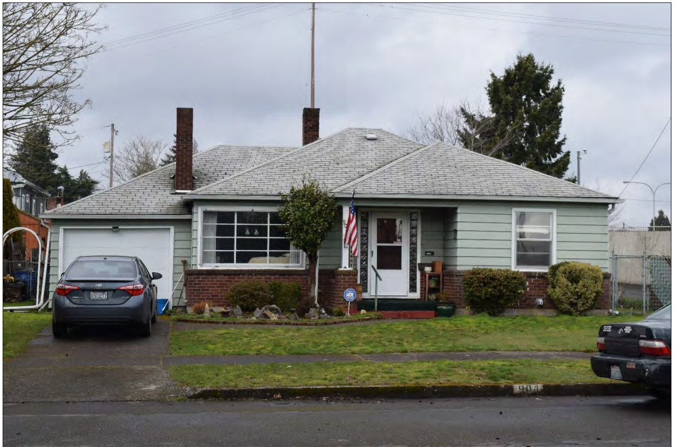
Figure 1. 904 East 28th Street, south elevation. View facing north (WillametteCRA March 8, 2023).
