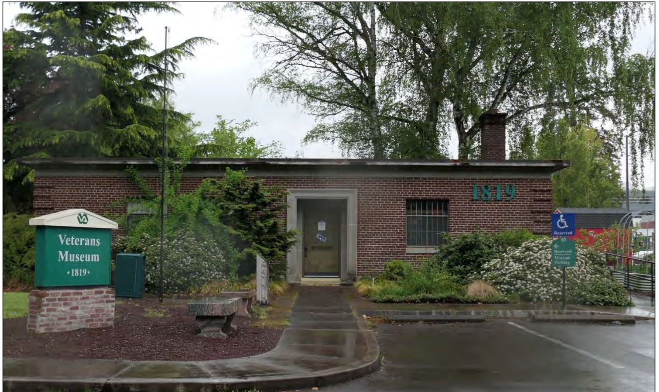
Figure 1. Radio Transmission Building, south elevation, view facing north (WillametteCRA May 4, 2023).
