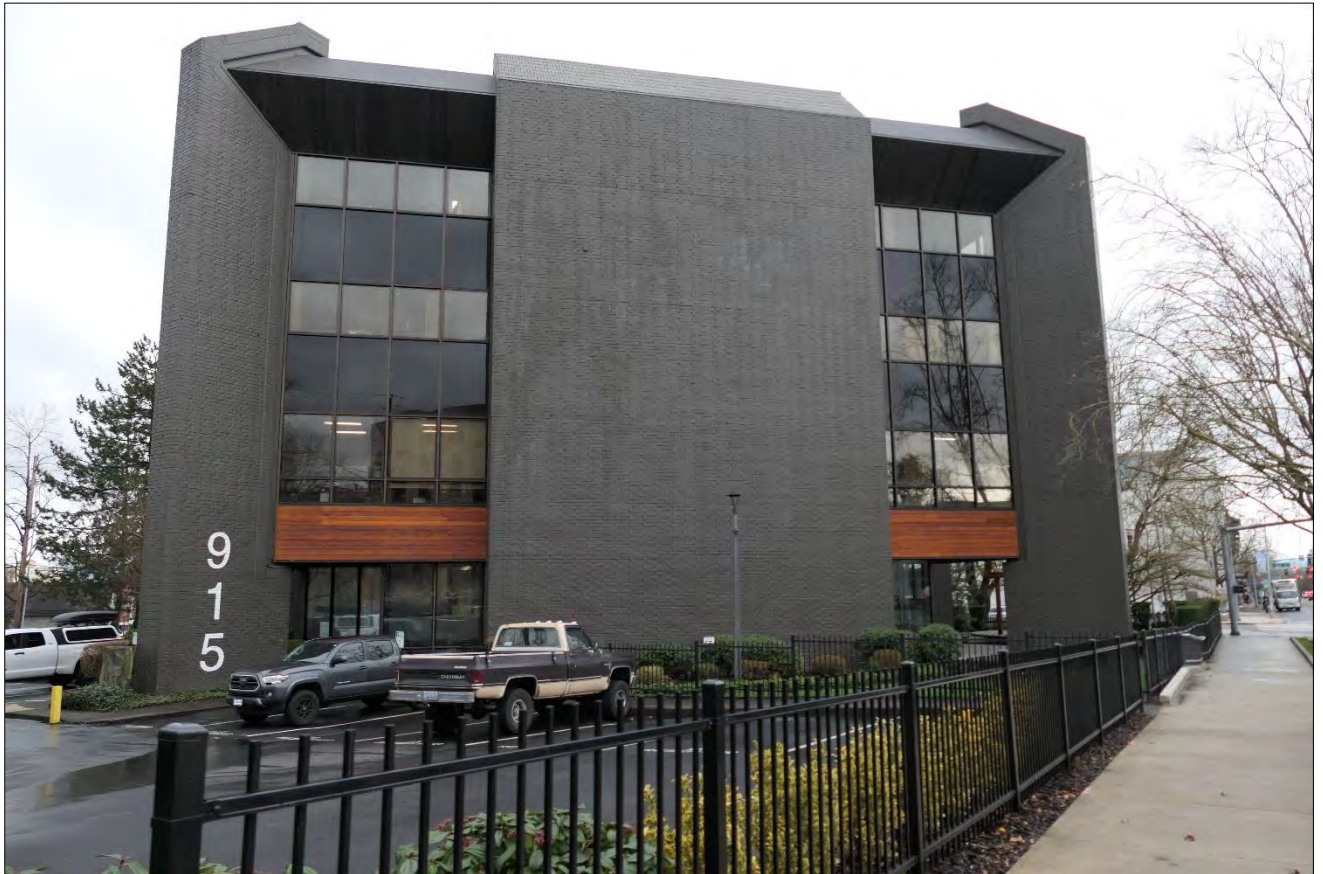
Figure 1. Northeast elevation of 915 Broadway Street, view facing southwest (WillametteCRA January 22, 2024).
