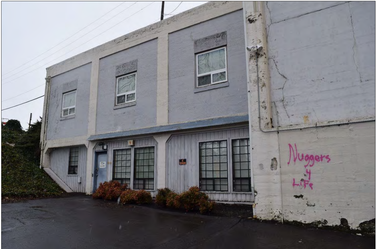
Figure 10. Closeup view of 100 SE Columbia Way from southeast (WillametteCRA March 8, 2023).
