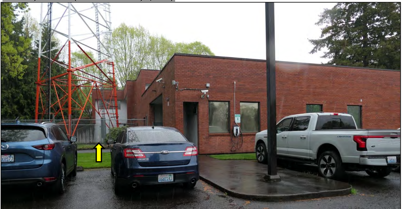
5 Figure 6. WSP District Five Headquarters, west and south elevation, view facing northeast. The arrow points to the location of a side entrance to the south elevation's west inset corner which is more visible in Figure 7 (WillametteCRA May 4, 2023).
