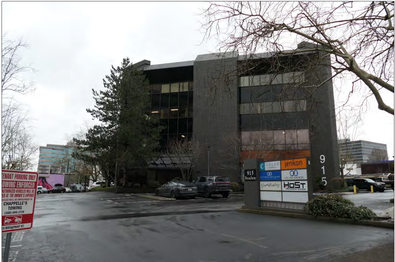
Figure 7. Southwest elevation of Pacific First Federal, looking northwest (WillametteCRA January 22, 2024).
