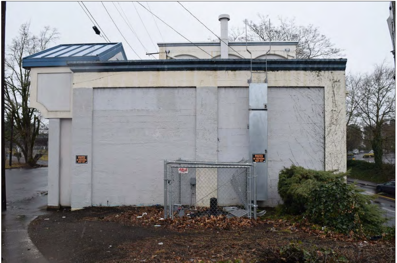
Figure 12. View of 100 SE Columbia Way from west (WillametteCRA March 8, 2023).
