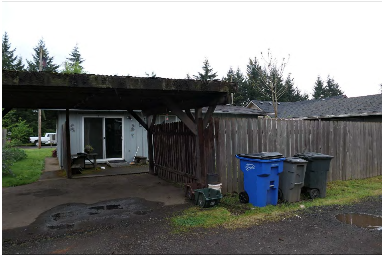
Figure 7. 3505 K Street, east elevation, view facing west (WillametteCRA May 4, 2023).
