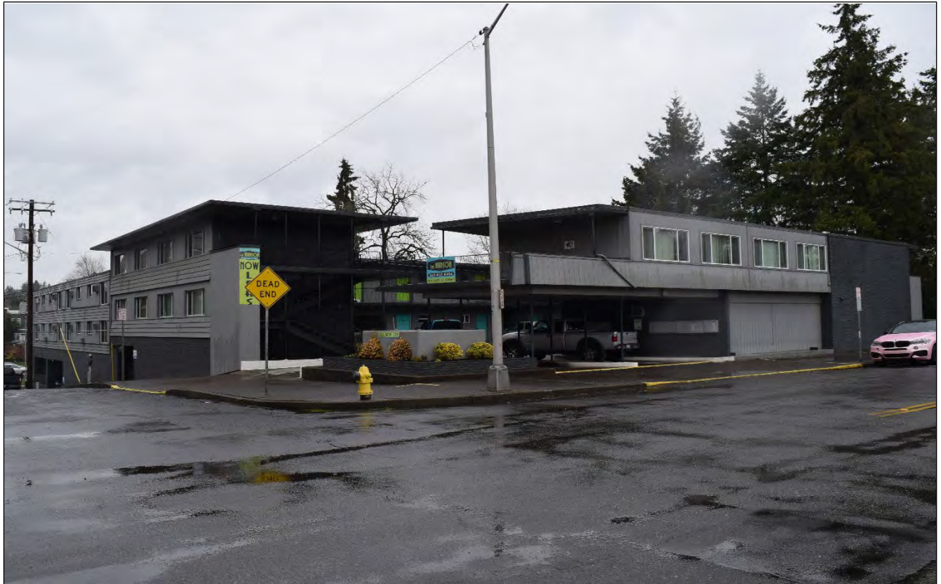
Figure 1. The Hudson (Fort Motel). View facing northeast (WillametteCRA January 16, 2023).
