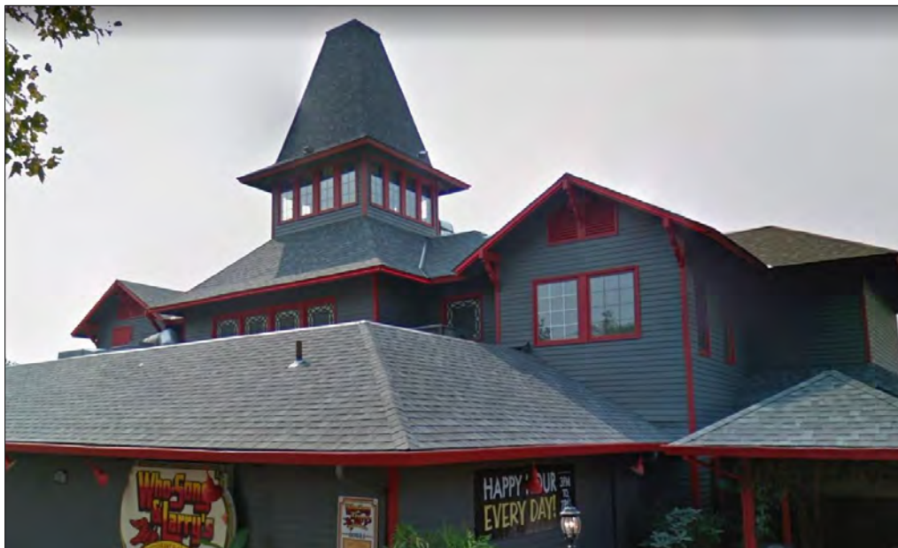
Figure 20. Who Song & Larry's Restaurant, north elevation, view facing after reroofing and repainting (Google Street View, August 2017).
