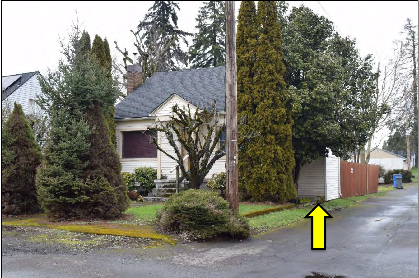
Figure 6. Peter Rosegard House, south elevation view facing northwest. Arrow points to one-story projection (WillametteCRA, March 8, 2023).
