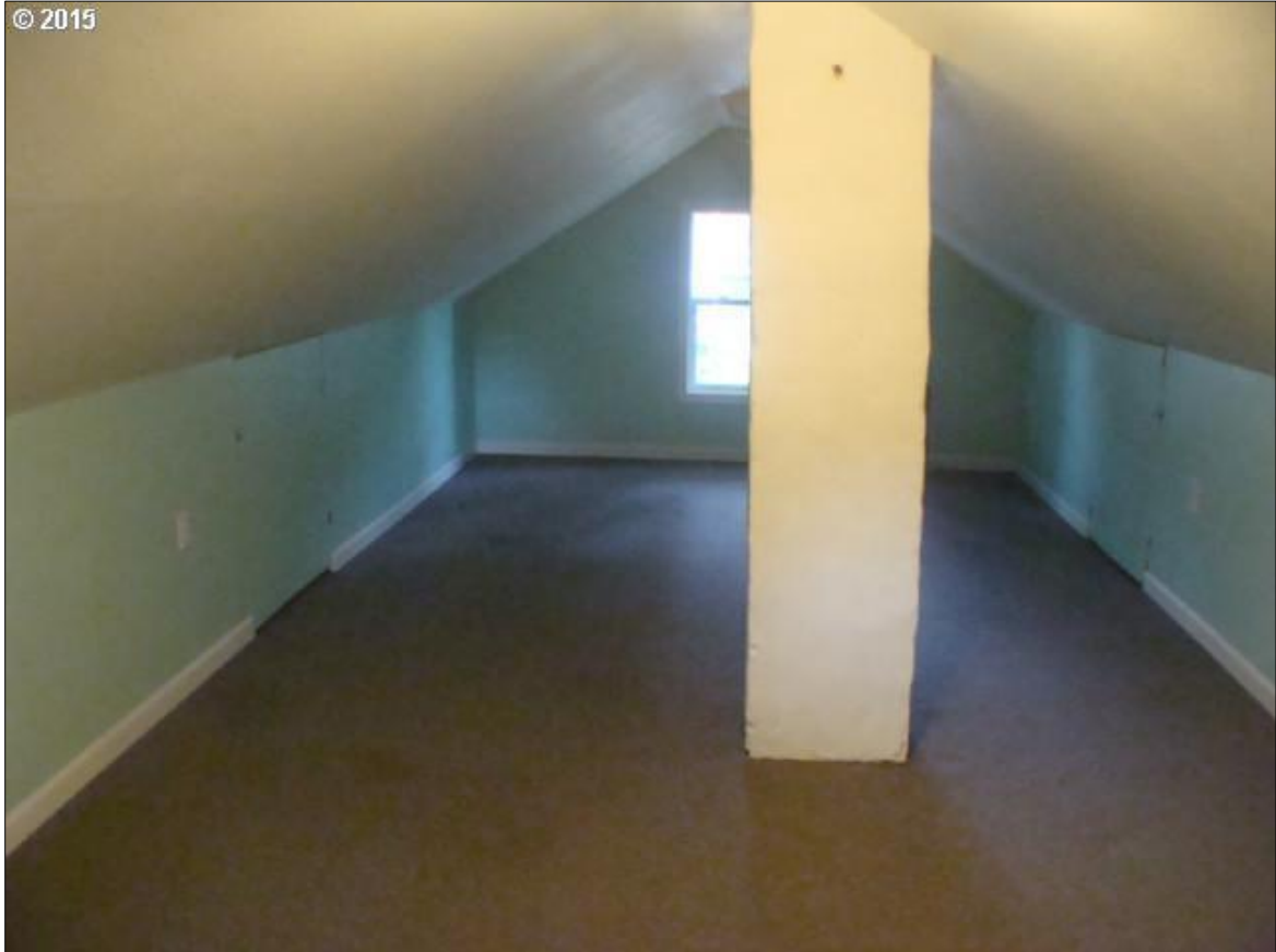
Figure 10. The Maude Erhardt House, upper room interior showing carpeted flooring (Redfin 2016).
