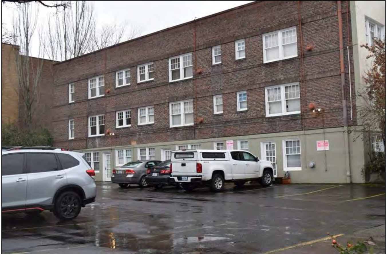
Figure 6. The west elevation of the Normandy Apartments showing the three ground-level entrances to private apartments. View facing northeast (WillametteCRA January 16, 2023).
