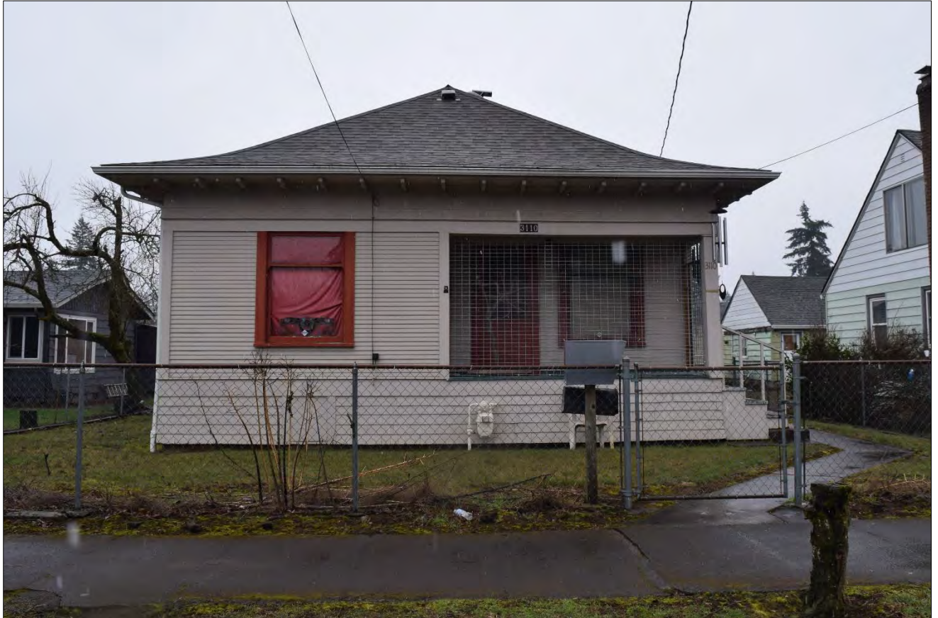
Figure 1. 3110 K Street, west elevation, view facing east (WillametteCRA March 8, 2023).
