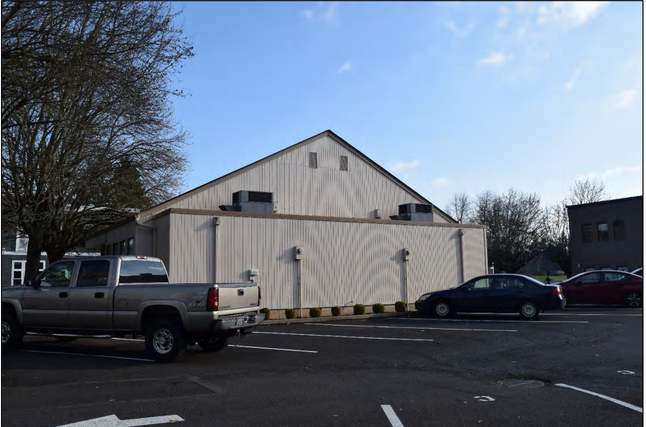
Figure 6. View of the Office Building at 1514 E Street, looking east (WillametteCRA December 14, 2022).
