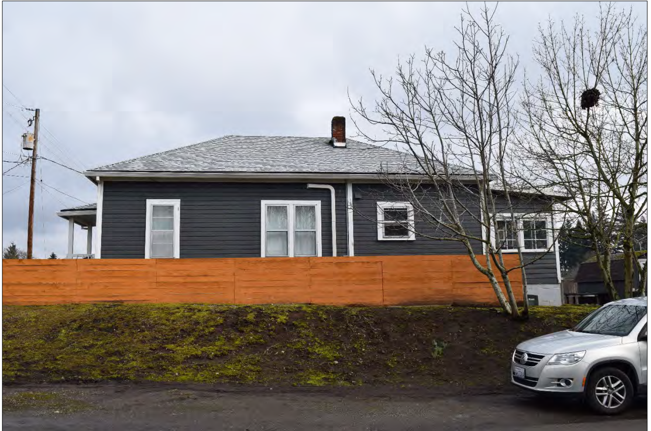
Figure 6. 901 East 29th Street, west elevations, view facing east (WillametteCRA March 8, 2023).
