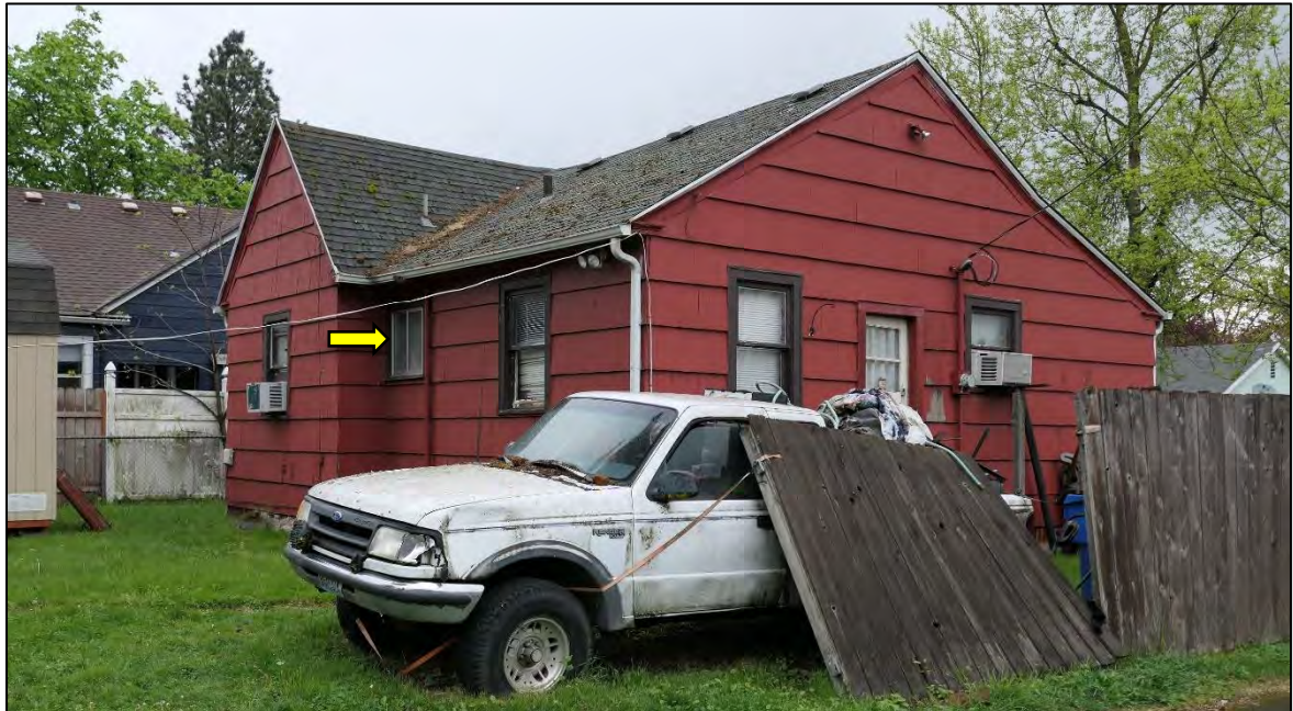
Figure 6. Walter E. and Leona M. Pearson House, south elevation (left) and east elevation (right), view facing northwest. Arrow points to replacement aluminum window (WillametteCRA, May 4, 2023).
