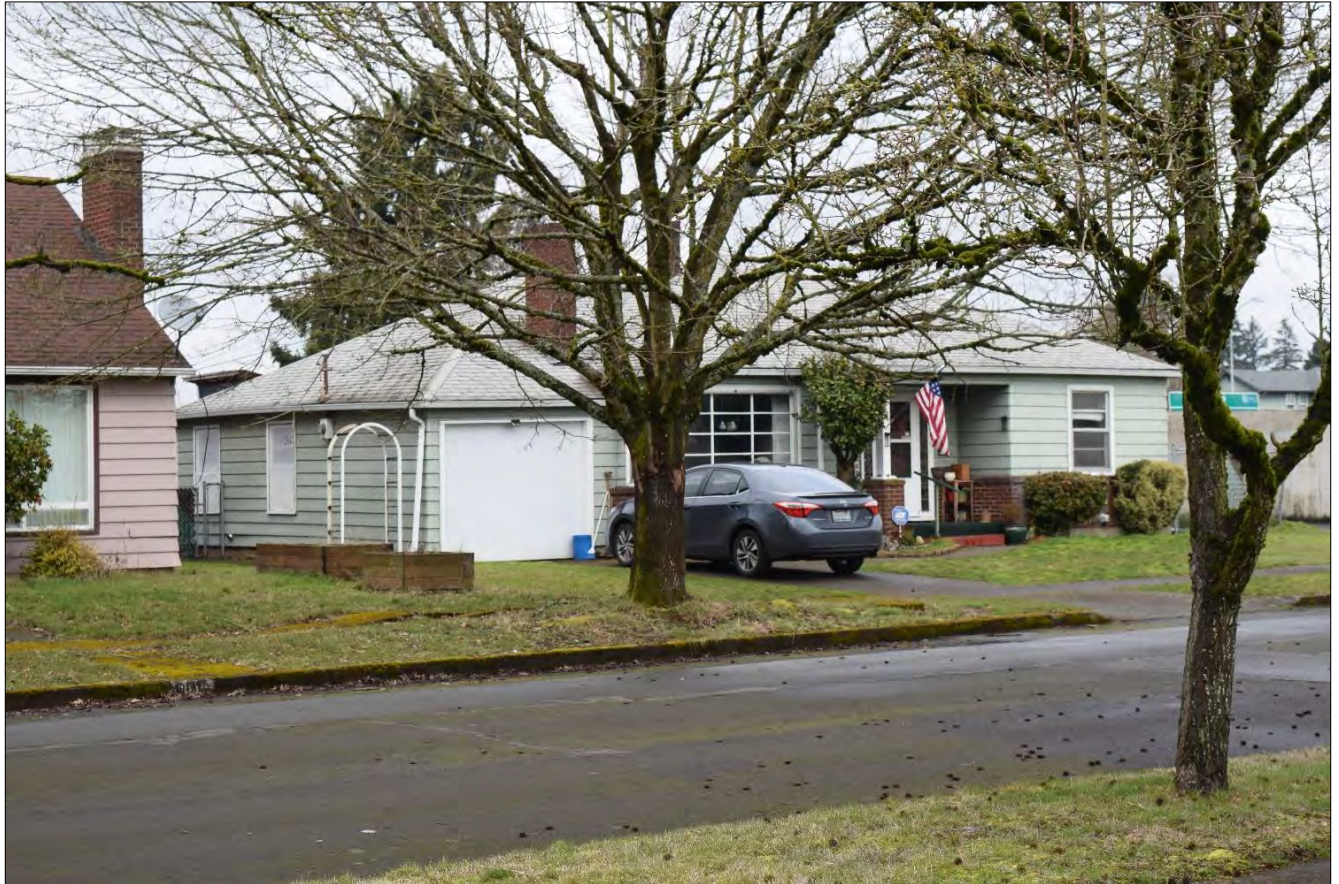
Figure 6. Deane House, south and west elevations. View facing northeast (WillametteCRA March 8, 2023).
