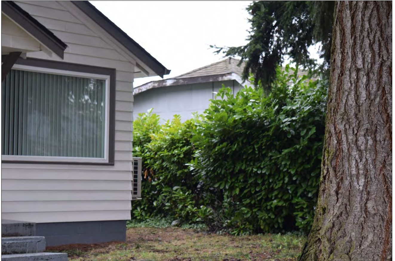
Figure 8. 3609 I Street, north elevation, view facing southeast (WillametteCRA March 8, 2023).
