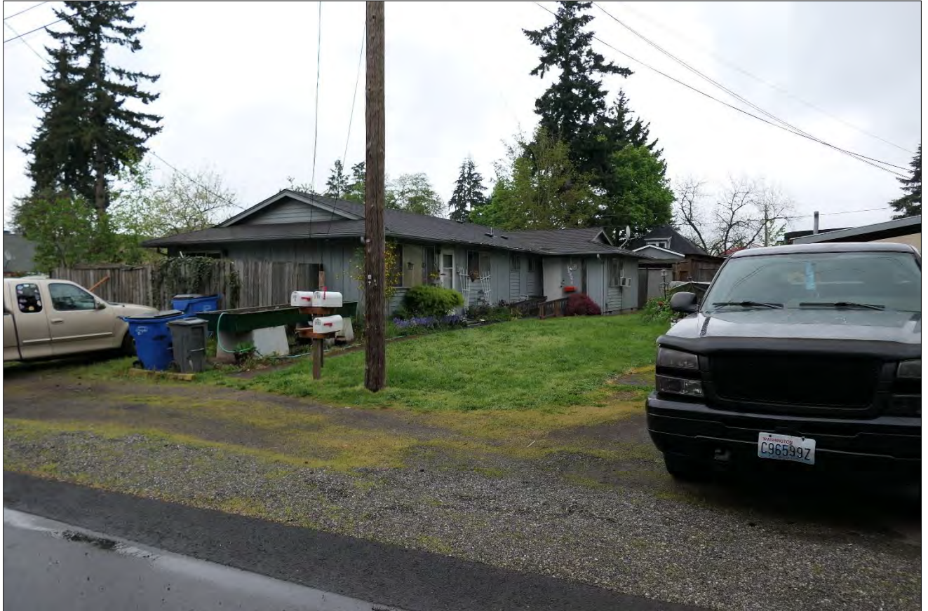
Figure 1. Ost Duplex, 3505 K St, south and west elevations, view facing northeast (WillametteCRA May 4, 2023).
