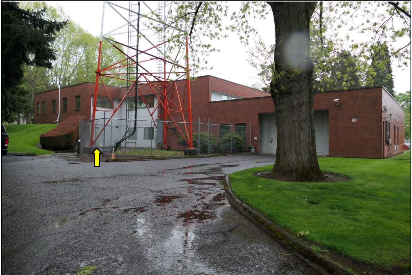
Figure 7. WSP District Five Headquarters, west elevation and west inset corner of south elevation (marked by the arrow), view facing northeast. The arrow also marks a clearer view of the side entrance noted in Figure 6 (WillametteCRA May 4, 2023).
