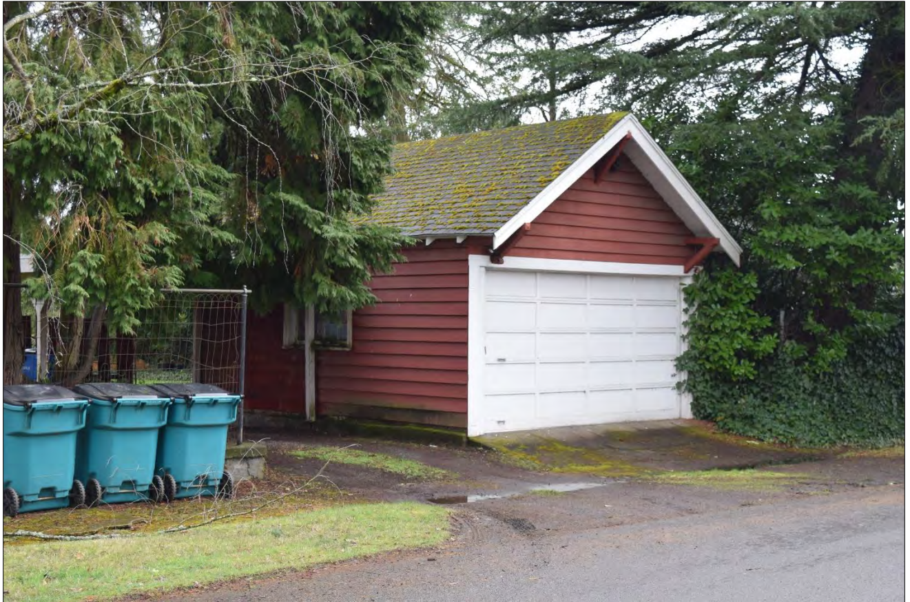
Figure 9. Hall House, detached garage, north and west elevations, view facing southeast (WillametteCRA March 8, 2022).
