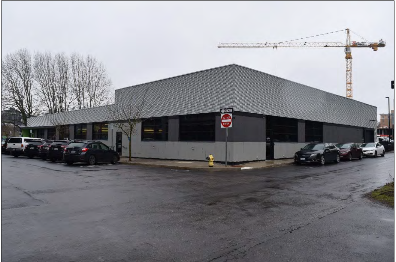
Figure 7. 210 West 3rd Street / 300 Washington Street, south and east elevations, view facing northwest (WillametteCRA March 8, 2023).
