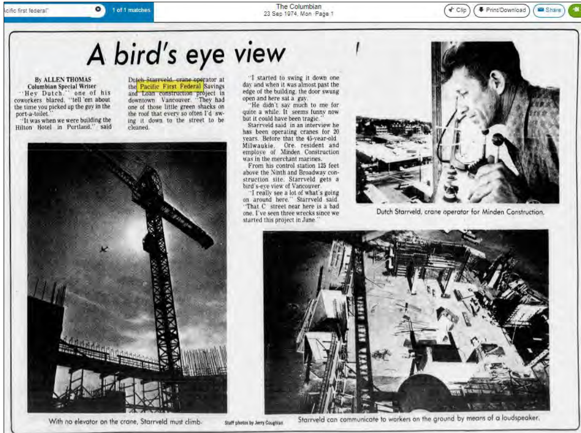
Figure 10. Views of Pacific First Federal under construction ( The Columbian [Vancouver, WA], September 23, 1974, 1).
