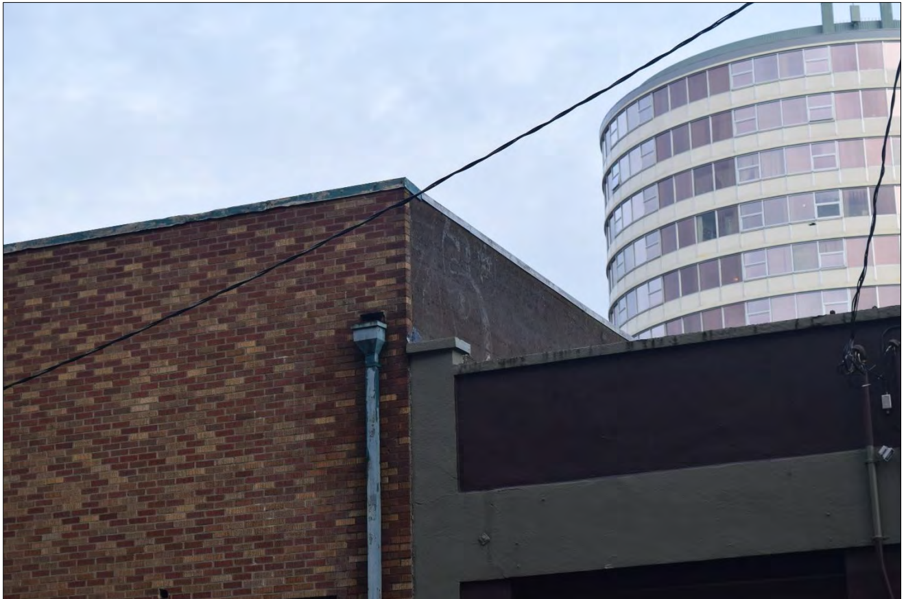
Figure 4. Southwestern corner of Fendrich's Furniture Store, view facing northeast, including brick and poured concrete elements (WillametteCRA January 13, 2023).
