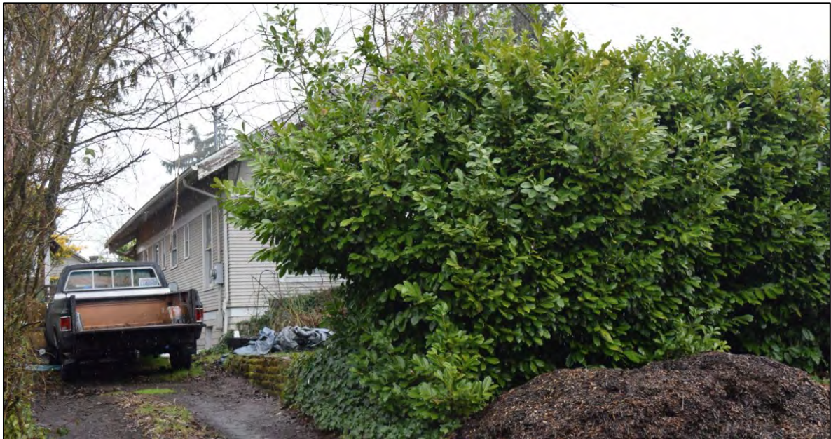
Figure 5. Hood Residence, north (left) and west (right) elevations, view facing southeast (WillametteCRA, March 8, 2023).
