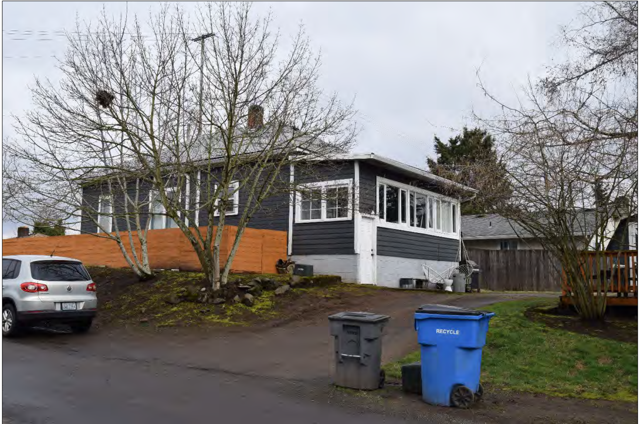
Figure 7. 901 East 29th Street, west and south elevations, view facing northeast (WillametteCRA March 8, 2023).
