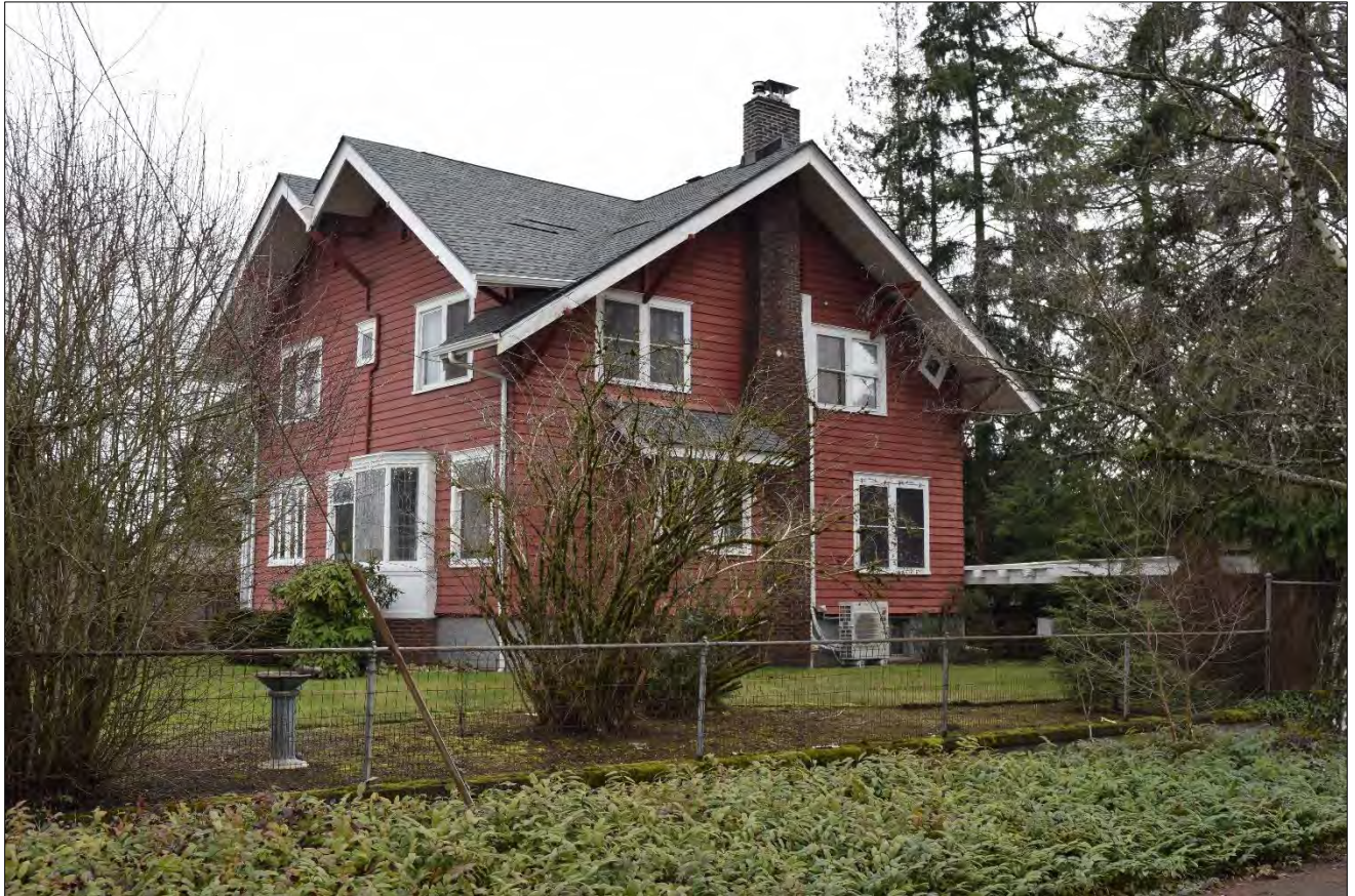
Figure 7. Hall House, north and west elevations, view facing southeast (WillametteCRA March 8, 2022).
