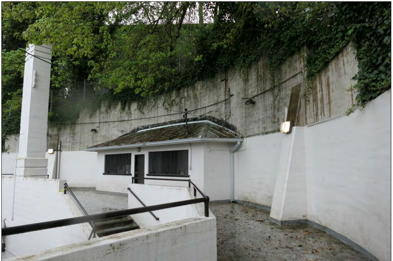
Figure 19. Kiggins Bowl stadium, upper entrance to rear stairwell. View facing south (WillametteCRA May 6, 2023).
