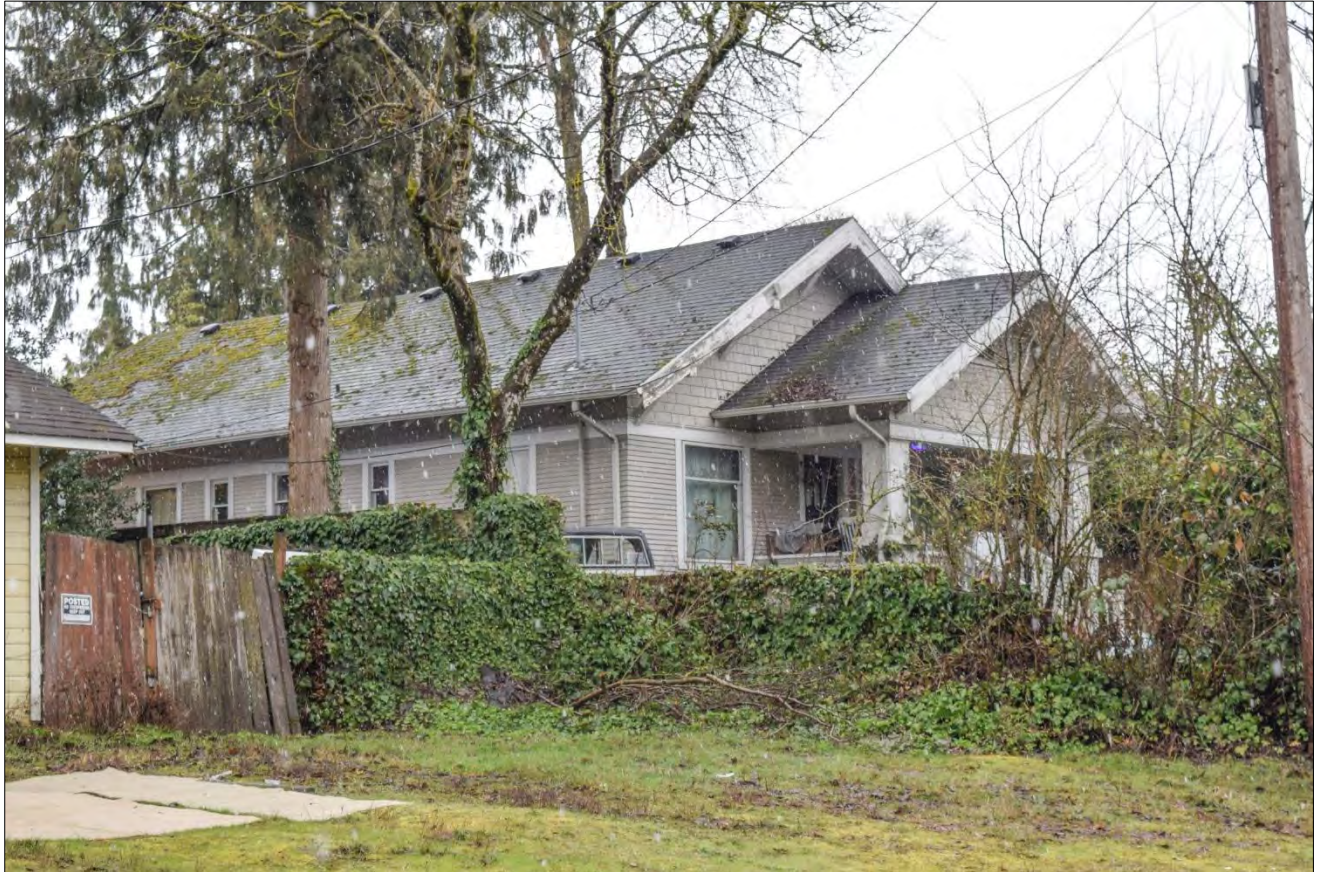
Figure 1. 3405 K Street, north and west elevations, view facing southeast (WillametteCRA, March 8, 2023).
