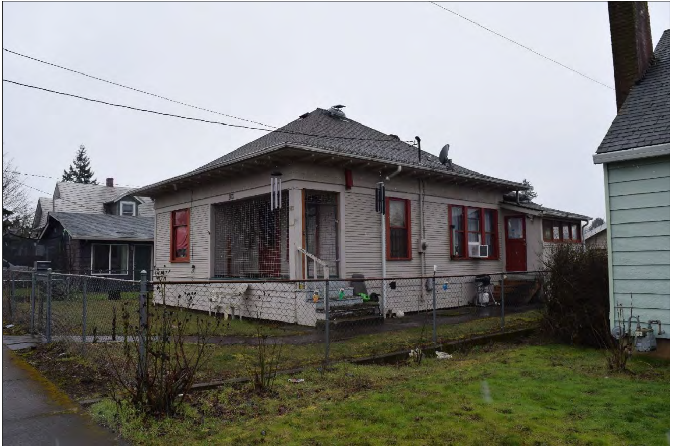
Figure 4. The Jennie Camets House, 3110 K Street, east and north elevations, view facing southwest. Note the addition of the enclosed entry at the northwest corner of the building ( WillametteCRA March 8, 2023 ).
