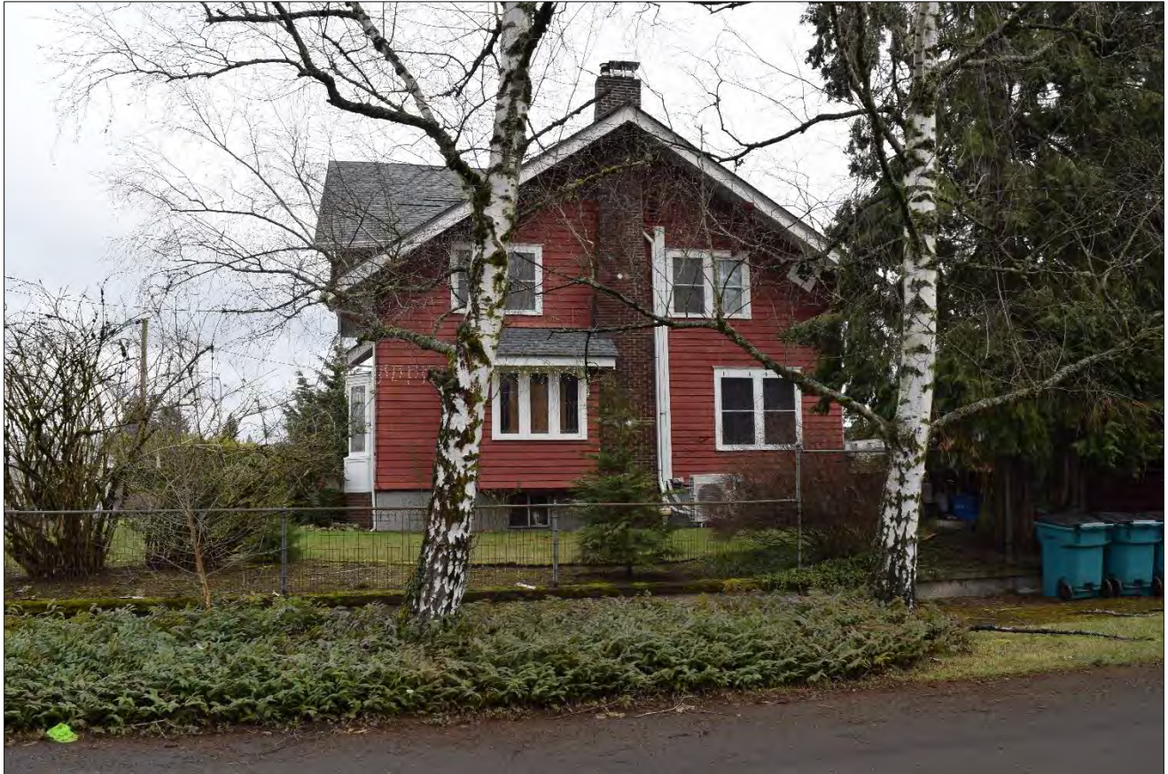
Figure 8. Hall House, west elevation, view facing east (WillametteCRA March 8, 2022).
