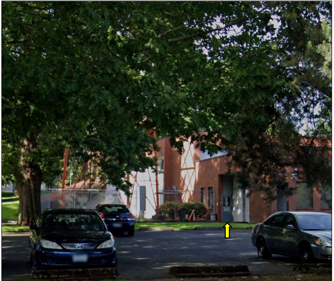
Figure 14. WSP District Five Headquarters, west and south elevation, view facing northeast. The arrow points to a half glass metal side entrance door (Google Street View, June 2019).
