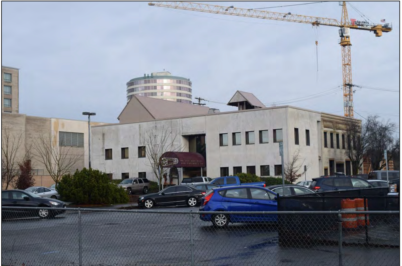
Figure 6. Webber Machine Works, west and south elevations, view facing northeast (WillametteCRA January 16, 2023).
