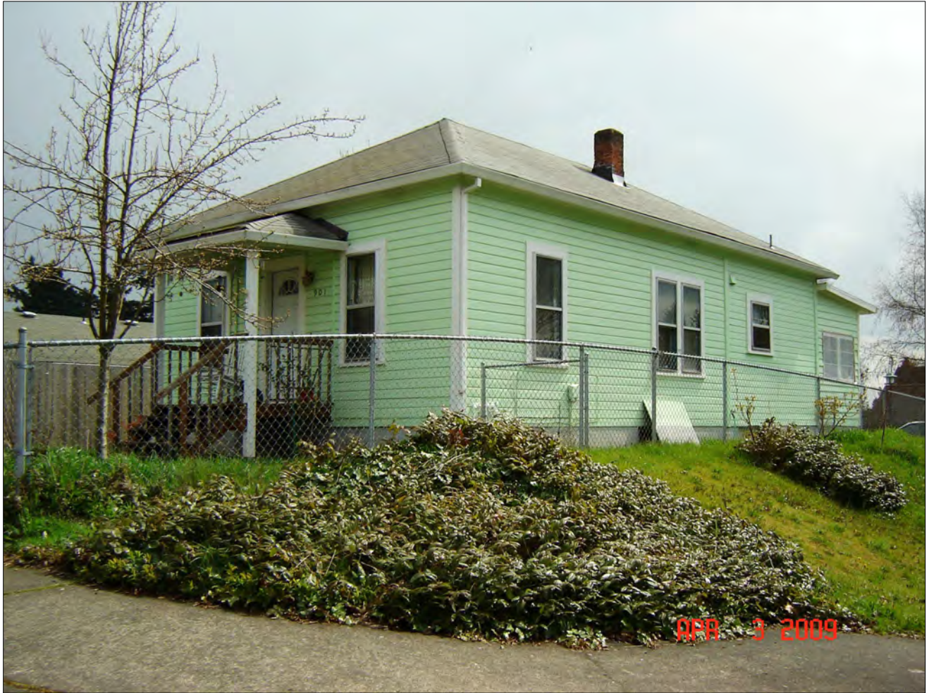
Figure 9. 901 East 29th Street, north and west elevations, view facing southeast (Clark County Assessor, 2009).
