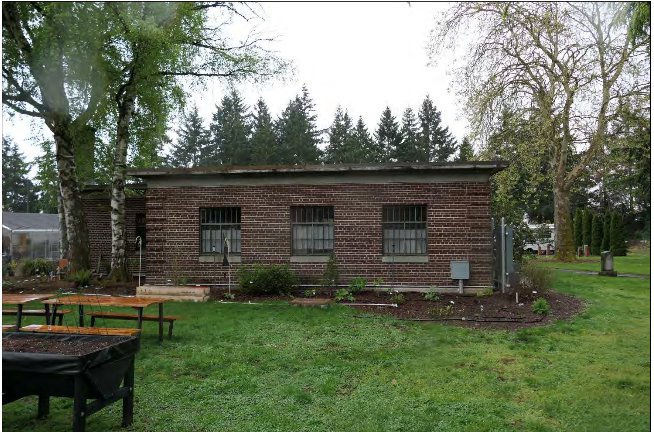
Figure 5. The Radio Transmission Building, north elevation, view facing south (WillametteCRA May 4, 2023).
