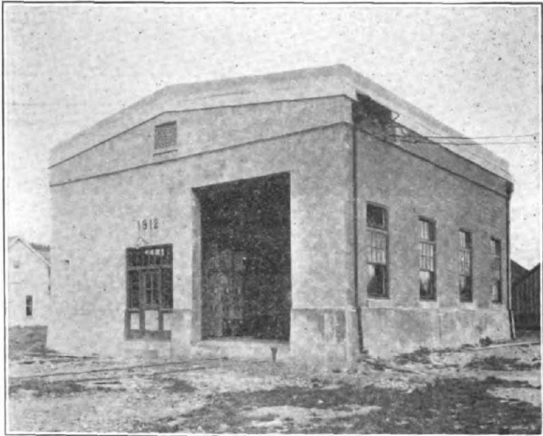
Exterior Dundee Substation.
