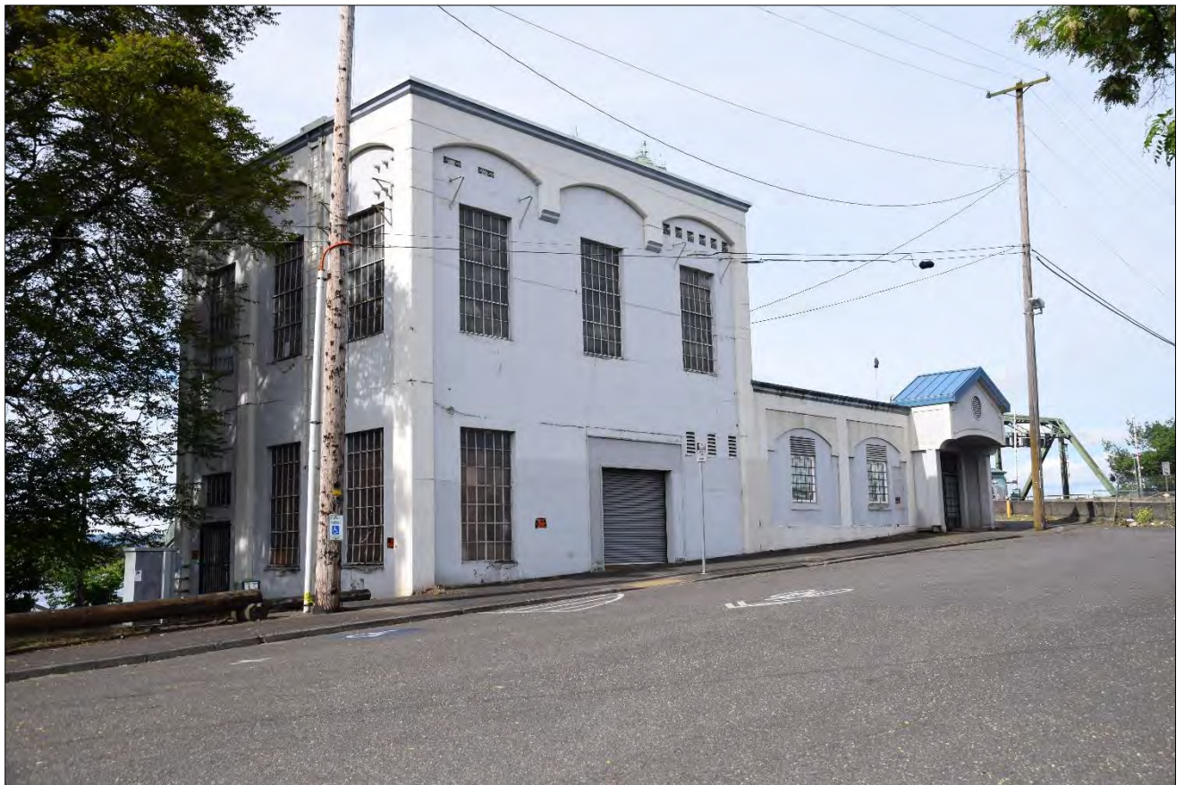
Figure 1. View of 100 SE Columbia Way from northeast (WillametteCRA June 8, 2022).
