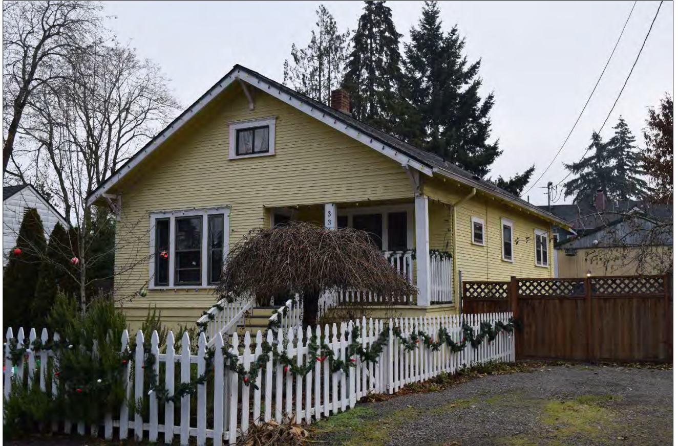
Figure 1. 3317 K Street Residence, west and south elevations, view facing northeast (WillametteCRA, December 14, 2022).
