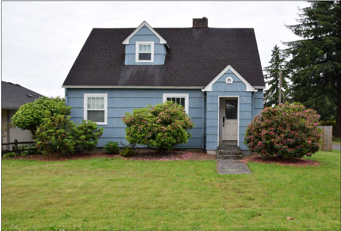
Figure 1. 901 East 32nd Street, north elevation, view facing south (WillametteCRA January 16, 2023).
