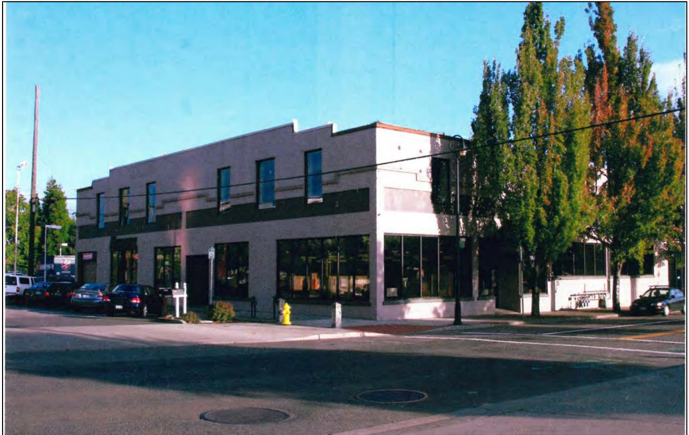
Figure 7. The Hankel Building, north and west elevations, view facing southeast, ca. 2008. Note the darker anodized aluminum windows on the first story and the enlarged second-story windows (Clark County Heritage Nomination Form for the Hankel Building, August 4, 2009).
