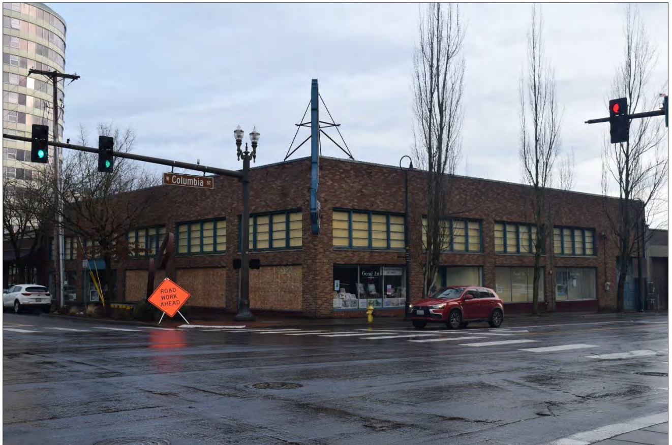
Figure 1. Fendrich's Furniture, north and west elevations, view facing southeast. Note vandalism of north-facing shopfront windows. (WillametteCRA January 13, 2023).
