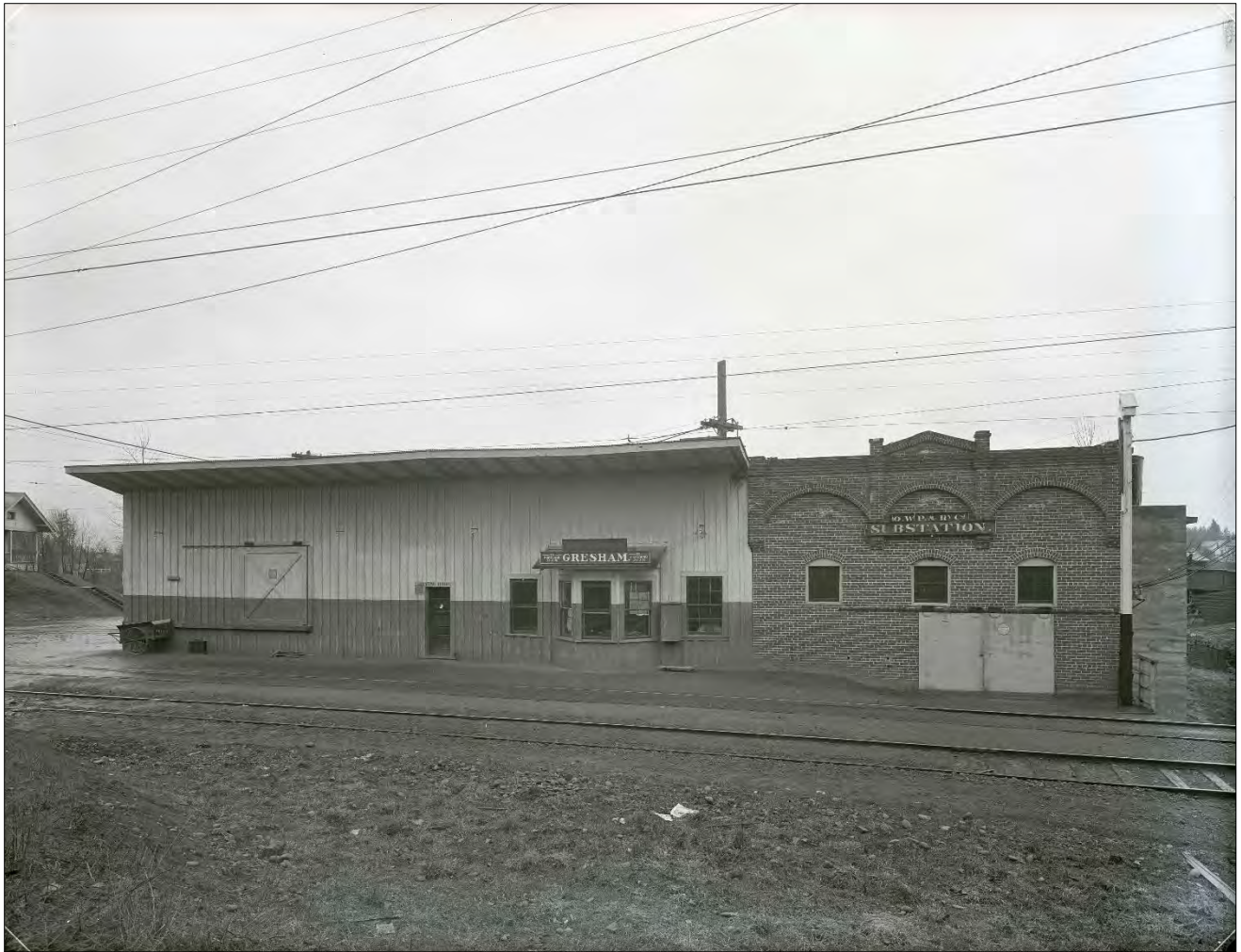
Figure 31. Portland Railway, Light and Power (PRLP) substation at Gresham, undated. Note the three segmental arches at the top of the substation, which recall the segmental arches on the exterior of the Bridge Substation (Oregon Historical Society).
