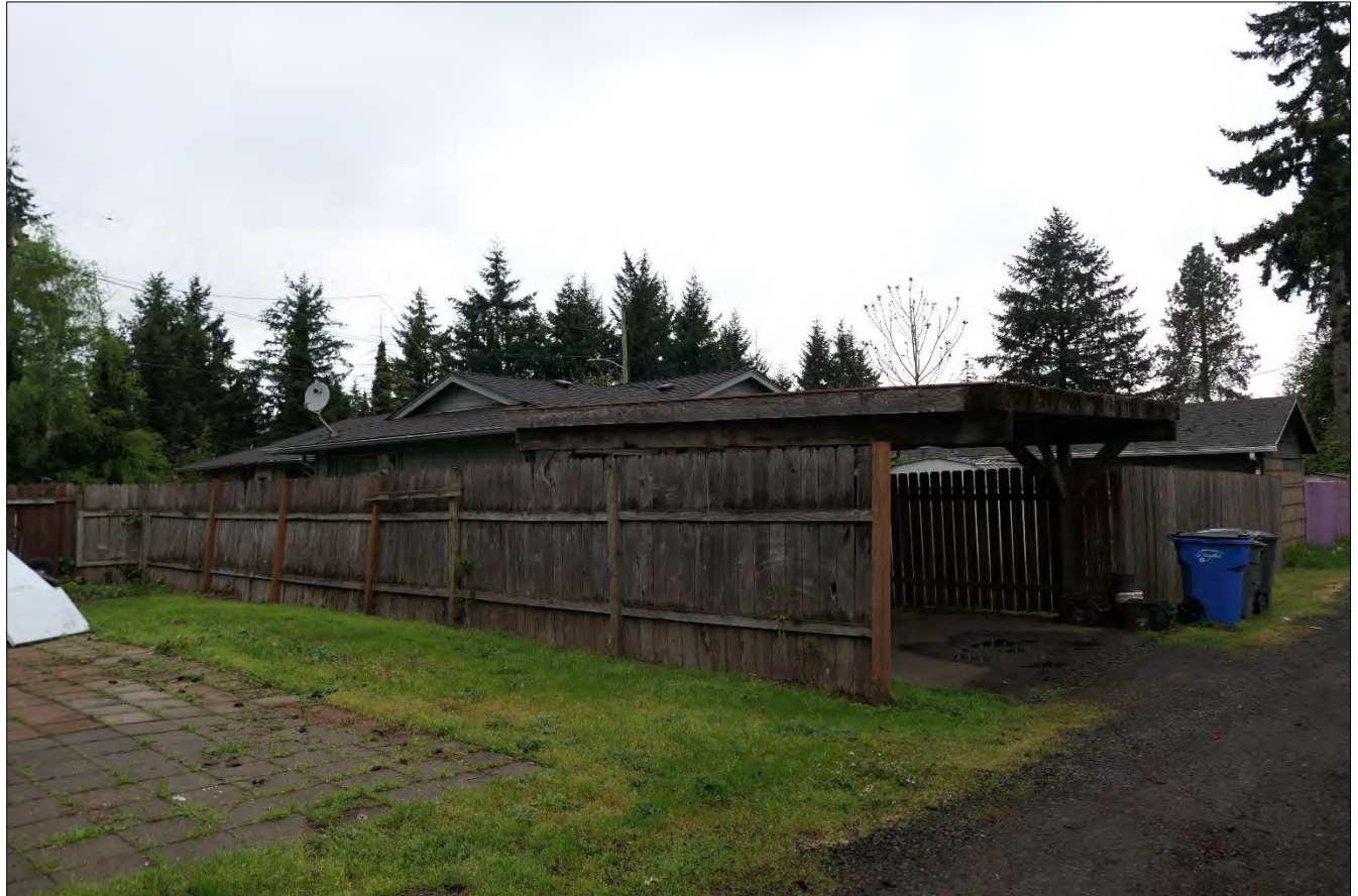
Figure 6. 3505 K Street, rear parking, view facing northwest (WillametteCRA May 4, 2023).
