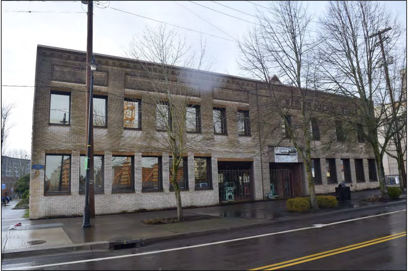
Figure 4. Webber Machine Works, east elevation, view facing northwest (WillametteCRA January 16, 2023).
