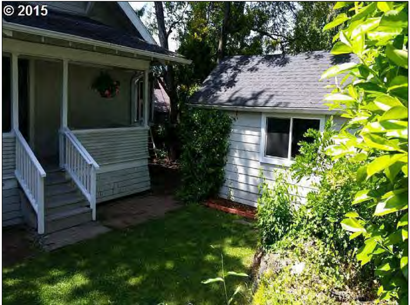
Figure 9. Hood Residence, east elevation, view facing northwest (Zillow, 2015).
