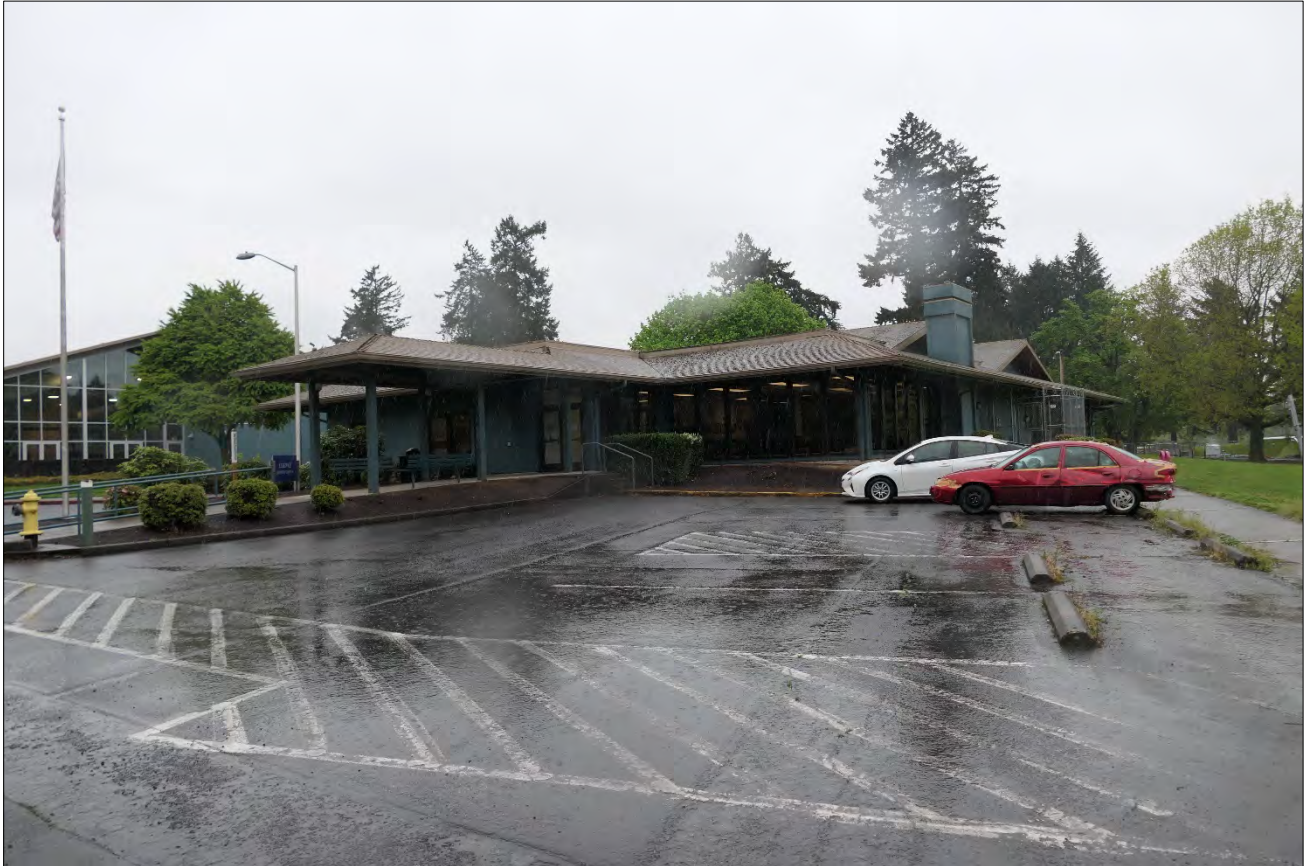
Figure 1. Luepke Center, southwest corner including main entrance, view facing northeast. (WillametteCRA, May 4, 2023).
