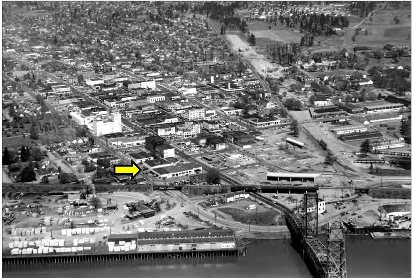
Figure 12. View facing northeast over downtown Vancouver, Washington, prior to the completion of the highway interchange, August 1953. Arrow points to the Hankel Building ( The Columbian via Pinterest).
