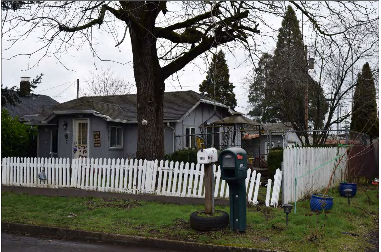
Figure 5. 3609 I Street, west and south elevations, view facing northeast (WillametteCRA March 8, 2023).
