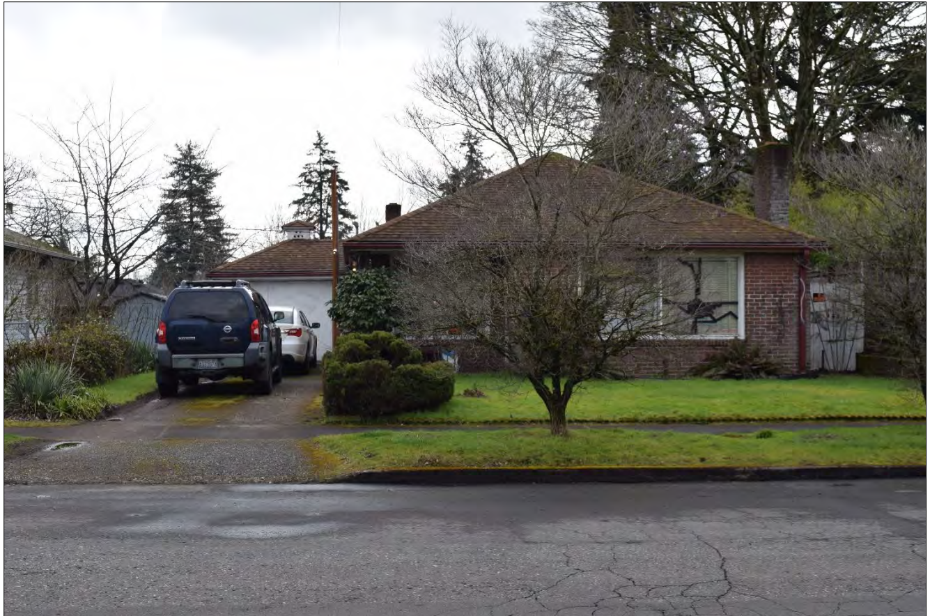
Figure 6. 809 East 29th Street, north elevation, view facing south (Willamette CRA March 8, 2023).
