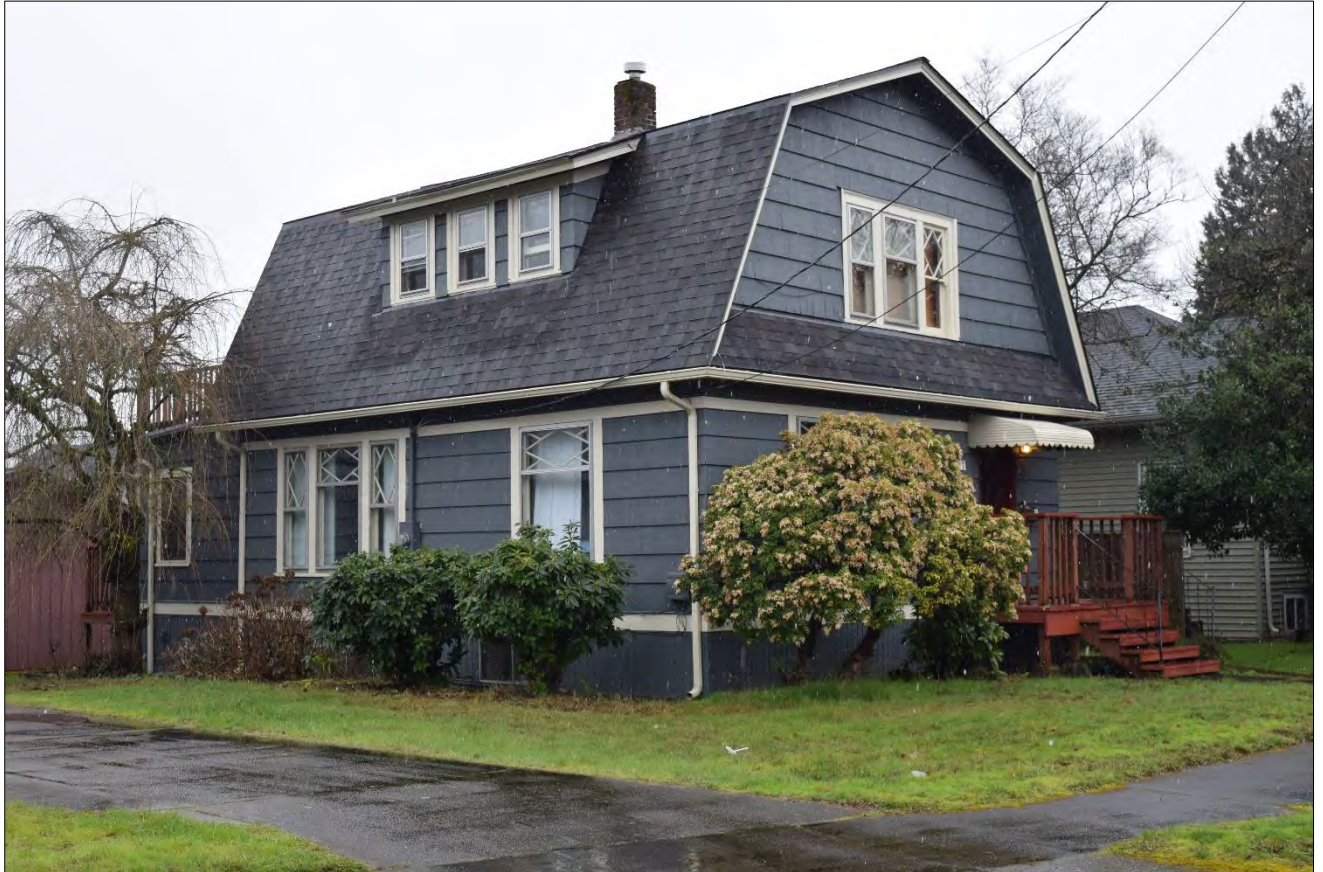
Figure 1. 3207 K Street, west and north elevation, view facing southeast (WillametteCRA March 8, 2023).
