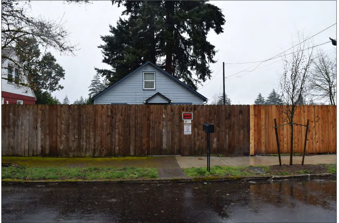
Figure 1. Maude Erhardt House, east elevation, view facing west. (WillametteCRA March 8, 2023).
