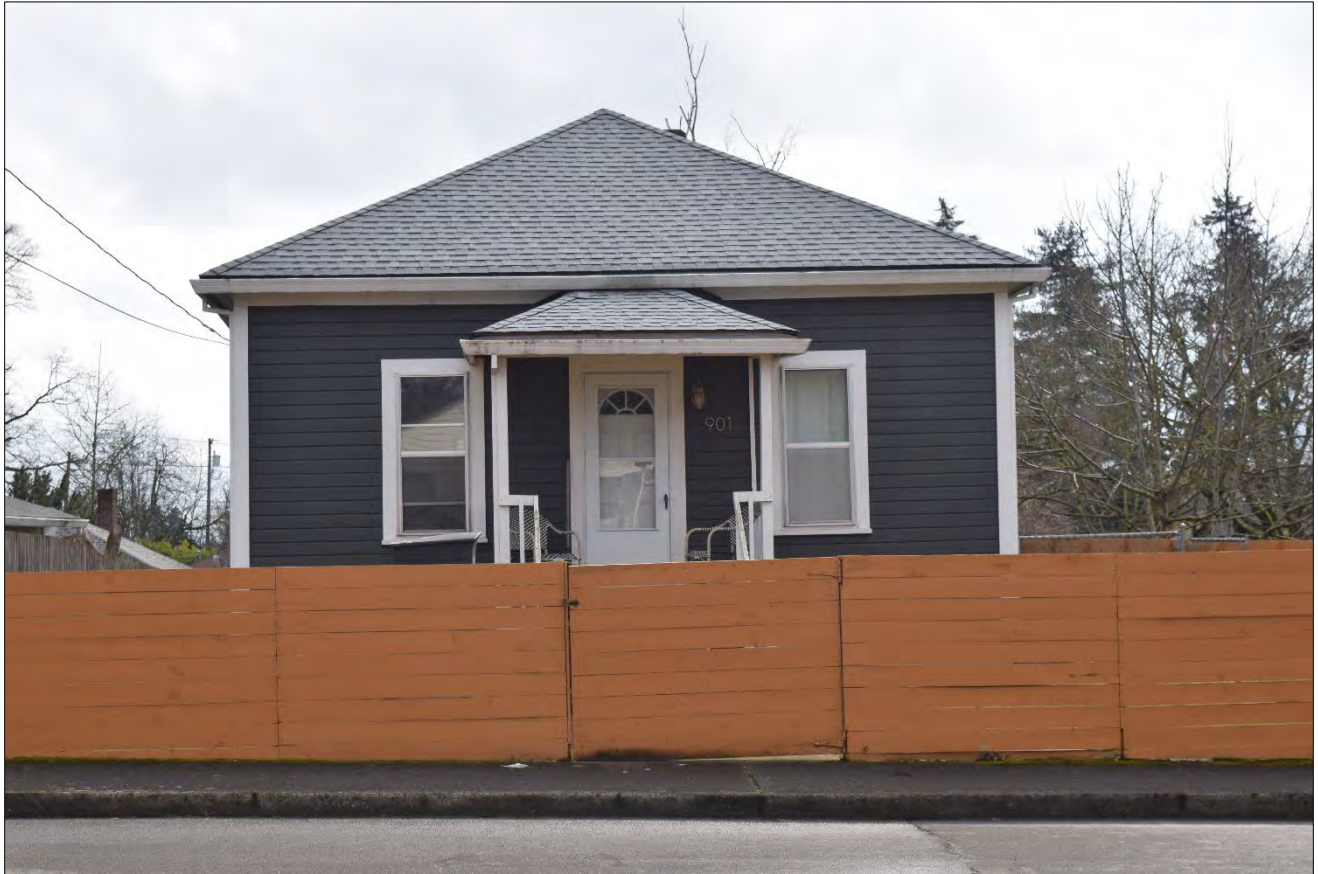
Figure 5. 901 East 29th Street, north elevation, view facing south (WillametteCRA March 8, 2023).
