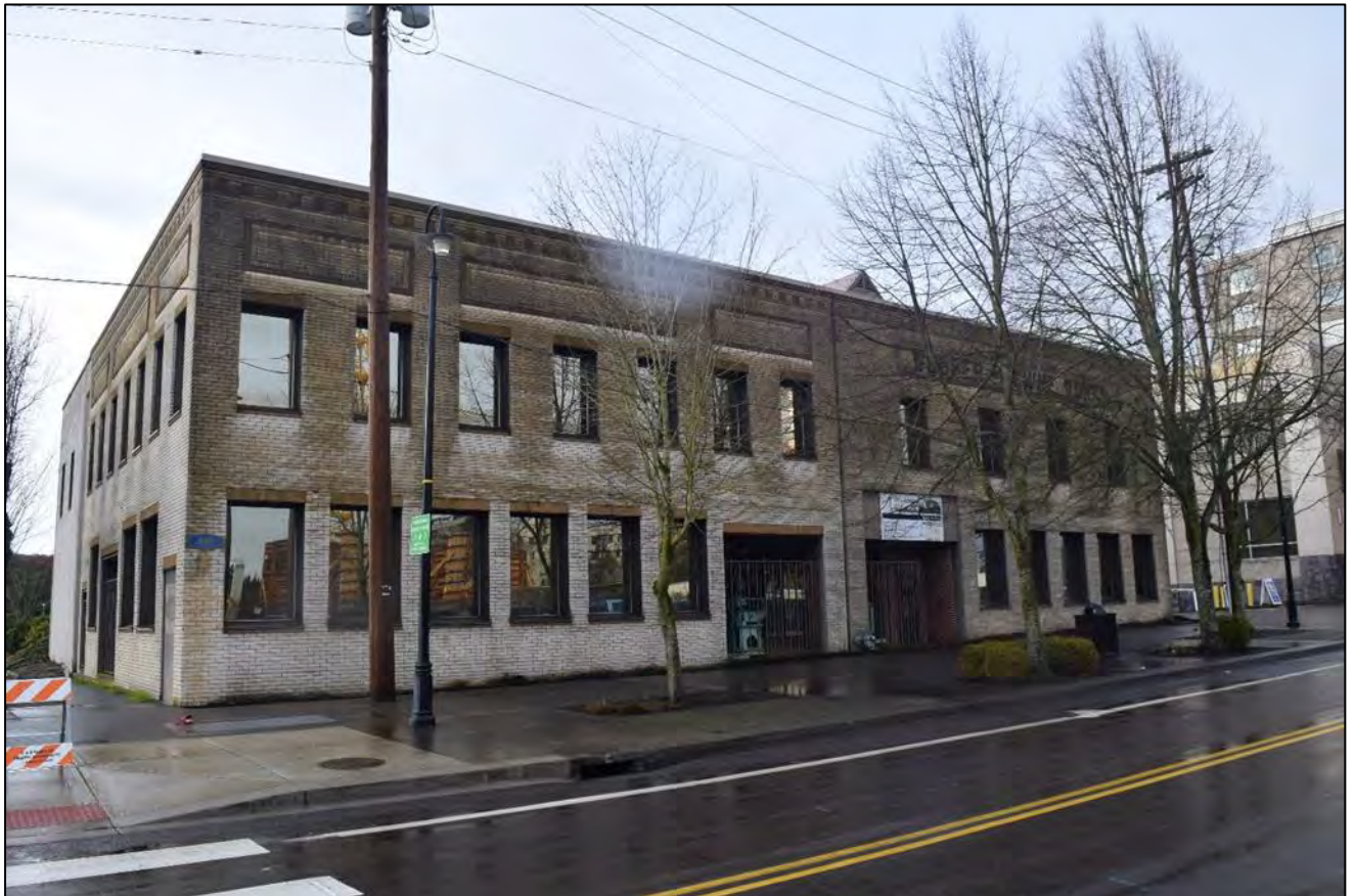
Figure 1. Webber Machine Works, south and east elevations, view facing northwest (WillametteCRA January 16, 2023).
