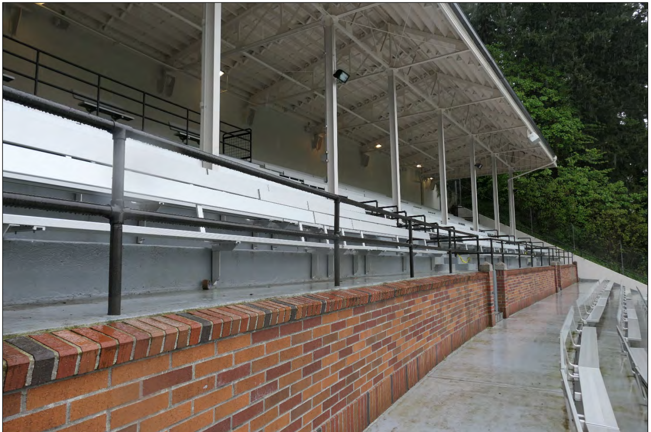
Figure 15. Kiggins Bowl stadium, detail of new brick retaining wall. View facing northwest (WillametteCRA May 6, 2023).
