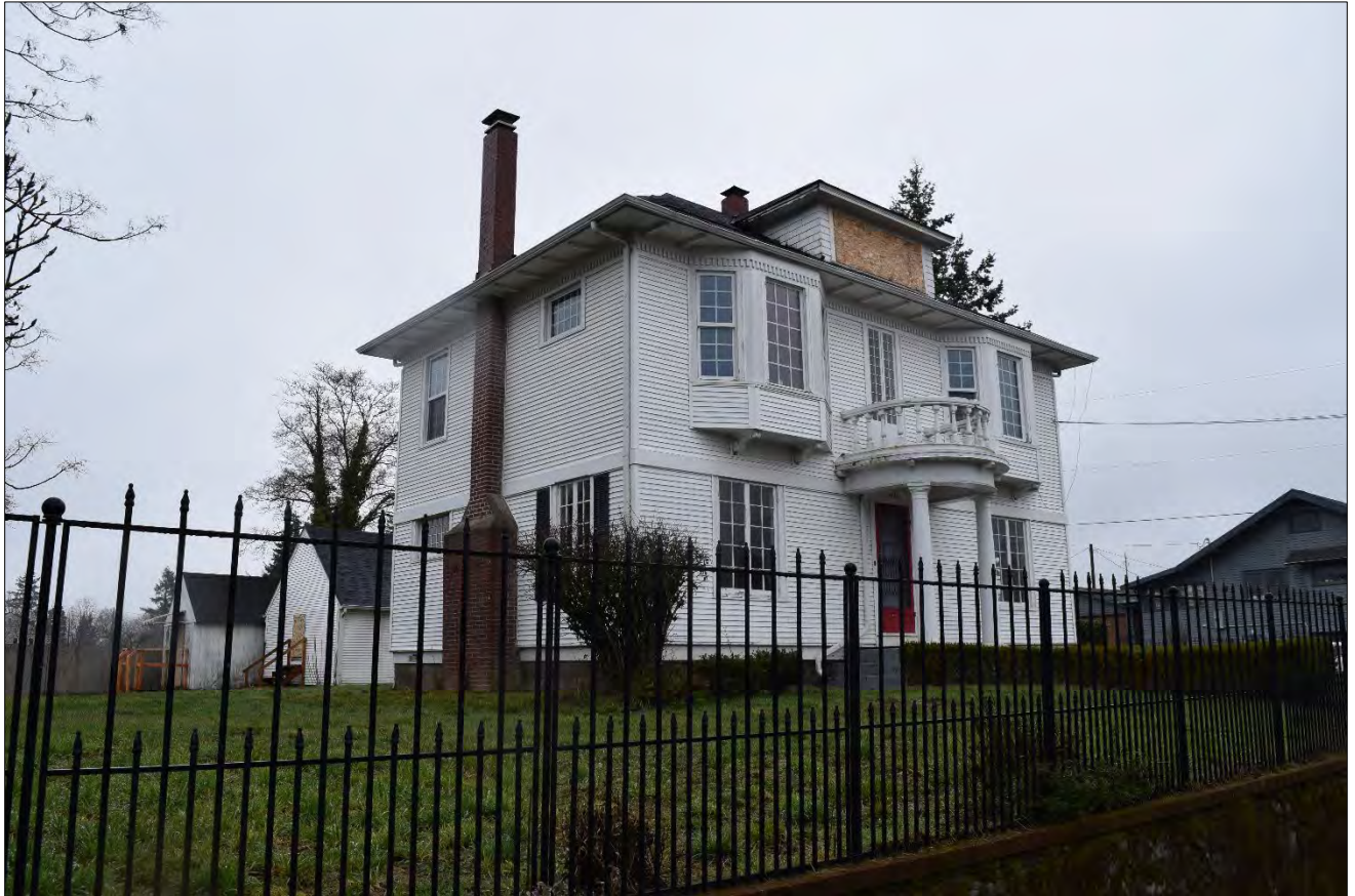
Figure 7. East and south elevations of 2914 K Street, view facing northwest. Note the garage and shed at the rear (WillametteCRA March 8, 2023).
