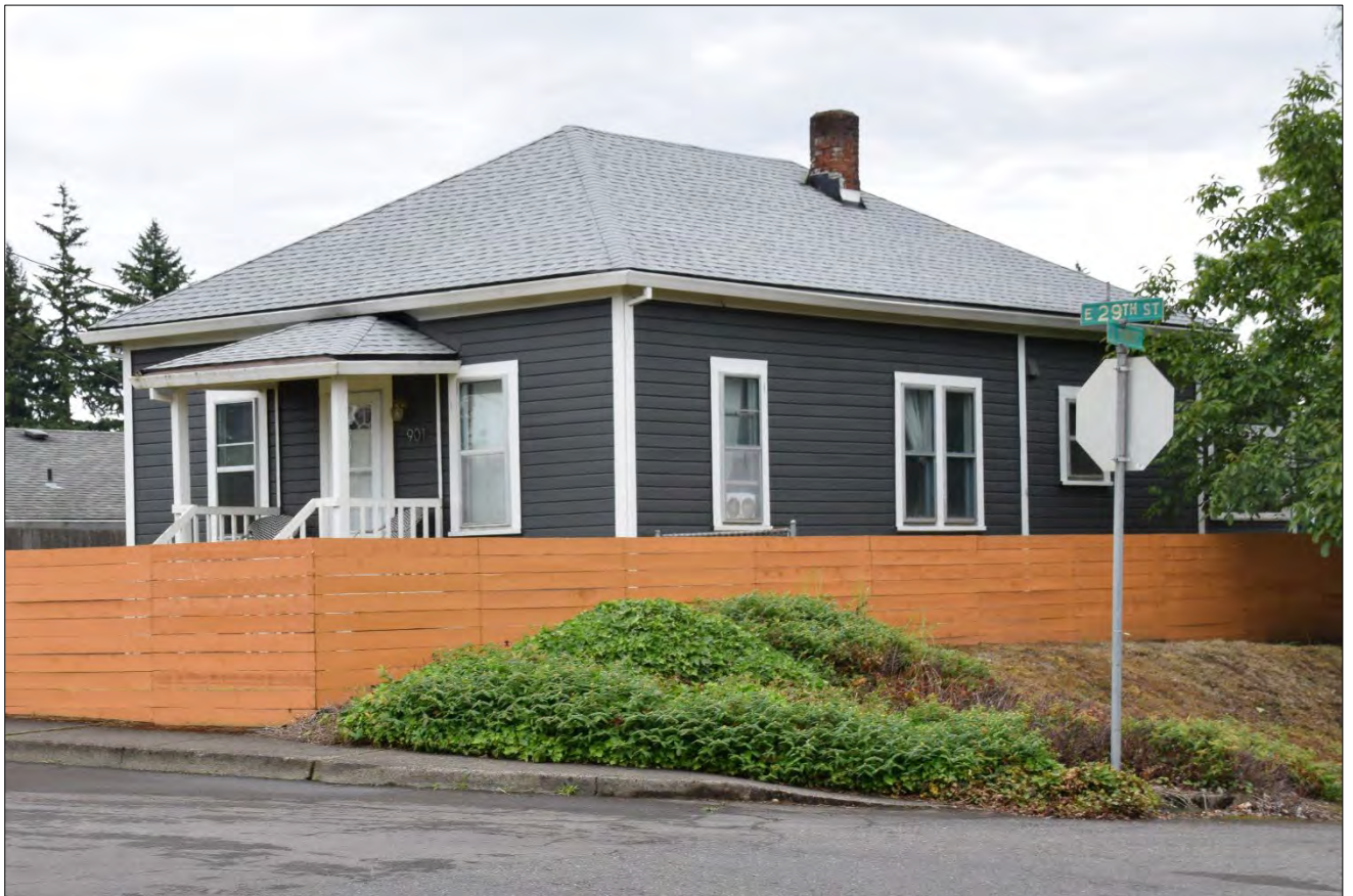
Figure 1. Mickler House, north and west elevations, view facing southeast (WillametteCRA June 9, 2022).
