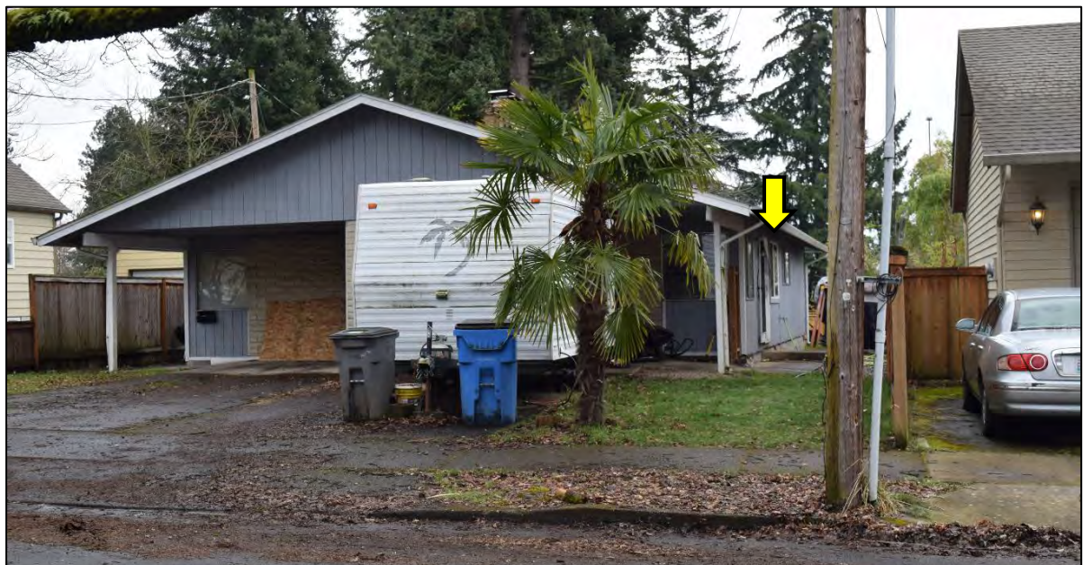
Figure 6. 607 East 27th Street Duplex Residences, north elevation (left) and west elevation (right), view facing southeast. Arrow points to vinyl window (WillametteCRA, March 8, 2023).
