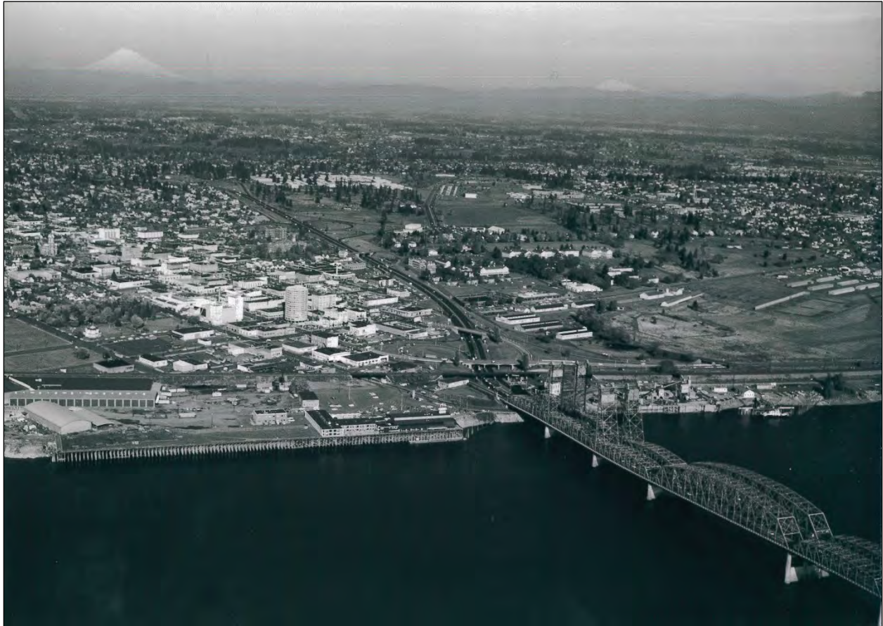
Figure 20. Aerial photograph of Vancouver, oblique view looking northeast, ca. 1965. The Smith Tower in downtown Vancouver is visible in the left side of the photograph and Vancouver Barracks is visible in the right side (Washington State Archives AR115-B-2_ph004881).
