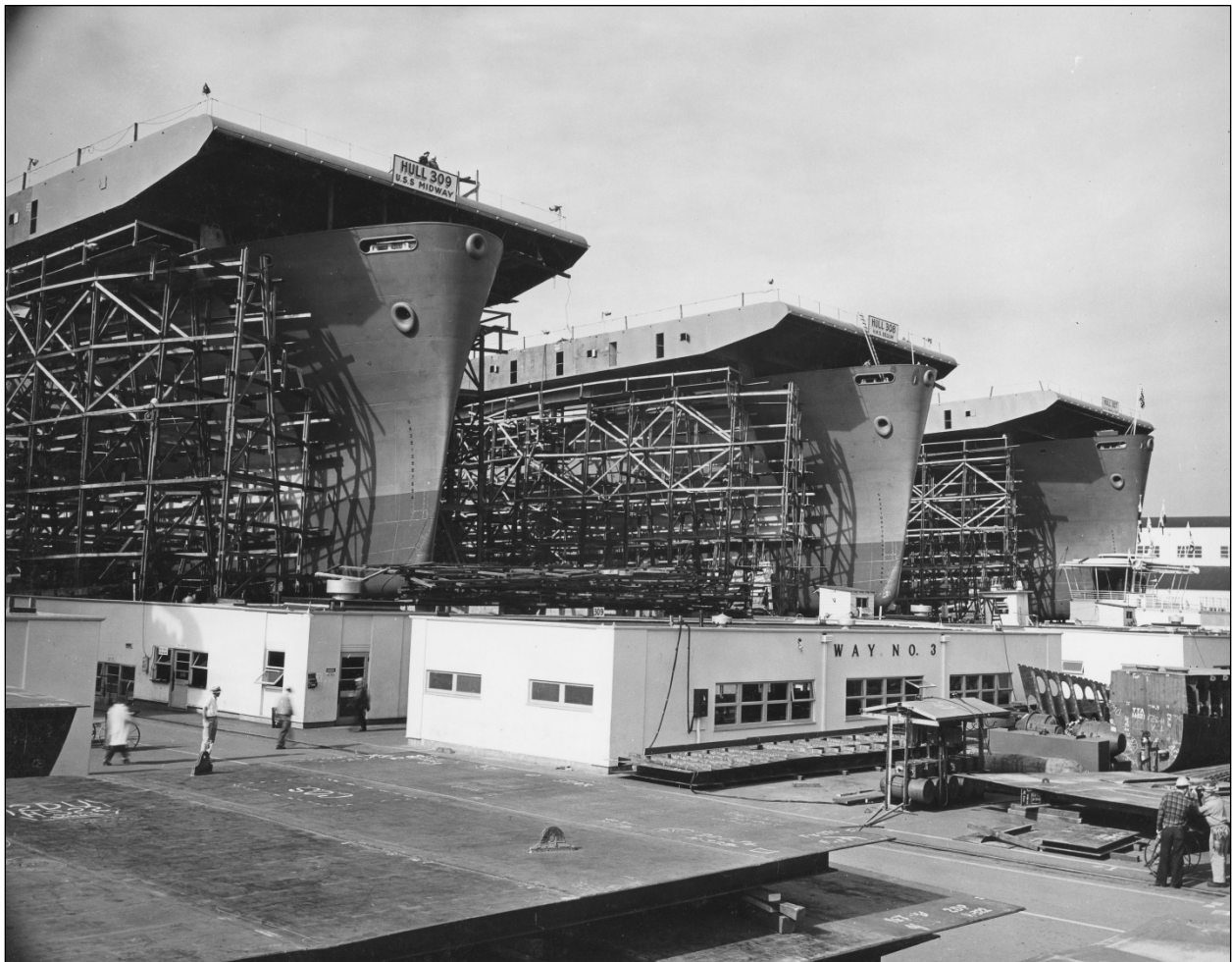
Figure 18. Aircraft carriers under construction at Vancouver's Kaiser shipyard. Louis Lee. Ships at dry dock . Ca. 1940s. Asset ID: B5D779CF-1DD8-B71B-0B02ACDDFFA9720D (NPS).
