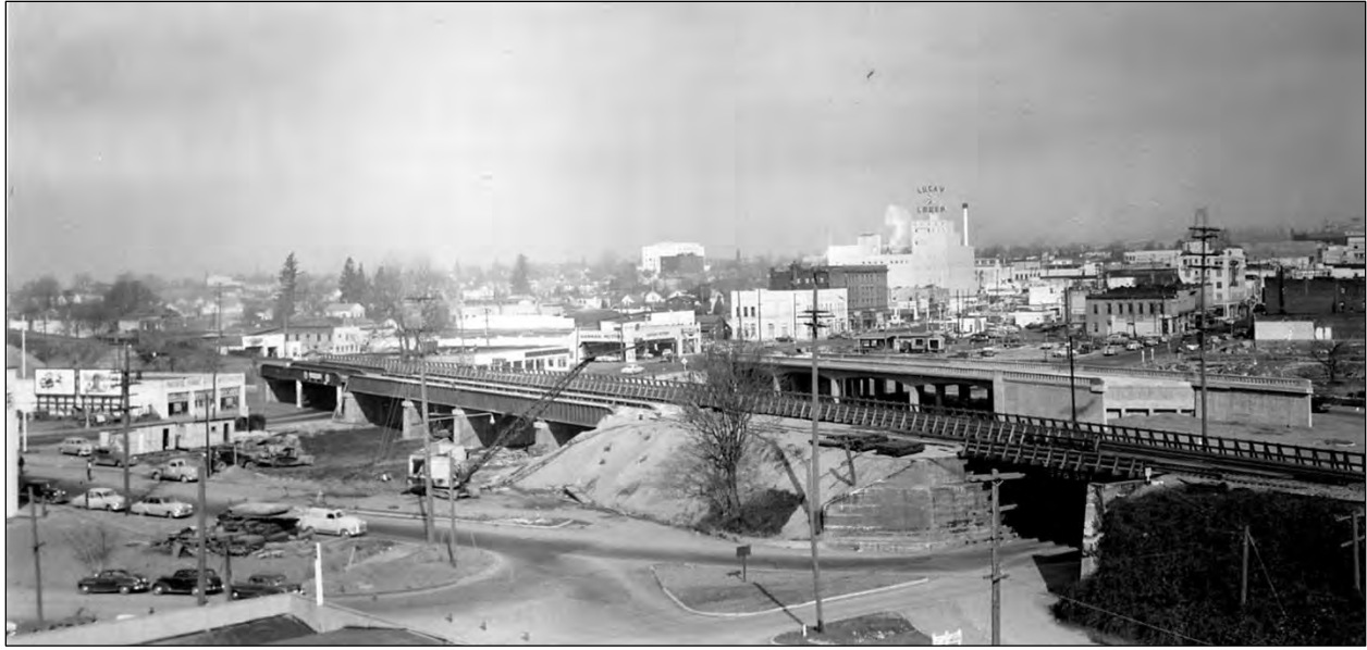
Figure 31. Initial construction of the Vancouver Freeway, view looking northwest, ca. November 1951 to June 1953. (Washington Department of Transportation).
