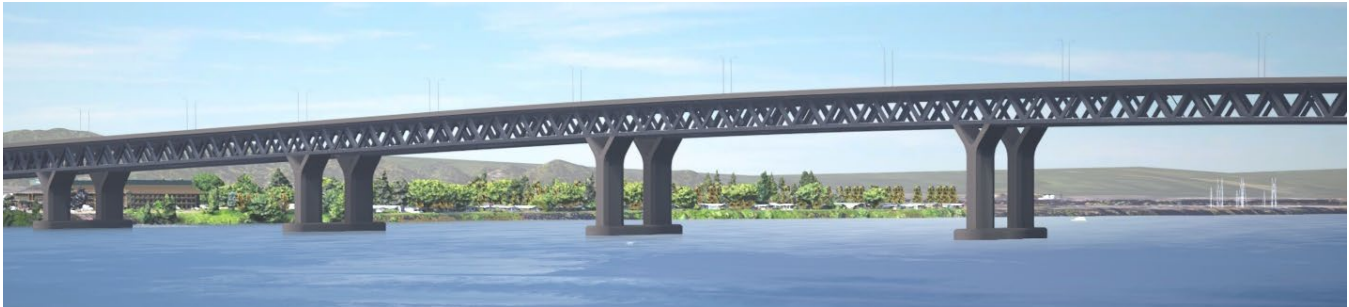
Figure 1-15. Conceptual Drawing of a Double-Deck Fixed-Span Configuration
