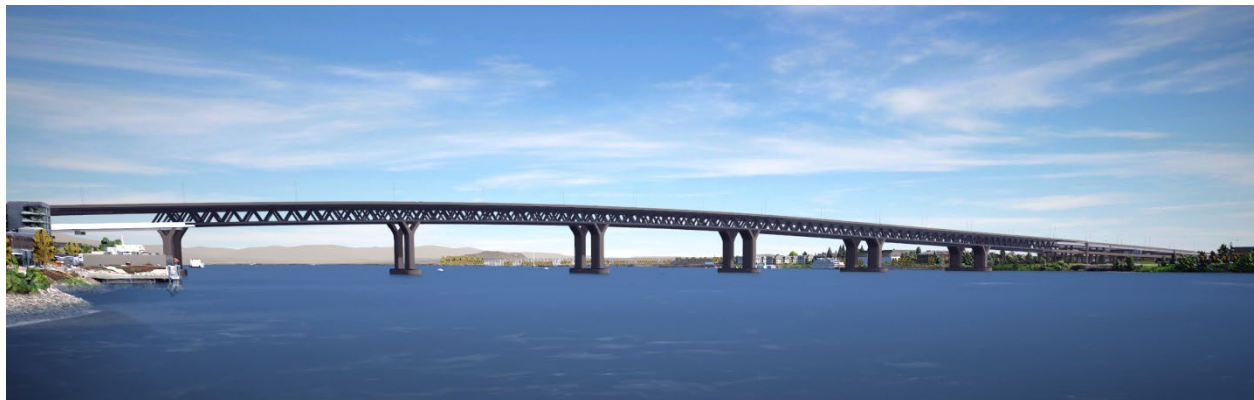
Figure 3. Conceptual Drawing of the Double-Deck Fixed-Span Bridge Configuration
