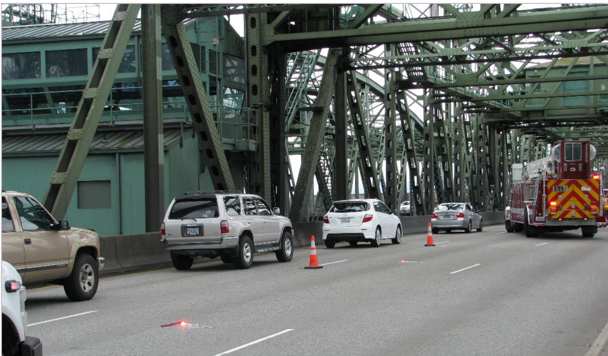
Figure 1-2. Crash Blocking the Interstate Bridge
