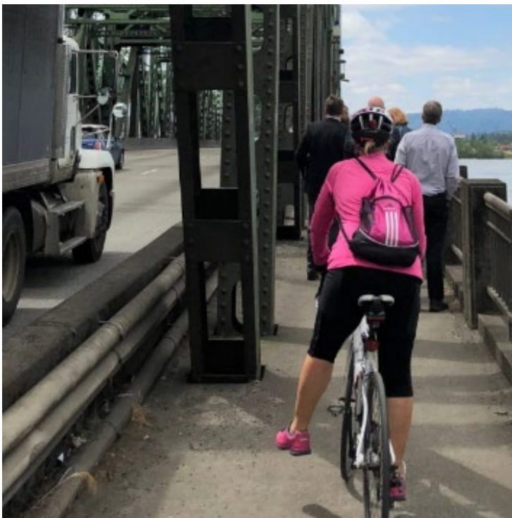
Figure 3. Bicycle and Pedestrian Path on the Interstate Bridge
