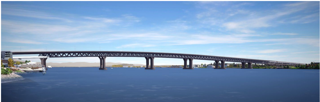
Figure 1-14. Conceptual Drawing of a Double-Deck Fixed-Span Configuration
