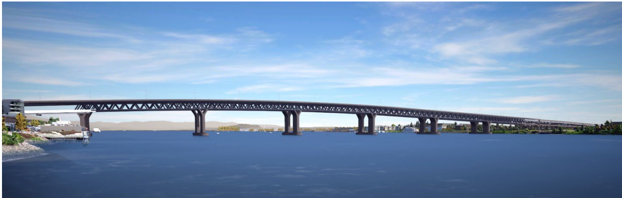
Figure 1-14. Conceptual Drawing of a Double-Deck Fixed-Span Configuration
