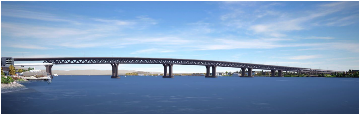
Figure 1-14. Conceptual Drawing of a Double-Deck Fixed-Span Configuration
