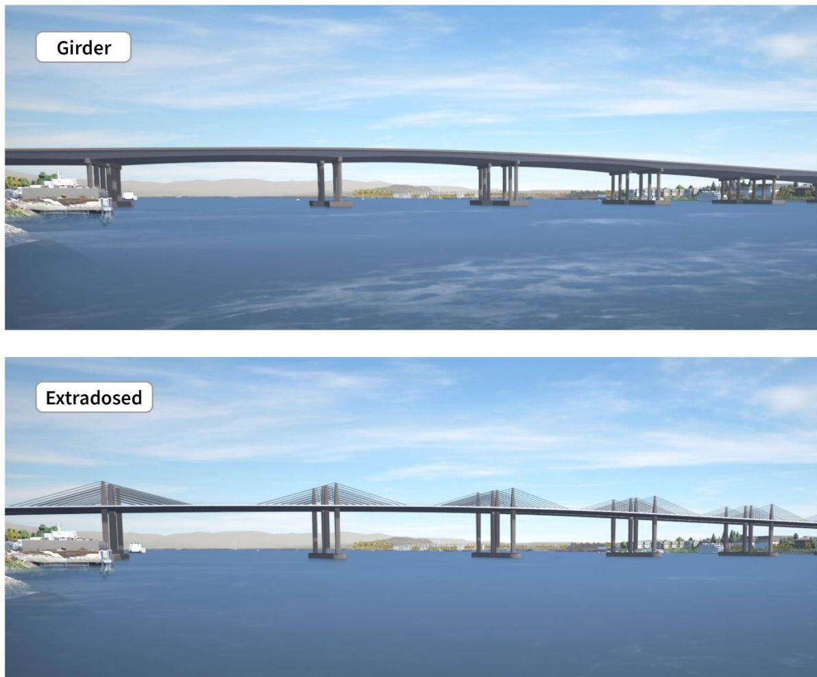
Figure 1-16. Conceptual Drawings of Single-Level Fixed-Span Bridge Types
