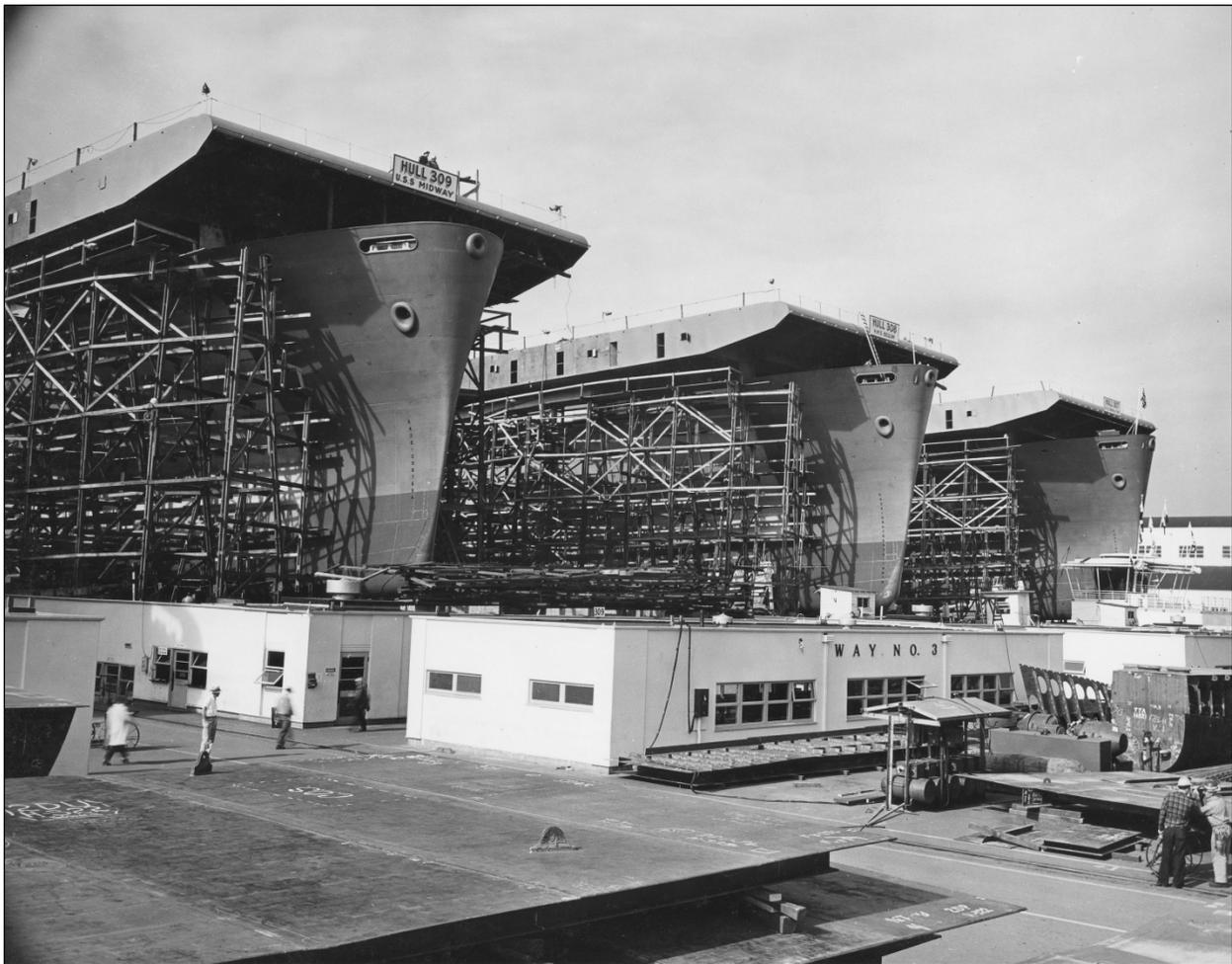
10 Figure 18. Aircraft carriers under construction at Vancouver's Kaiser shipyard. Louis Lee. *Ships at dry dock*. Ca. 1940s. Asset ID: B5D779CF-1DD8-B71B-0B02ACDDFFA9720D (NPS).
