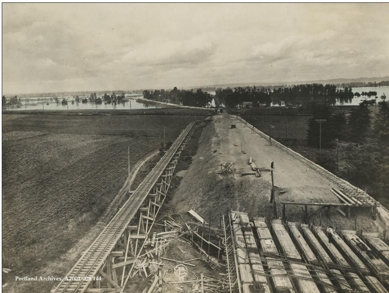
Figure 19. Union Avenue (present-day NE Martin Luther King Boulevard) under construction in 1916. View looking north-northwest. The partially constructed viaduct over the Oregon and Washington Navigation Company tracks is in the foreground while the line's shoefly is seen on the left (City of Portland Archives, A2001-008.144).
