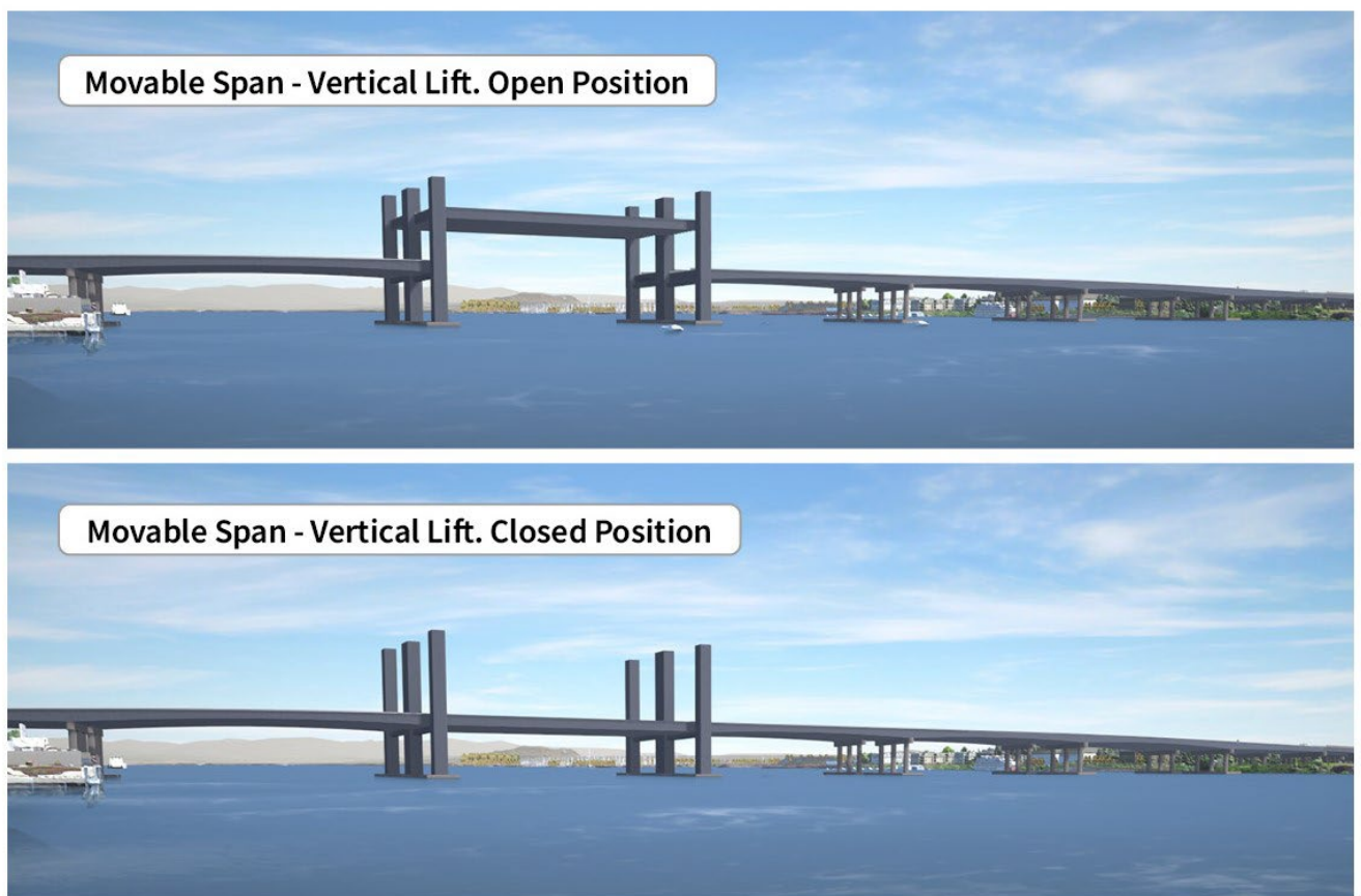
Figure 1-23. Conceptual Drawings of Single-Level Movable-Span Configurations in the Closed and Open Positions
