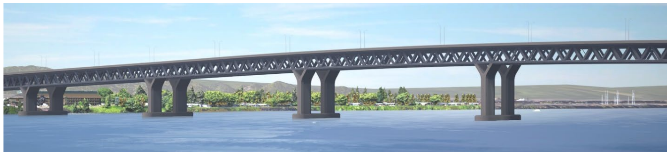
Figure 1-15. Conceptual Drawing of a Double-Deck Fixed-Span Configuration
