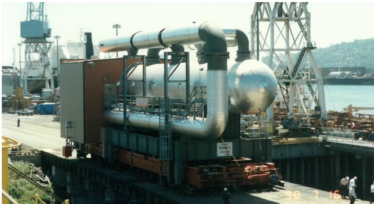
This massive process module is being loaded out for delivery to the North Slope of Alaska in July 1990. This industrial equipment rivals the size of most downtown buildings and is representative of the equipment currently being requested for North Slope expansion projects. Due to scale and complex nature of work, this sort of equipment cannot be manufactured at the remote jobsite or accomplished at all in Alaska.
