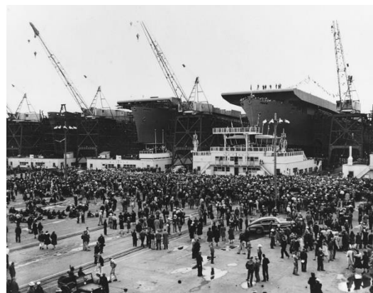
[1943] Escort carriers at the Vancouver Shipyards (current day Thompson Metal Fab)
