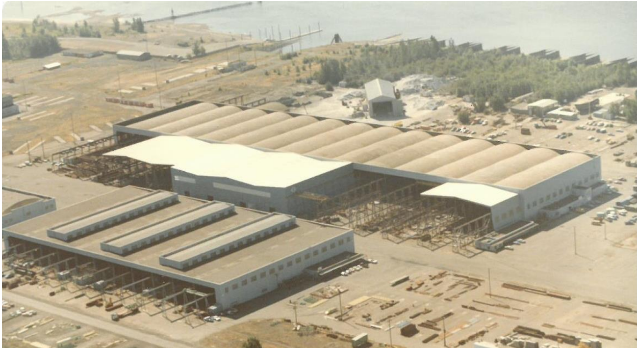
Taken in the early 1970's, the photo above shows Thompson Metal Fab shortly after closing the original facility in Portland and moving to Vancouver. Thompson added fiberglass roofing and walls to bays 5 through 9 to create an enclosed space. The land has been developed quite a bit in the last 40-years (including improvements to the roll-on/roll-off barge slip), but the building remains virtually the same.
