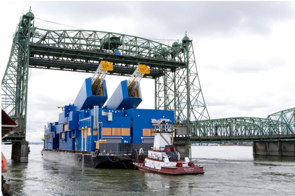
Picture of the Interstate Bridge in 2011 showing both the original Northbound span (background) and the second span (foreground) which opened in 1958 to traffic in both directions. In 1960, the second span was dedicated to Southbound traffic only. (Photo shows TMF manufactured drill rigs, AADU Rig 272 & 273 for Parker Drilling)
