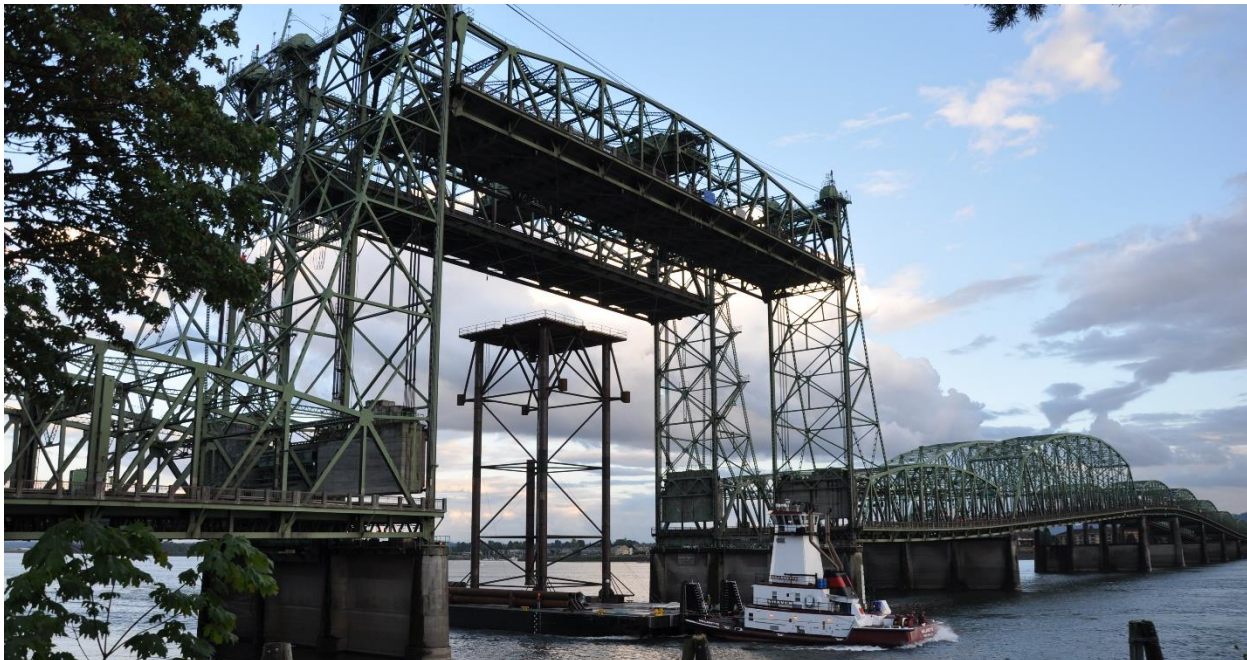
With a structural height of 126', this pile template for a monopod in the Cook Inlet (Alaska) is one of the largest structures to ship from the Columbia Business Center in the last 40-years. Thompson Metal Fab manufactured piling for this project, delivered in 2014.
