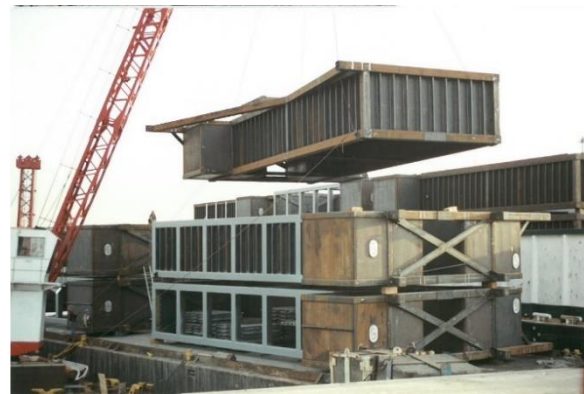
Shown above and below are multiple barge loadings for a massive project at Lower Granite Dam in the mid-1990’s. All structures were fabricated by Thompson Metal Fab and loaded out at the Columbia Business Center.
