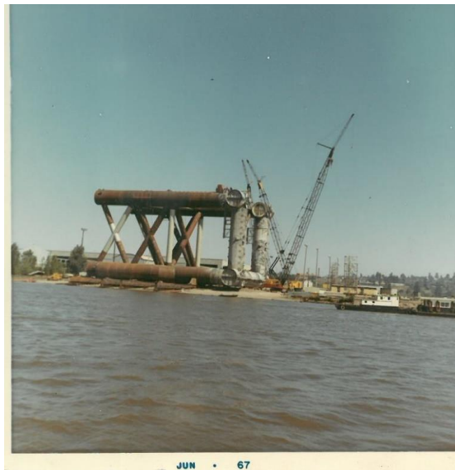
Infrastructure for the California offshore oil fields being manufactured at the Columbia Business Center in 1967. Thompson Metal Fab would begin operations here a few years later in 1973.
