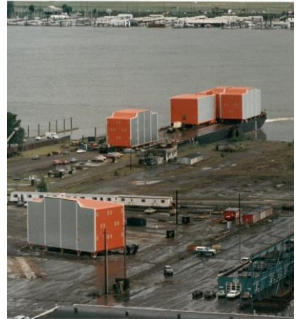
Load out of housing modules manufactured by Thompson Metal Fab. This housing will be used for the workers on Alaska’s North Slope.
