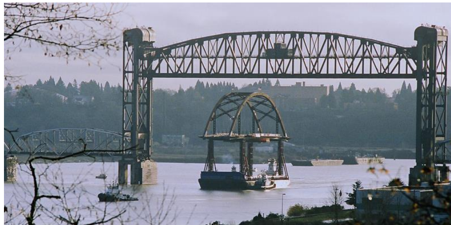
Image above shows the Sauvie Island Bridge being shipped to the jobsite via barge on the Willamette River and passing under the Burlington Northern RR Bridge in Portland, OR. Delivery of steel for the new Burnside Bridge would take a similar approach, due to the limited area for construction at the jobsite in downtown Portland, OR. Bridge steel coming from the Columbia Business Center would pass under the Interstate Bridge to reach the jobsite.
