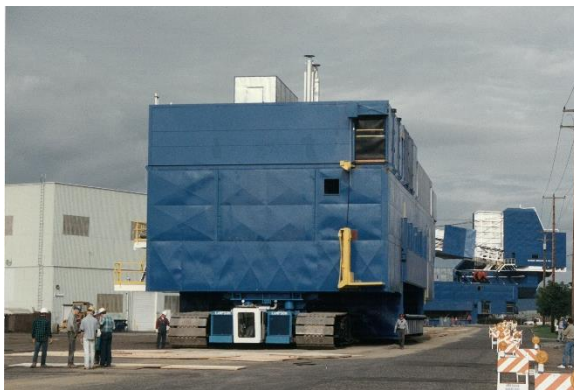
A large module for Parker Drilling Rig 245 moving from TMF's shop to their yard for assembly. Seen in the background is the mast and substructure of this massive drilling rig.
