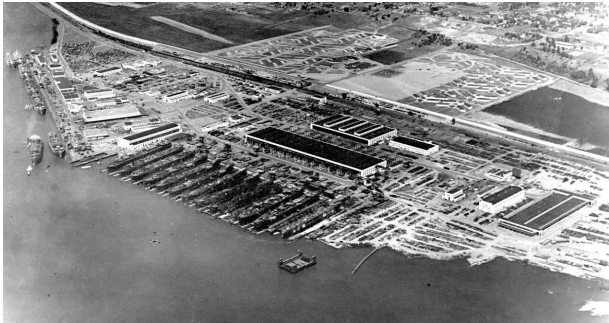
Building 40 and 41 of current day Thompson Metal Fab is shown prominently in the middle of this picture. At the time this picture was taken (circa early 1940's) the building and entire industrial area would have been known as Kaiser's Vancouver Shipyards.
