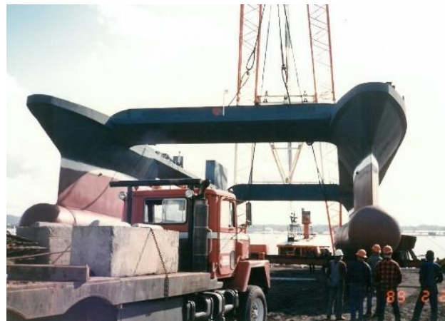
These structures are 9' diameter x 132' long and part of a Small Waterplane Area Twin Hull (SWATH). Once assembled in Thompson's yard, the hull measured 53' wide and nearly 60' high once outfitted with the superstructure. Thompson's location adjacent to the Columbia River was a key part in earning this business. After testing in the river, the "Navatek" shipped to Hawaii where the vessel still operates.
