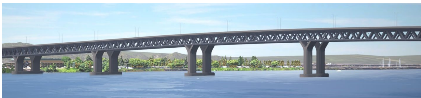
Figure 1-15. Conceptual Drawing of a Double-Deck Fixed-Span Configuration
