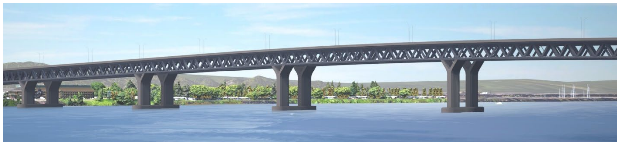
Figure 1-15. Conceptual Drawing of a Double-Deck Fixed-Span Configuration
