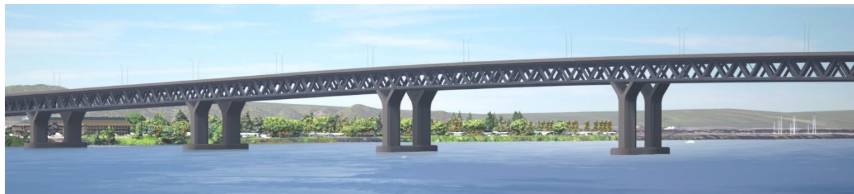
Figure 1-15. Conceptual Drawing of a Double-Deck Fixed-Span Configuration
