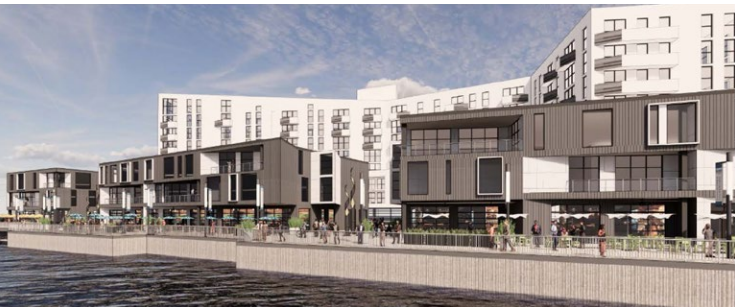
3 Proposed development at Renaissance Boardwalk
