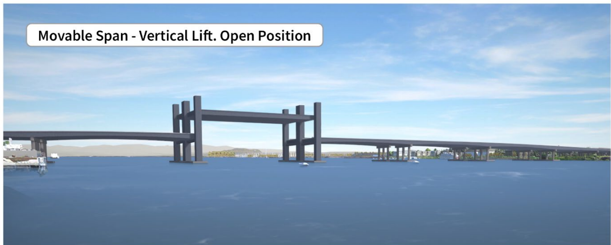
Figure 1-23. Conceptual Drawings of Single-Level Movable-Span Configurations in the Closed and Open Positions
