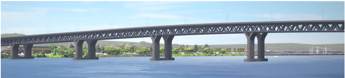
Figure 1-15. Conceptual Drawing of a Double-Deck Fixed-Span Configuration
