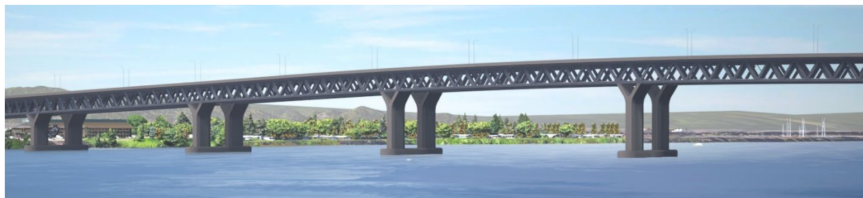
Figure 1-15. Conceptual Drawing of a Double-Deck Fixed-Span Configuration
