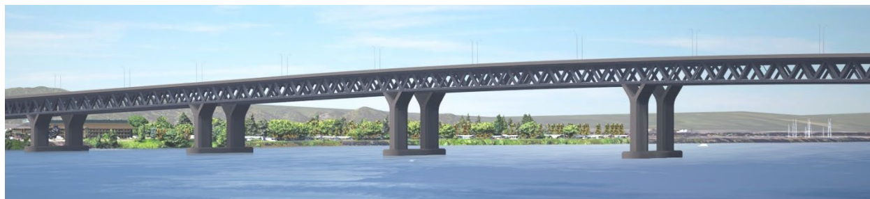
Figure 1-15. Conceptual Drawing of a Double-Deck Fixed-Span Configuration
