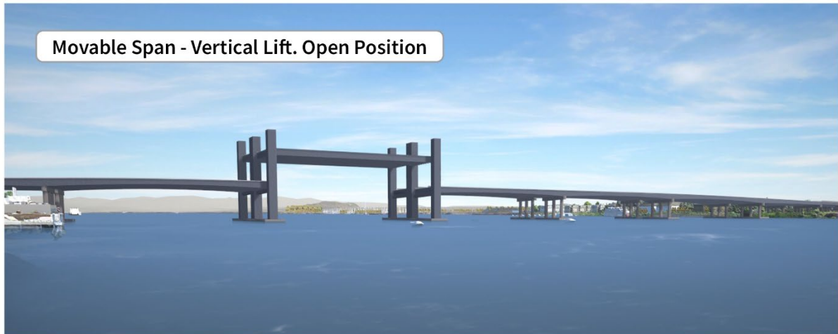
Figure 1-19. Conceptual Drawings of Single-Level Movable-Span Configurations in the Closed and Open Positions
