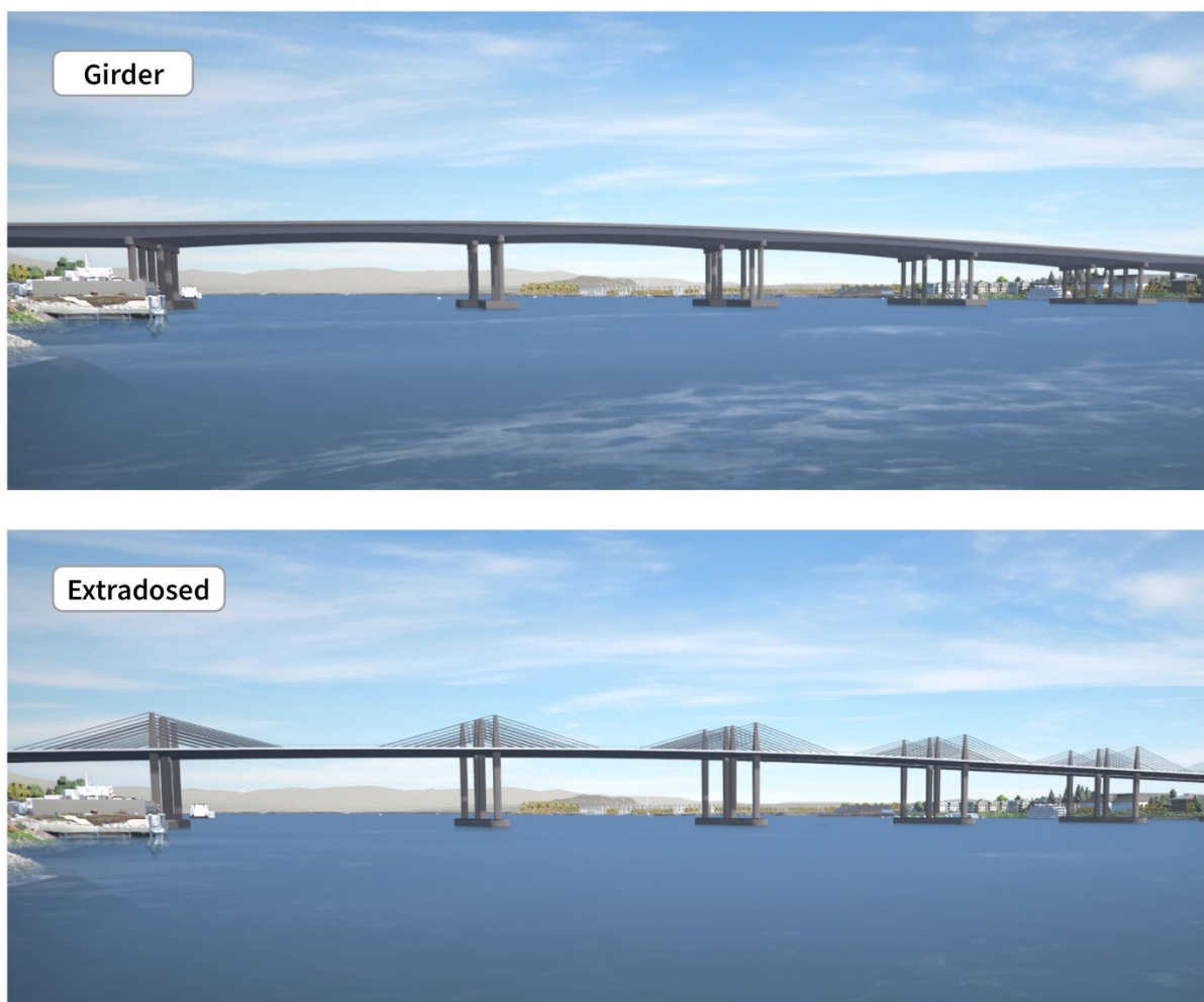
Figure 1-16. Conceptual Drawings of Single-Level Fixed-Span Bridge Types
