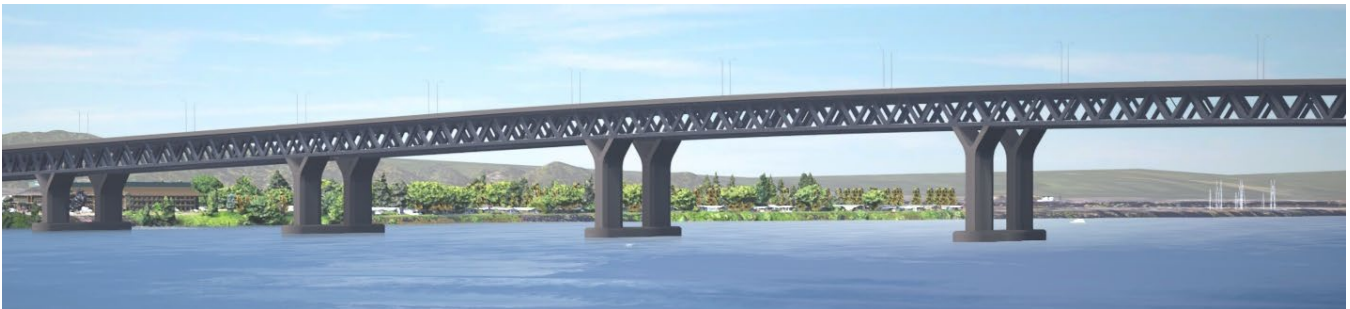
Figure 2-15. Conceptual Drawing of a Double-Deck Fixed-Span Configuration
