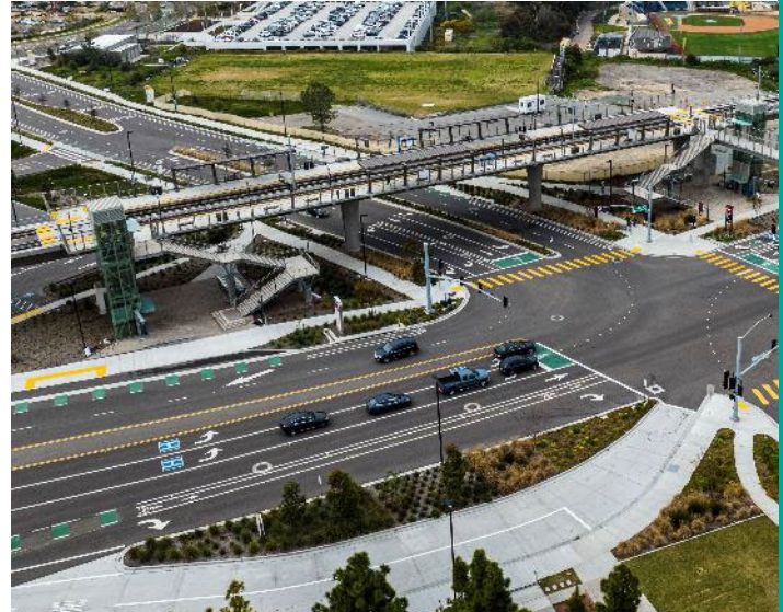
Elevated station example (UCSD)
