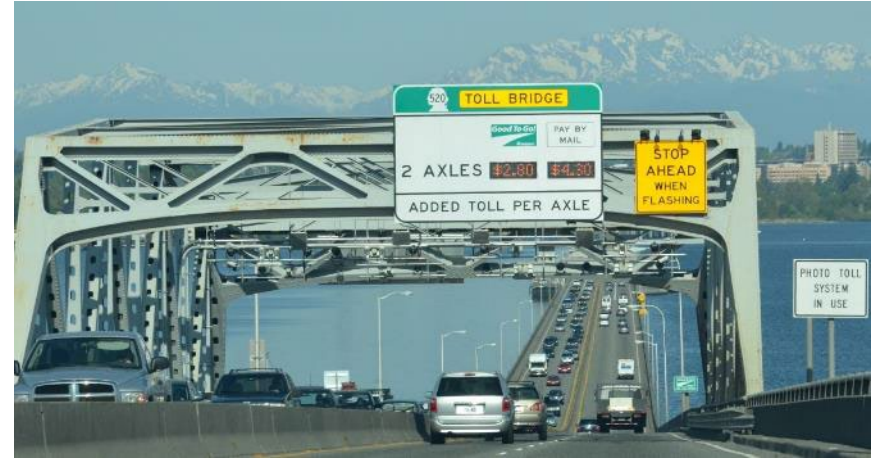
Electronic toll gantries on SR520 in Washington
